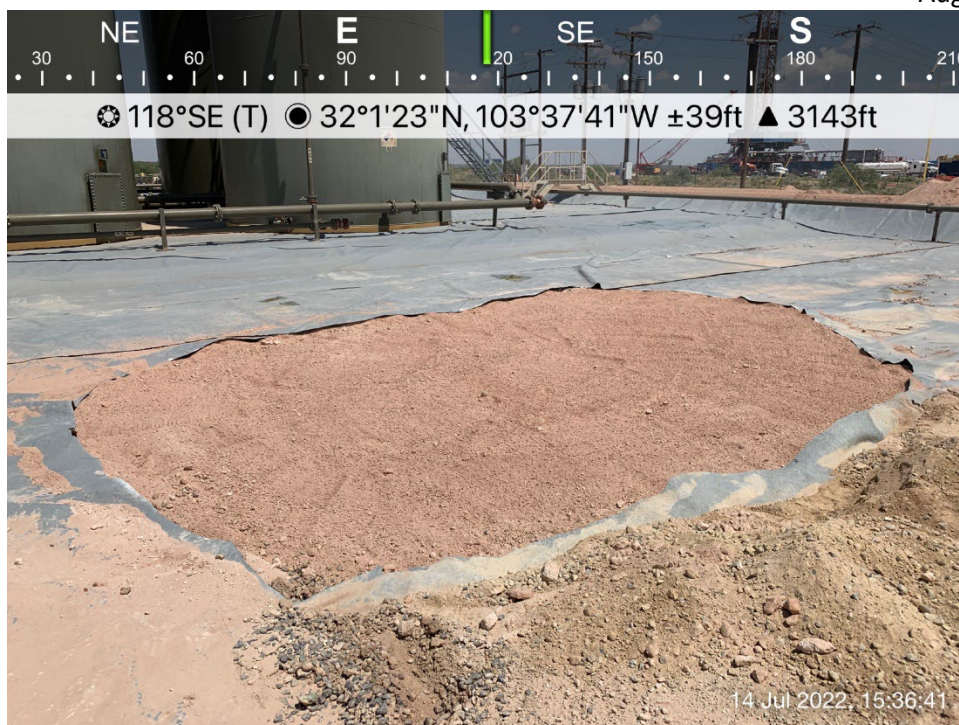
Backfilled excavation viewing southeast, July 14, 2022
