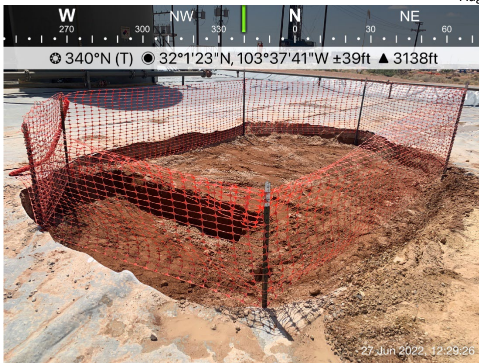
Excavated soil viewing North, June 27, 2022
