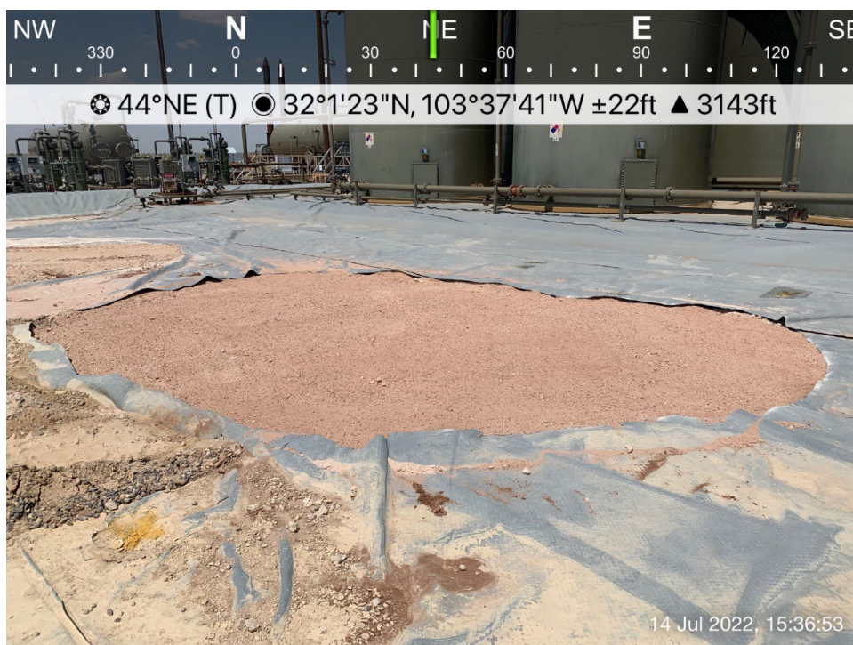
Backfilled excavation viewing southeast, July 14, 2022
