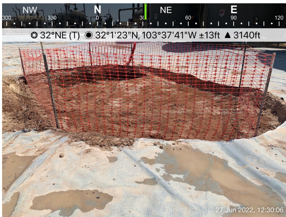
Excavated soil viewing Northeast, June 27, 2022
