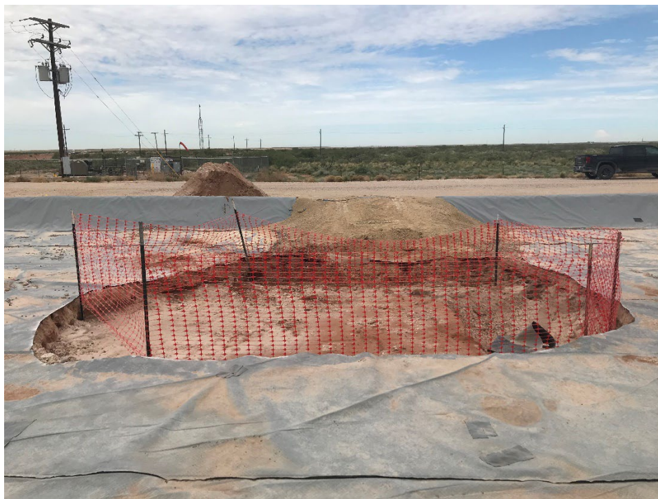
Additional soil excavated encompassing C-6 viewing west, July 6, 2022
