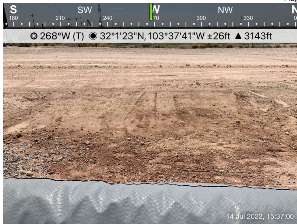
Impacted material and liner hauled to disposal viewing west, July 14, 2022
