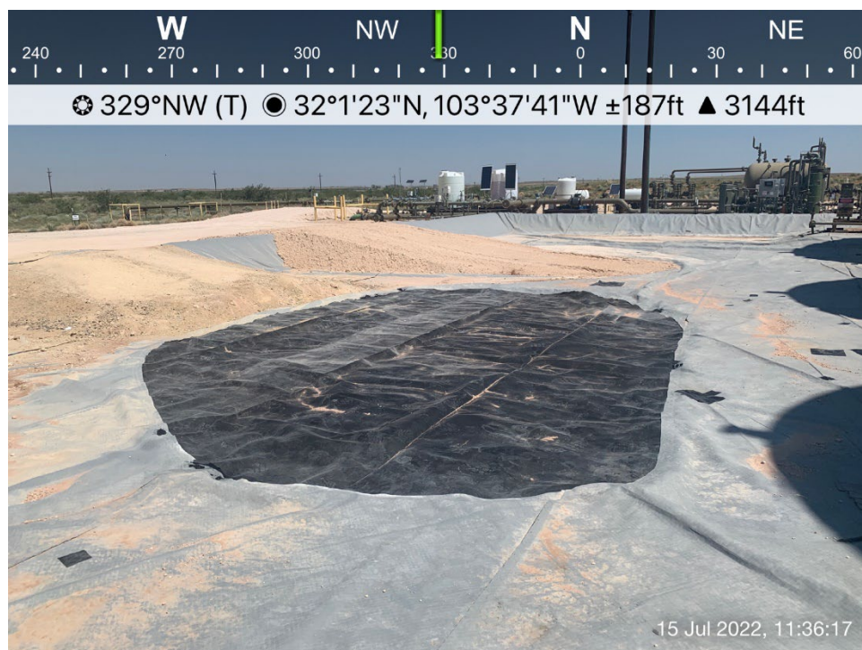
30-mil polyethylene liner replaced/repared viewing northeast, July 15, 2022
