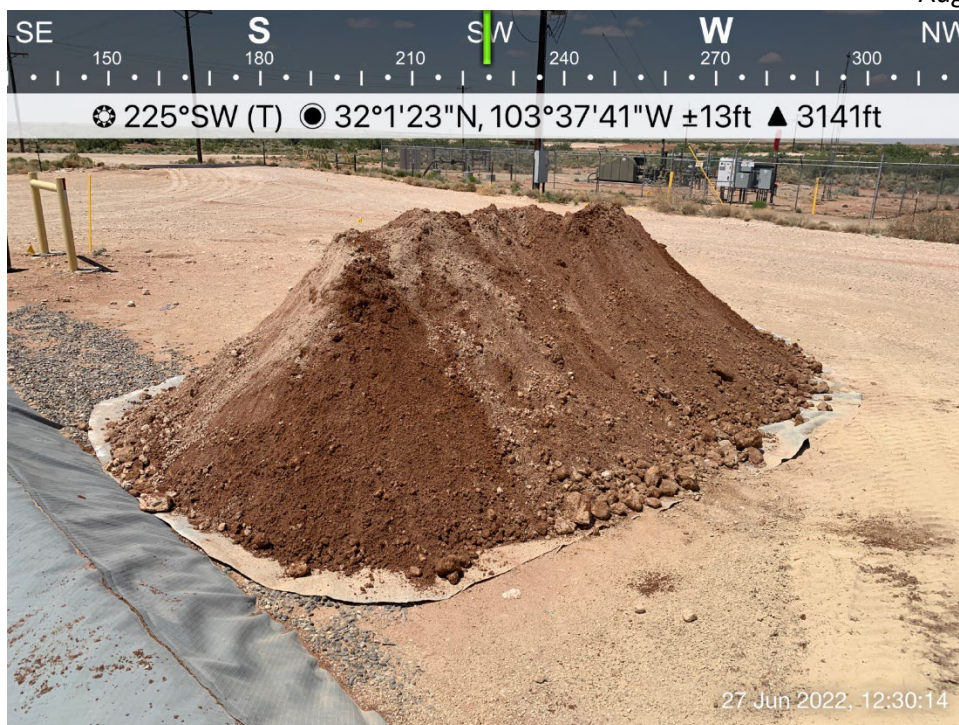
Impacted material stockpiled on a liner viewing southwest, June 27, 2022
