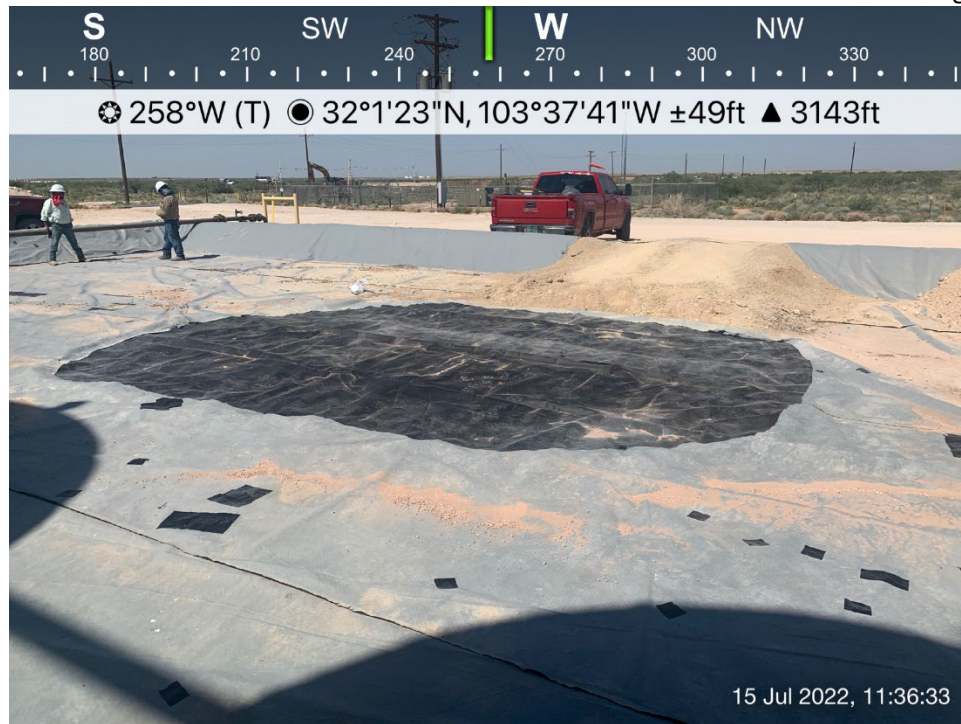
30-mil polyethylene liner replaced/repared viewing west, July 15, 2022
