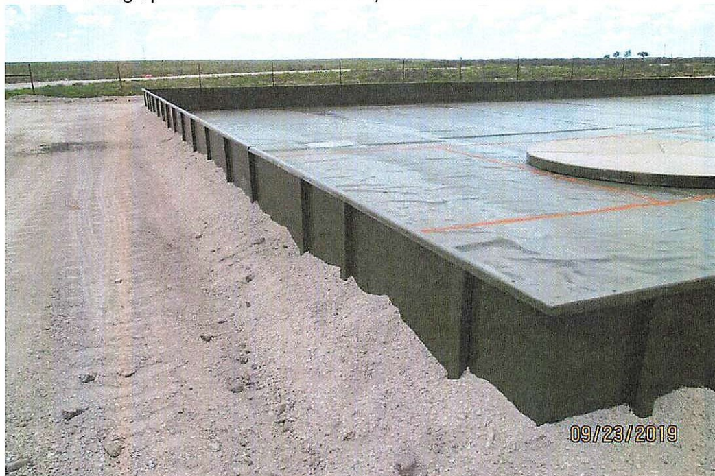
Photograph 7: Brand New Secondary Containment Structure Installed
