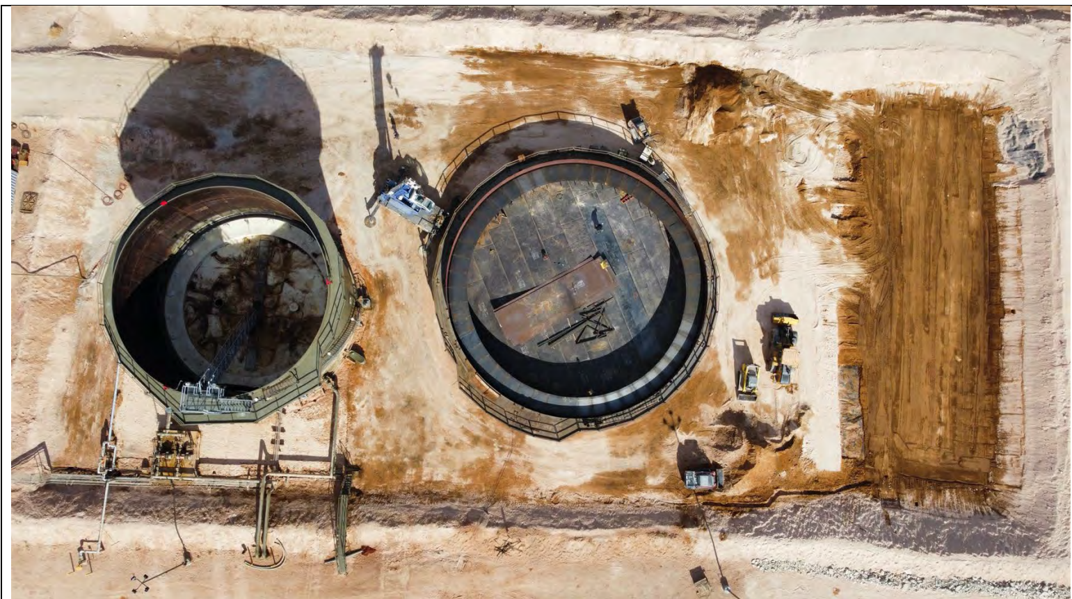
Photo 3 – Containment Berm After Initial Oil Recovery and During Initial Soil Removal
