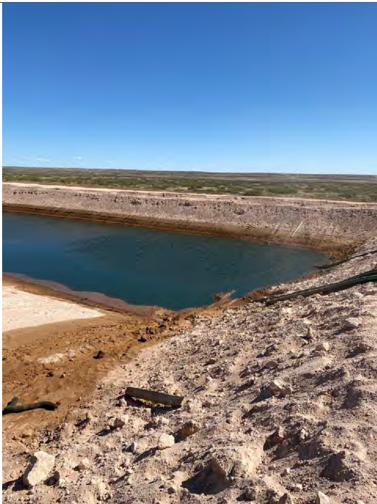
Photo 2: Containment Berm Sump within 24 Hours of Spill
