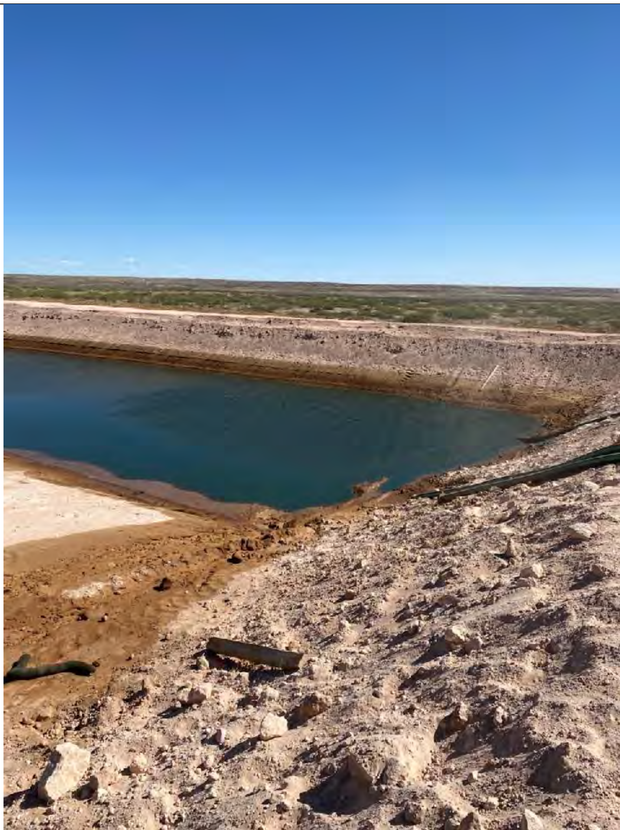
Photo 2: Containment Berm Sump within 24 Hours of Spill
