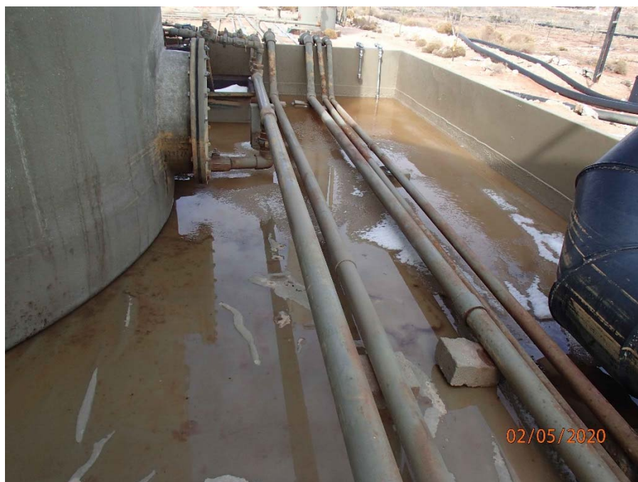
View of standing water and ice in the corner of the secondary containment.
