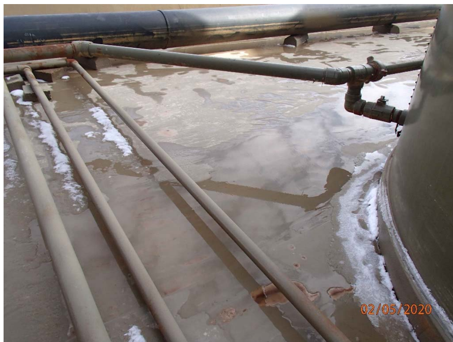
View of standing water and ice within the secondary containment.
