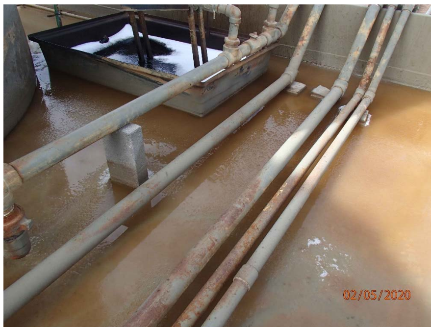
View of frozen standing water in the corner of the secondary containment.
