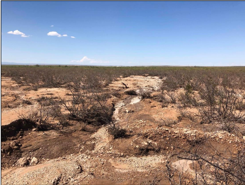
PHOTO 28: View of excavation facing HA-2, facing northwest. 9/26/2019
