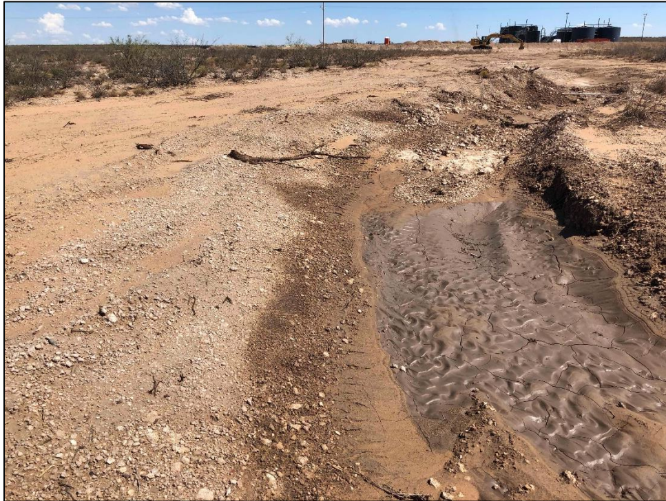
PHOTO 32: View of excavation facing HA-4, facing east. 9/26/2019
