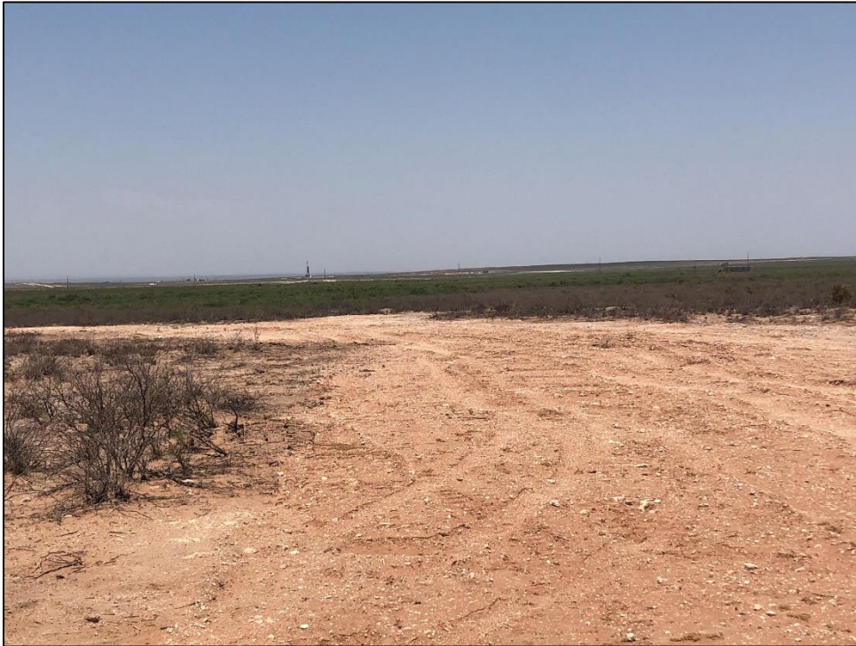
PHOTO 23: View of completed remediation in natural drainage area, facing west. 6/22/2020
