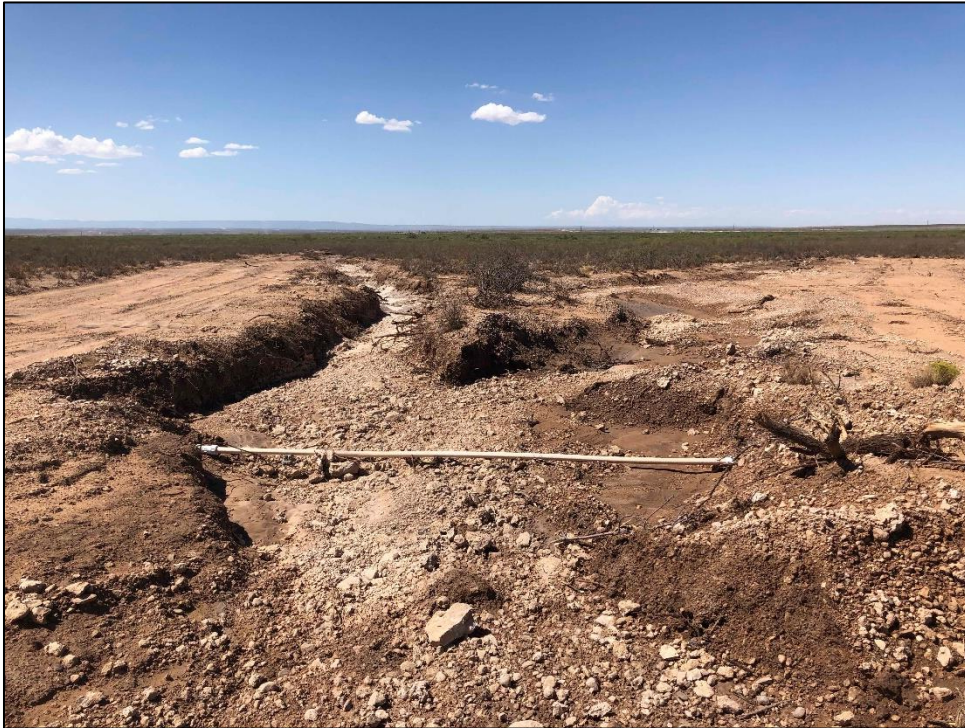
PHOTO 24: View of excavation, facing west. 9/26/2019
