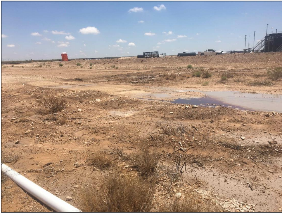
PHOTO 3: View of sight and staining (non reportable), facing northeast. 6/04/2019
