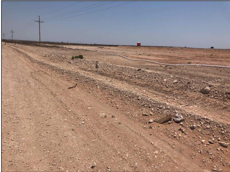
PHOTO 21: View of completed remediation, facing northeast. 6/22/2020
