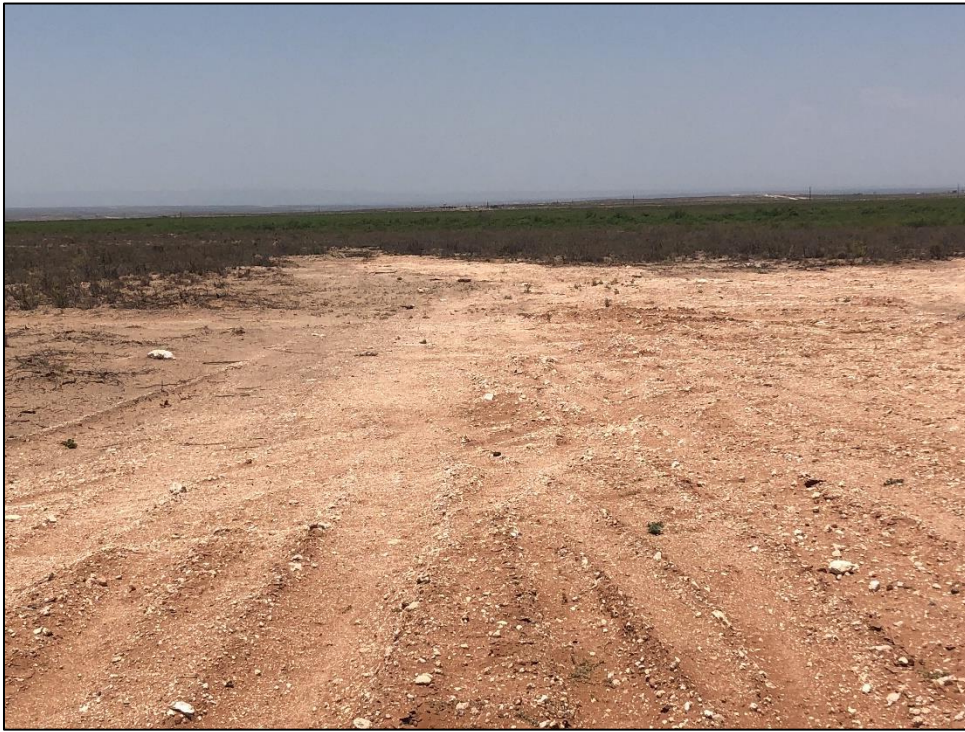
PHOTO 24: View of completed remediation toward HA-1, facing west. 6/22/2020
