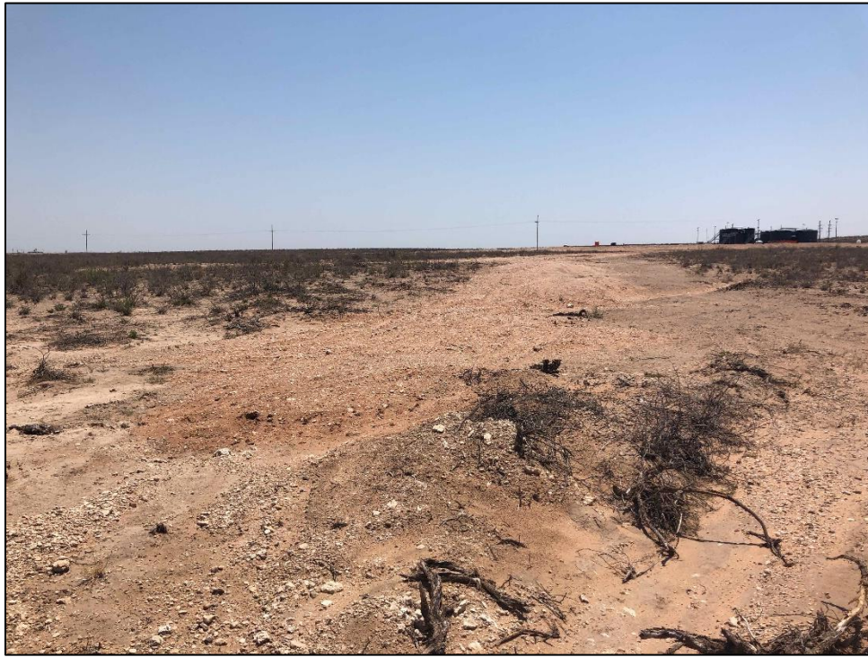
PHOTO 28: View of completed remediation from HA-1, facing east. 6/22/2020
