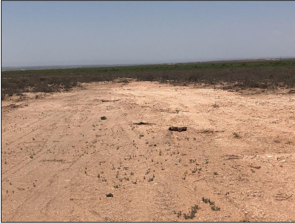
PHOTO 26: View of completed remediation toward HA-2, facing west. 6/22/2020
