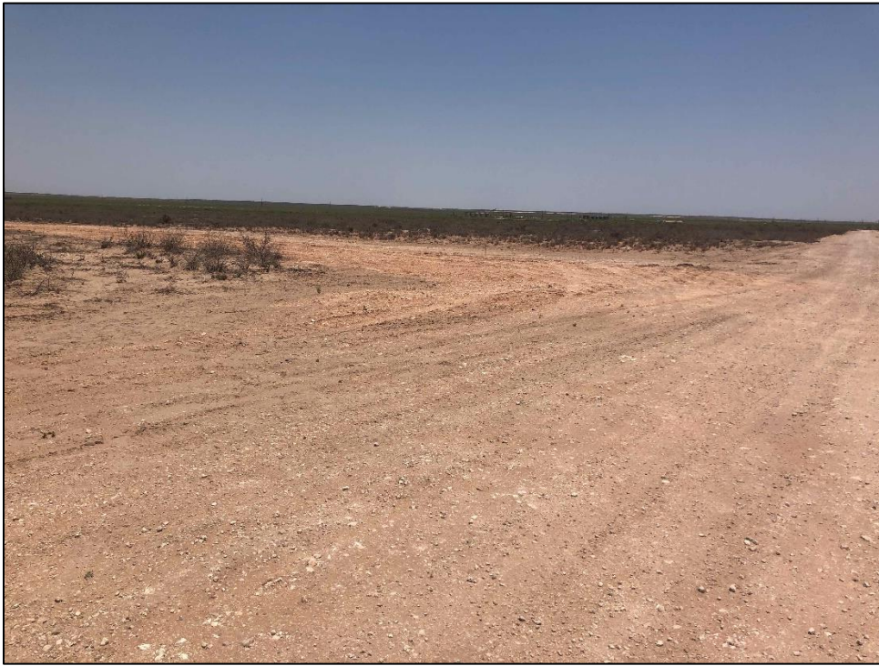
PHOTO 22: View of completed remediation in natural drainage area, facing north. 6/22/2020
