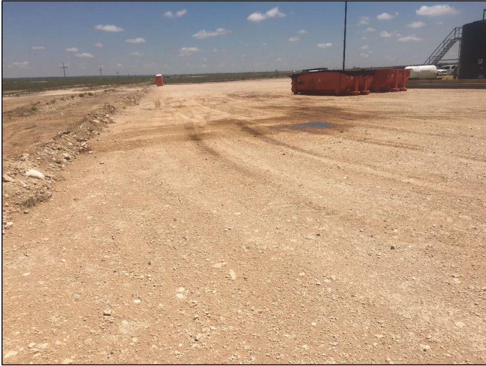
PHOTO 7: View of staining on pad (non-reportable), facing north. 6/04/2019
