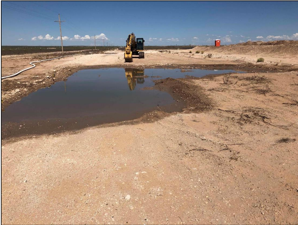
PHOTO 20: View of excavation full post rainfall, facing north. 9/26/2019
