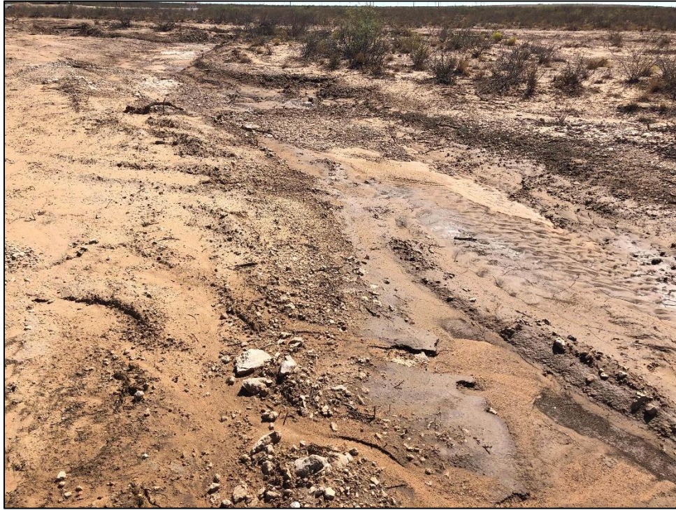
PHOTO 31: View of excavation from HA-2, facing southeast. 9/26/2019
