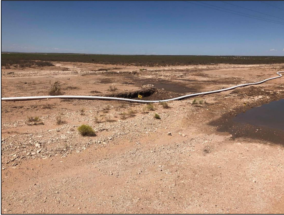
PHOTO 21: View of excavation going into natural drainage, facing northwest. 9/26/2019
