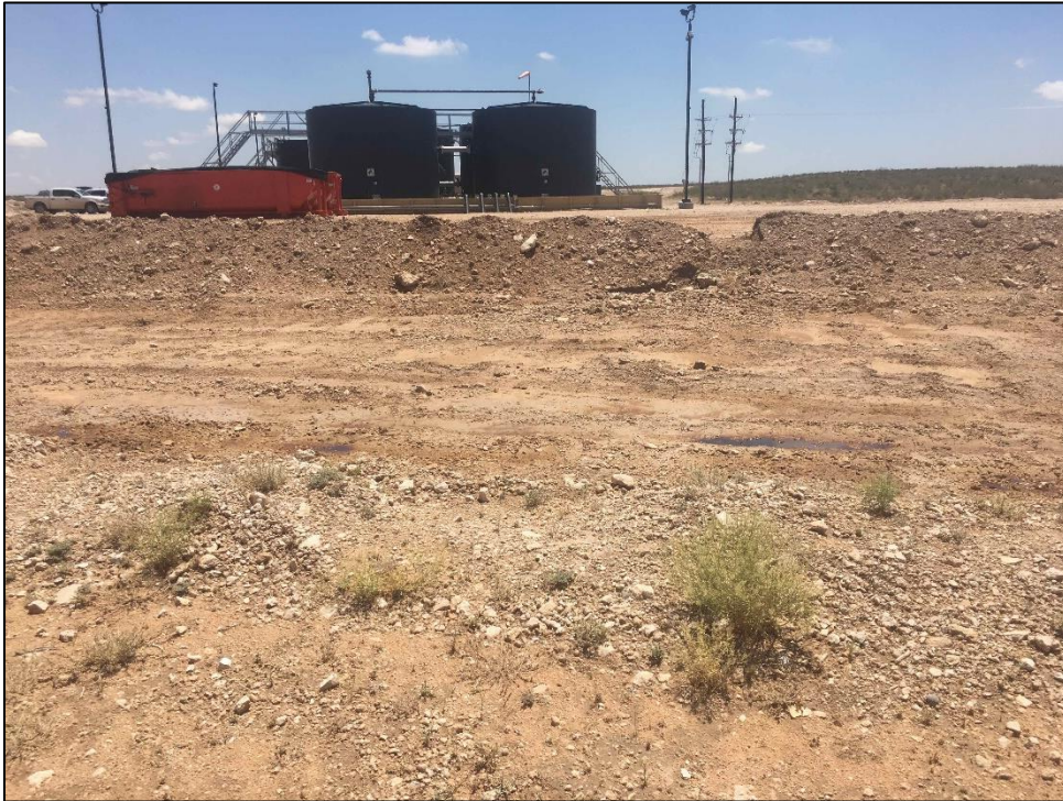
PHOTO 6: View of staining and flow path off pad (non-reportable), facing east. 6/04/2019
