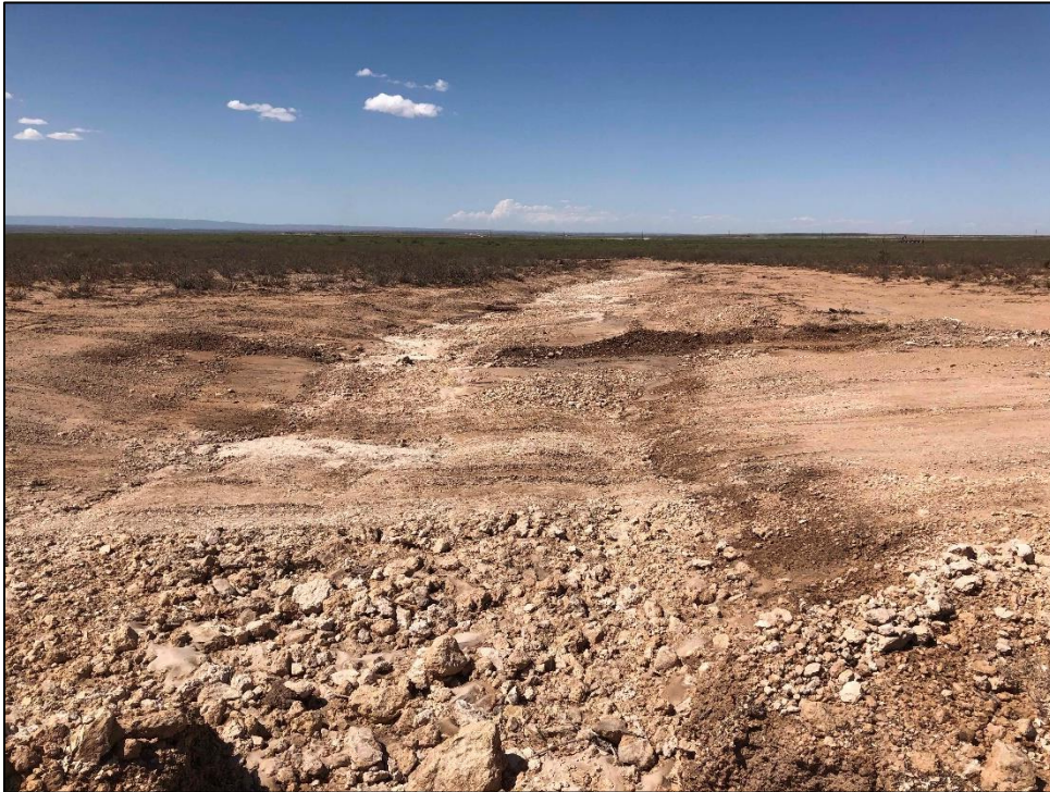
PHOTO 22: View of excavation in natural drainage area, facing west. 9/26/2019
