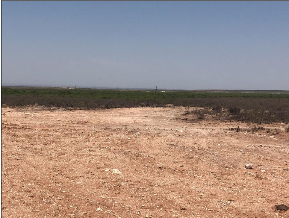
PHOTO 25: View of completed remediation toward HA-3, facing northwest. 6/22/2020
