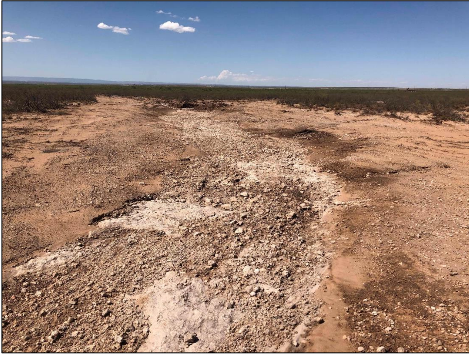
PHOTO 23: View of excavation from HA-4, facing west. 9/26/2019
