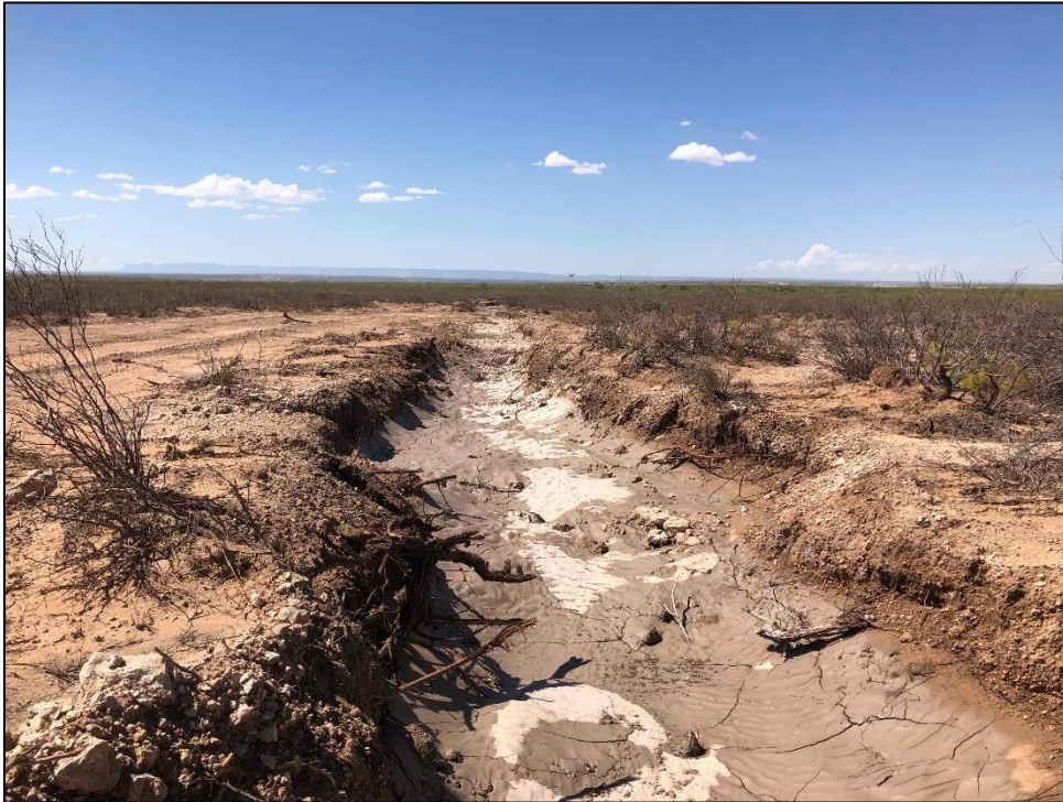
PHOTO 26: View of excavation on south fork, facing west. 9/26/2019
