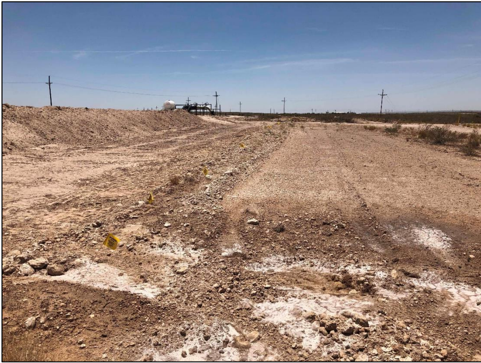
PHOTO 9: View of sight and staining, facing south. 7/15/2019
