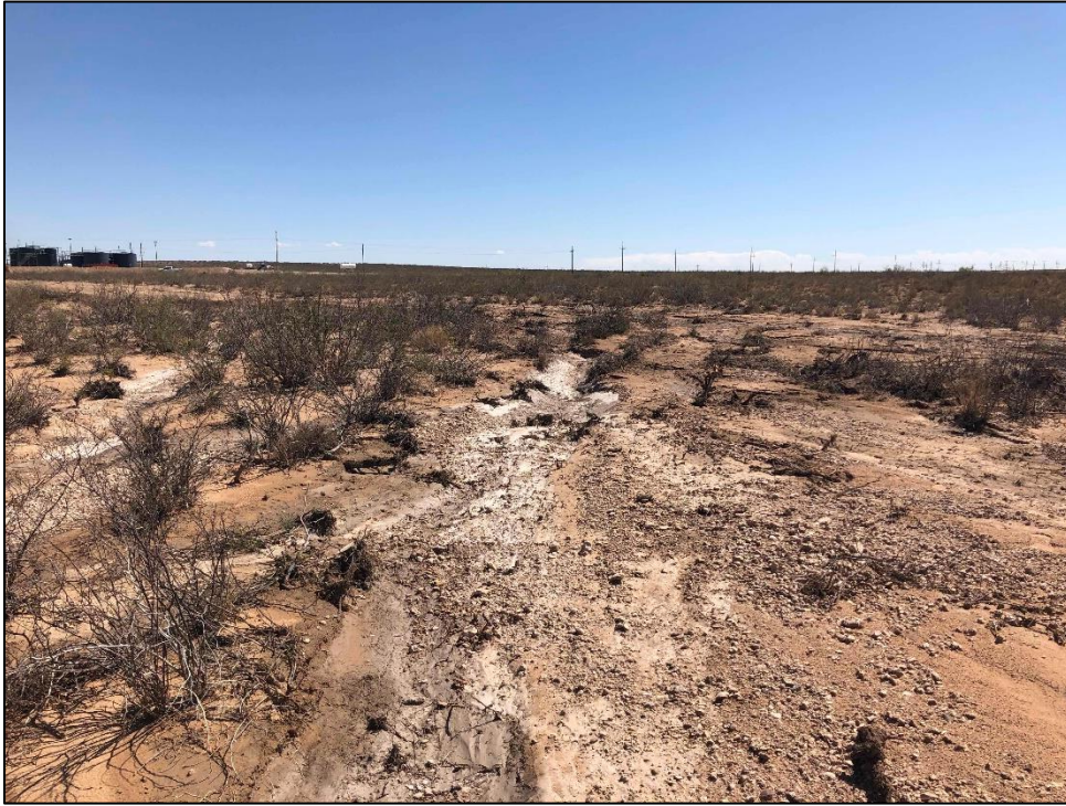
PHOTO 29: View of end of excavation facing HA-1, facing west. 9/26/2019
