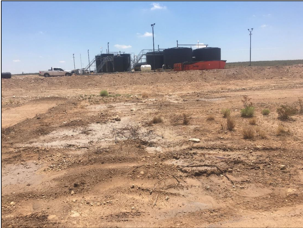
PHOTO 4: View of sight and staining (non-reportable), facing east. 6/04/2019
