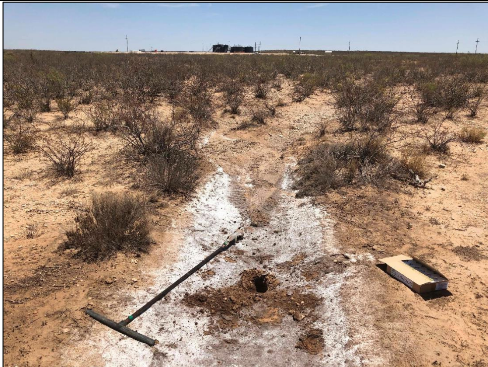
PHOTO 14: View of staining and HA-1, facing east. 7/15/2019
