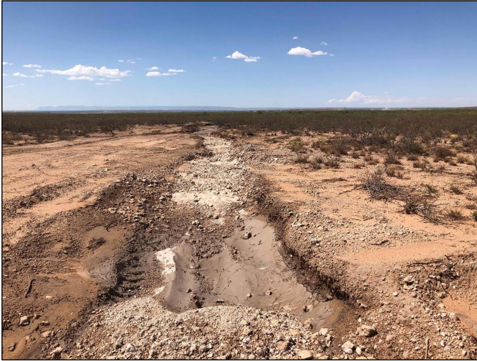
PHOTO 27: View of excavation on southern fork continued, facing west. 9/26/2019
