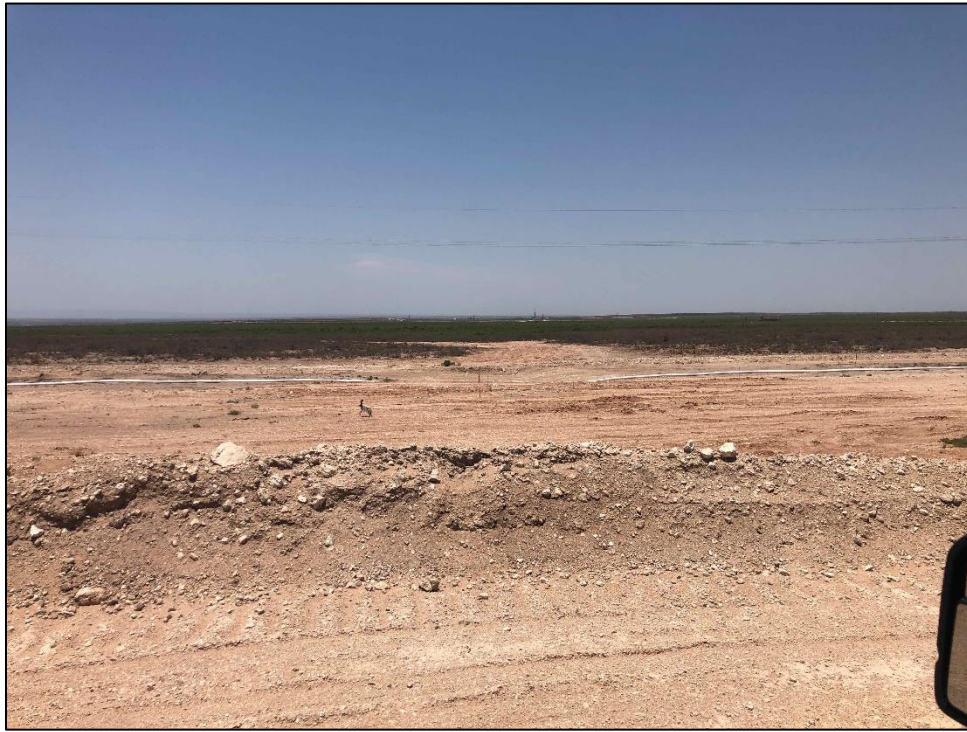
PHOTO 30: View of completed remediation, facing west. 6/22/2020
