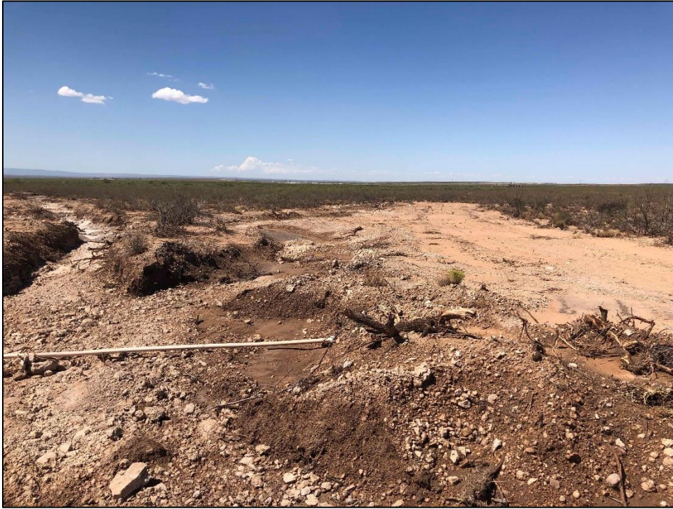
PHOTO 25: View of excavation toward HA-3, facing northwest. 9/26/2019
