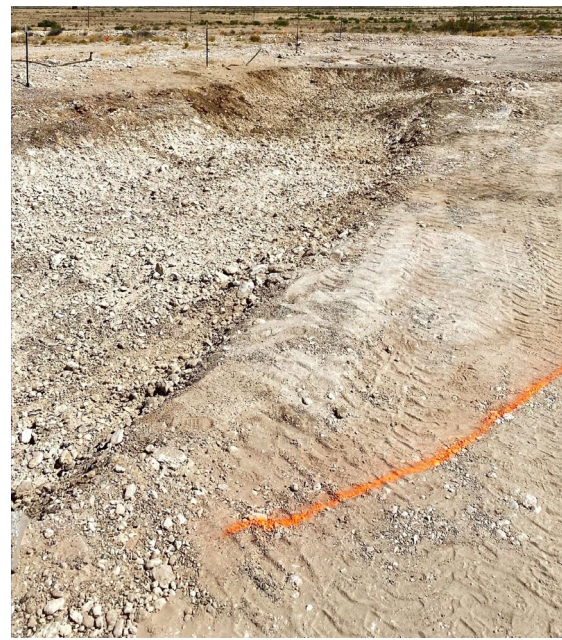
Photograph 4 Date: 26-May-22 Description: Beginning of excavation facing north.
