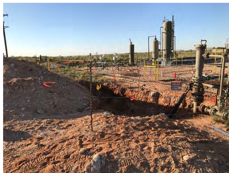
Photograph 12: View of open excavation (2RP-4398), facing northwest.
