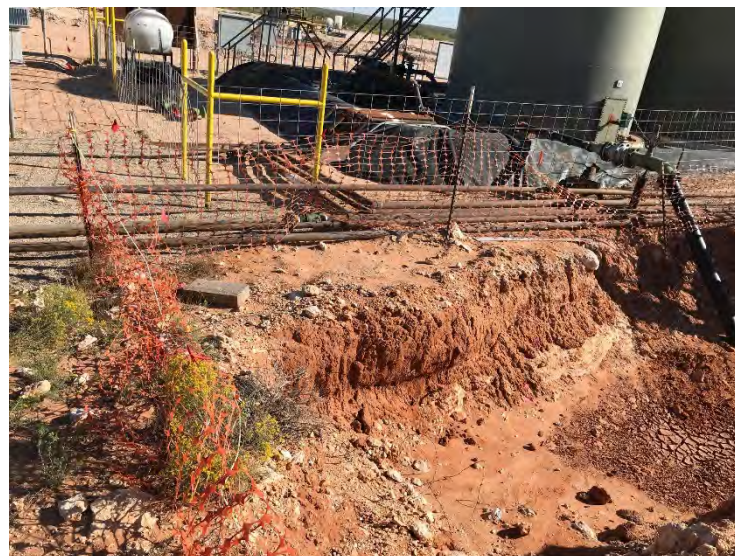
Photograph 10: View of open excavation (2RP-4398), facing north.
