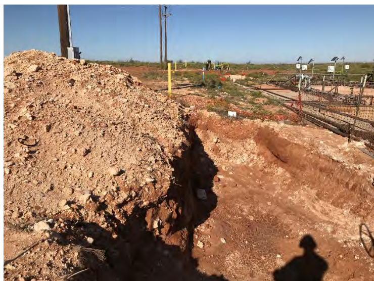
Photograph 11: View of open excavation (2RP-4398), facing west.
