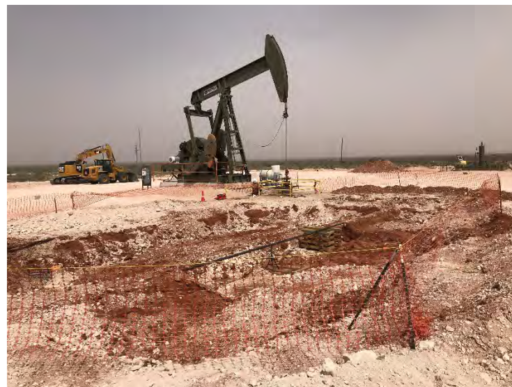
Photograph 4: View of excavation (2RP-2526), facing northeast.
