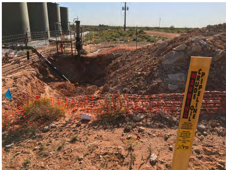
Photograph 9: View of open excavation (2RP-4398), facing east.
