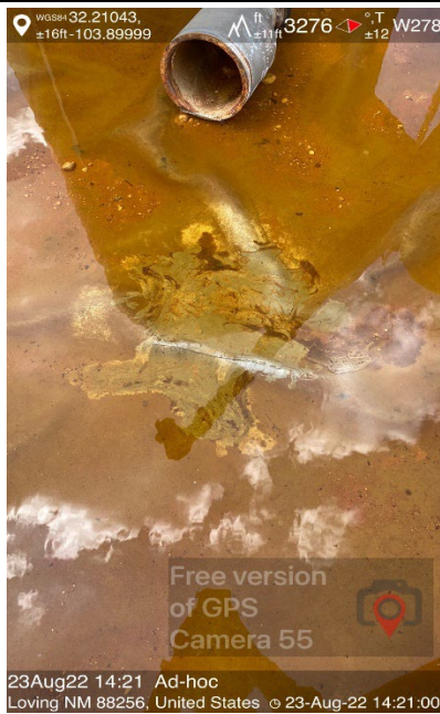
Photograph 3 Date: Aug 23, 2022 Description: View of liner patch. The patch is holding water following a recent rain.
