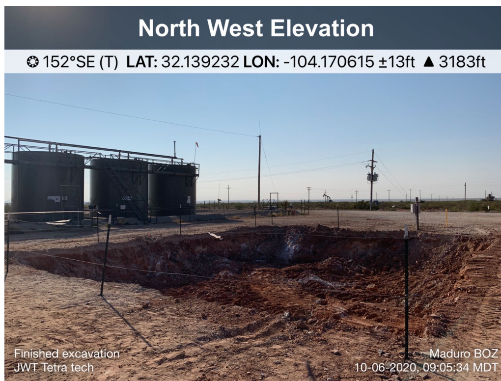
View of Remediation – View Northwest
