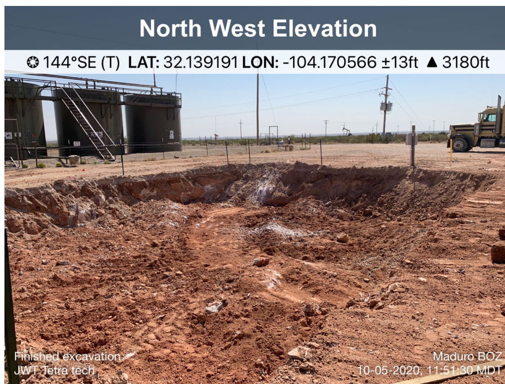
View of Remediation Activities – View Northwest
