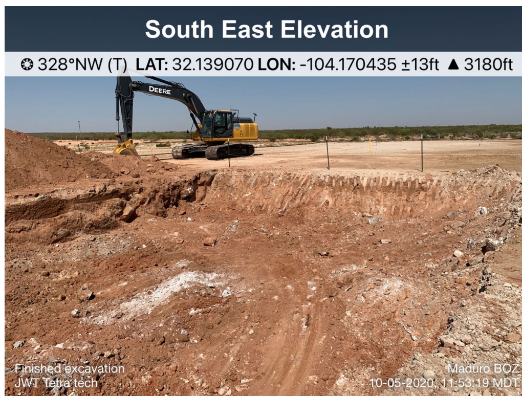
View of Remediation Activities – View Southeast
