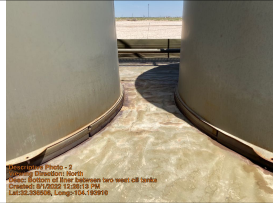
Bottom of liner between two west oil tanks
