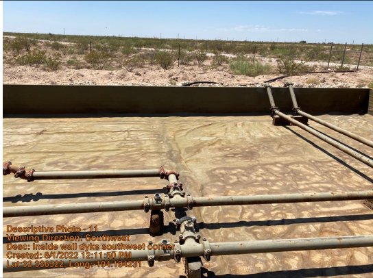
Inside wall dyke southwest corner
