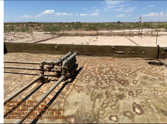
Inside wall dyke west end
