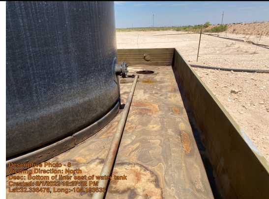
Bottom of liner east of water tank
