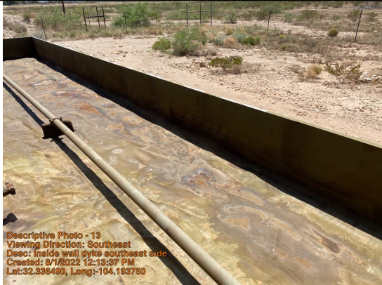
Inside wall dyke southeast side
