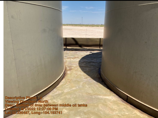
Bottom of liner between middle oil tanks
