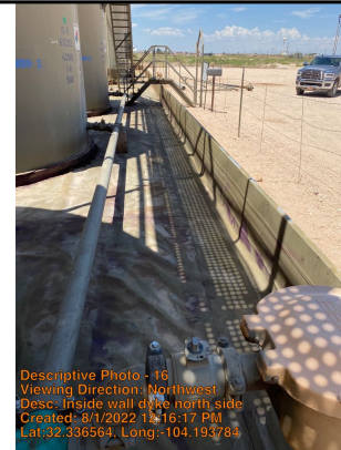
Inside wall dyke north side
