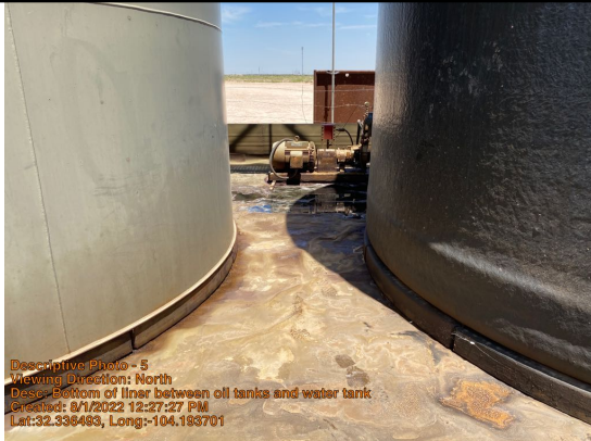
Bottom of liner between oil tanks and water tank
