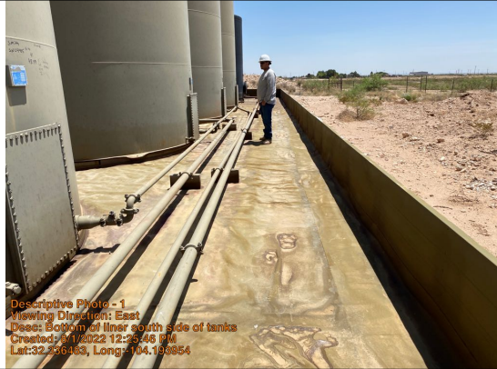
Bottom of liner south side of tanks
