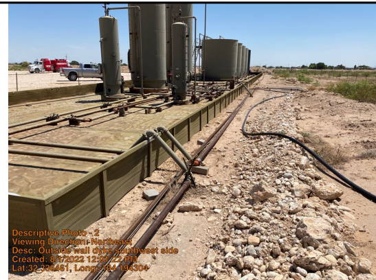
Outside wall dyke southwest side
