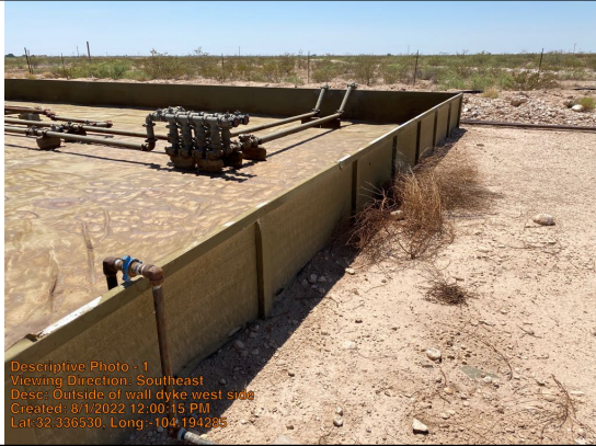
Outside of wall dyke west side
