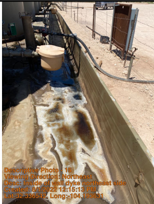
Inside of wall dyke northeast side
