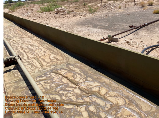
Inside wall dyke south side
