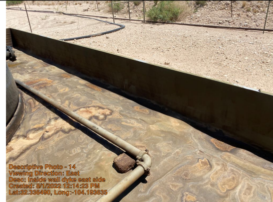
Inside wall dyke east side
