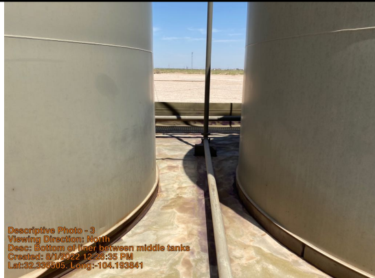
Bottom of liner between middle tanks
