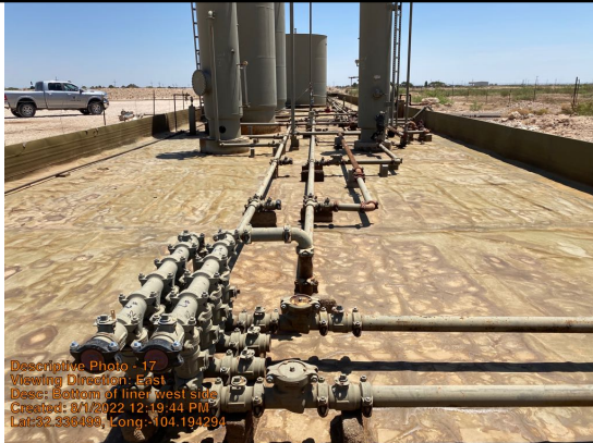
Bottom of liner west side
