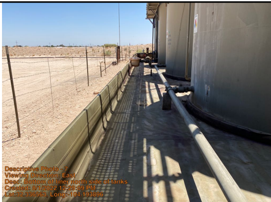
Bottom of liner north side of tanks
