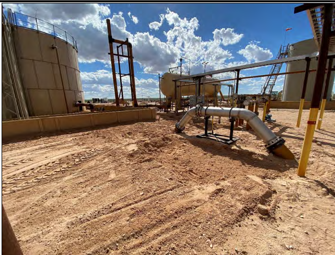
PHOTO 6: View of the excavated area facing southwest. 9/29/22
