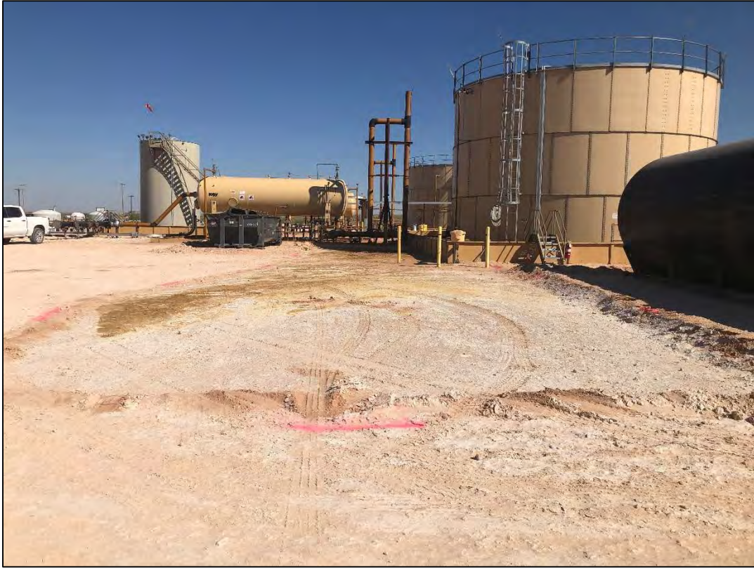
PHOTO 1: View of the impacted area facing north. 9/29/22
