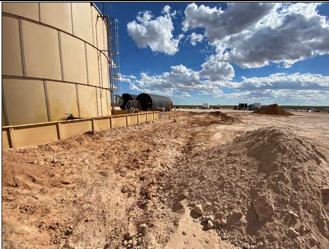
PHOTO 5: View of the excavated area facing southwest. 9/29/22
