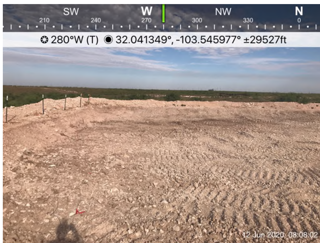
View of Remediation Activities – View West
