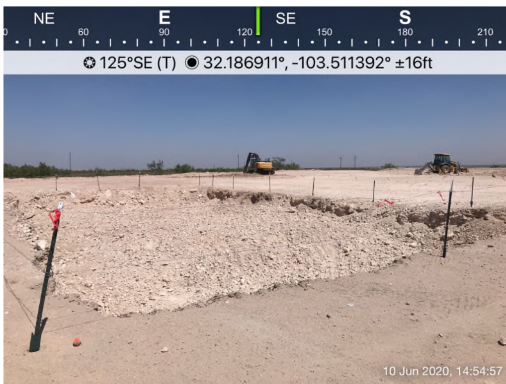
View of Remediation Activities – View Southeast
