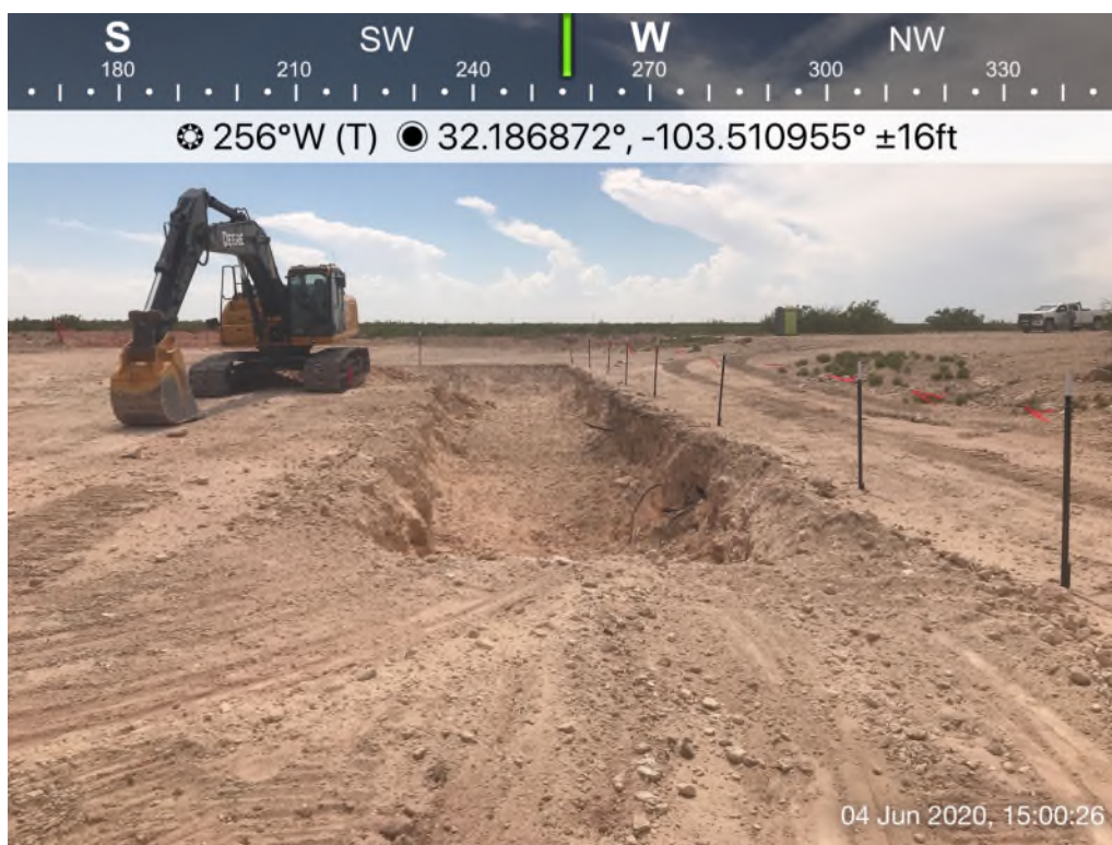
View of Remediation Activities – View West
