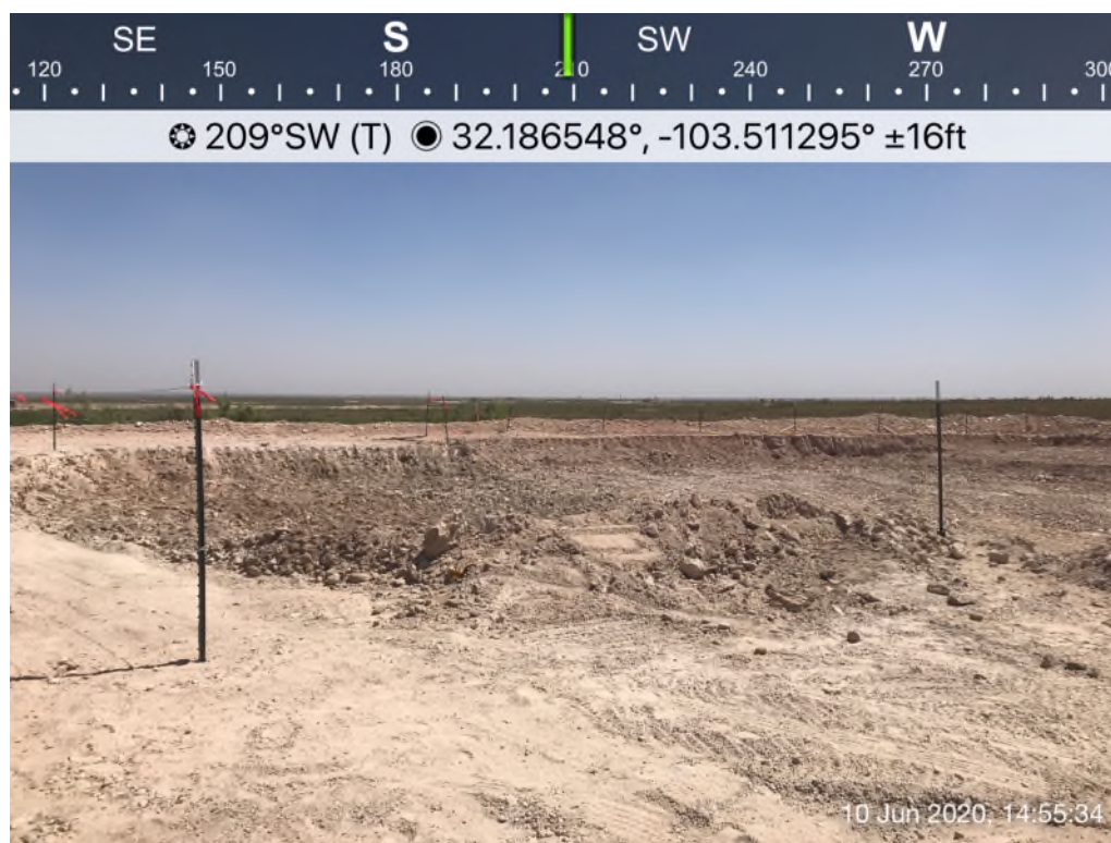
View of Remediation Activities – View Southwest
