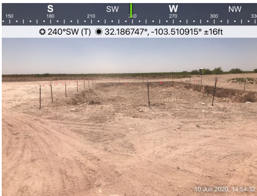
View of Remediation Activities – View Southwest
