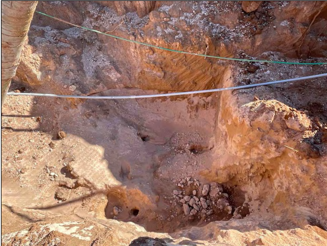
PHOTO 14: View of the additionally excavated area, associated with sample area CS-15, under the riser facing south. 11/28/22
