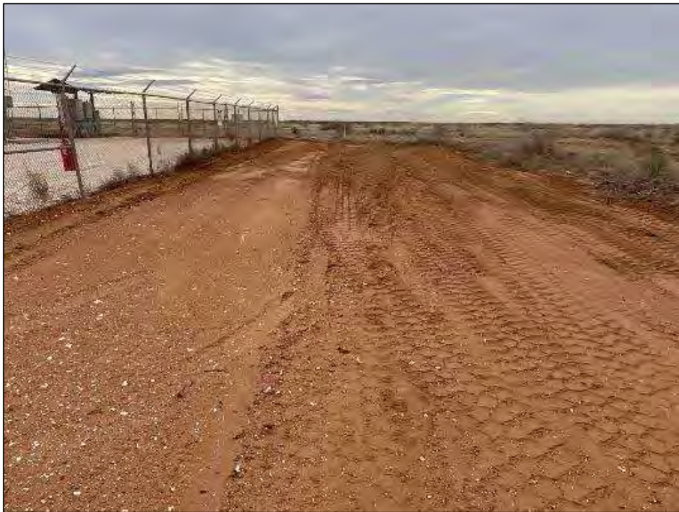
PHOTO 20: View of the remediated and backfilled native soil area west of the riser area facing south. 1/3/23
