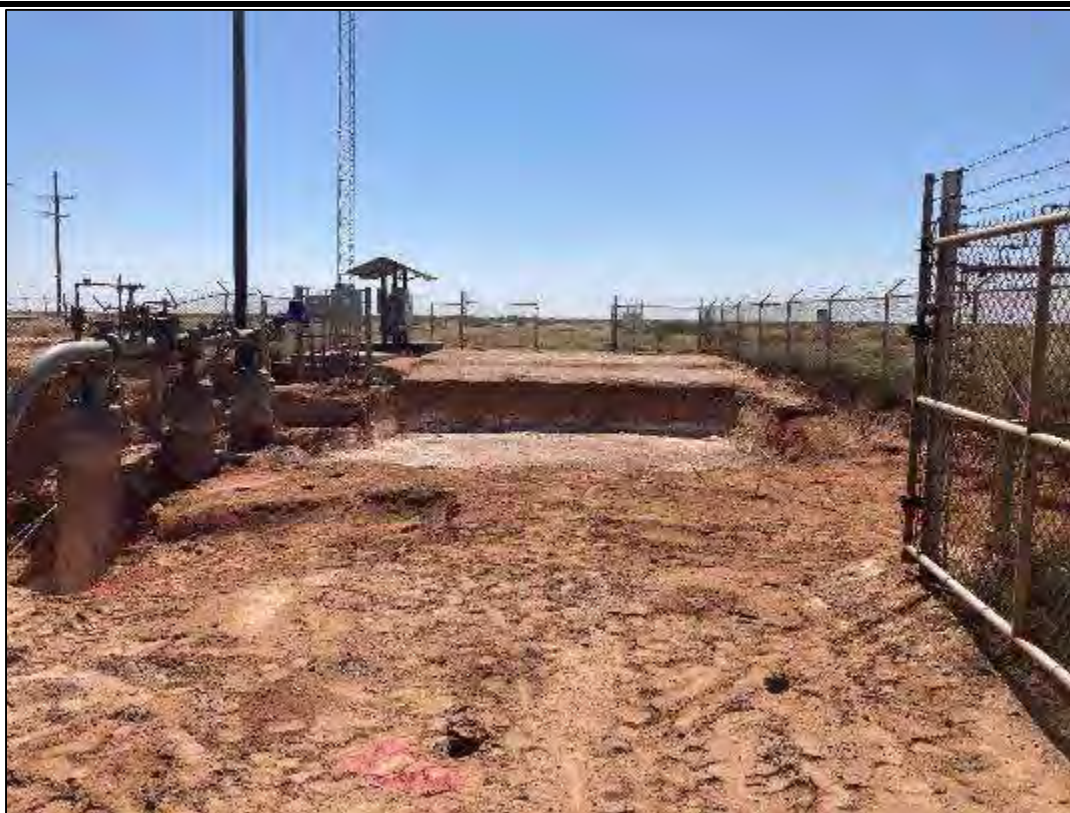
PHOTO 10: View of the excavated area facing south. 10/12/22
