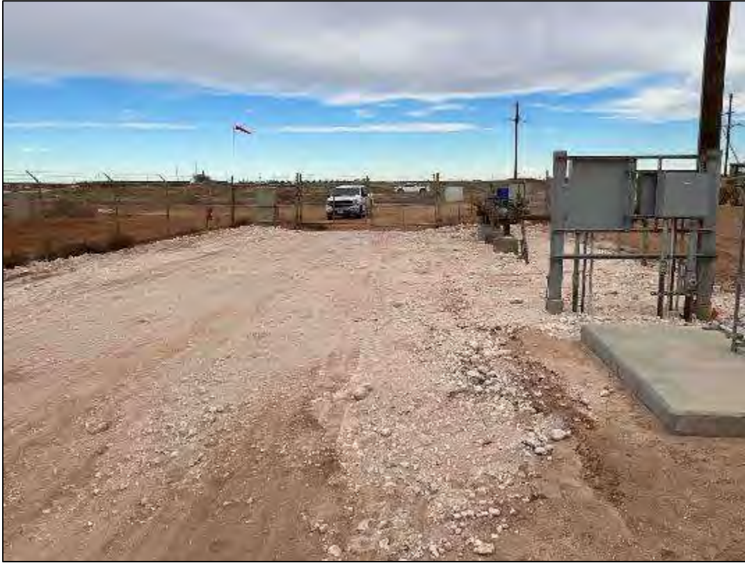
PHOTO 17: View of the remediated and backfilled area within the riser security fence facing north. 1/3/23
