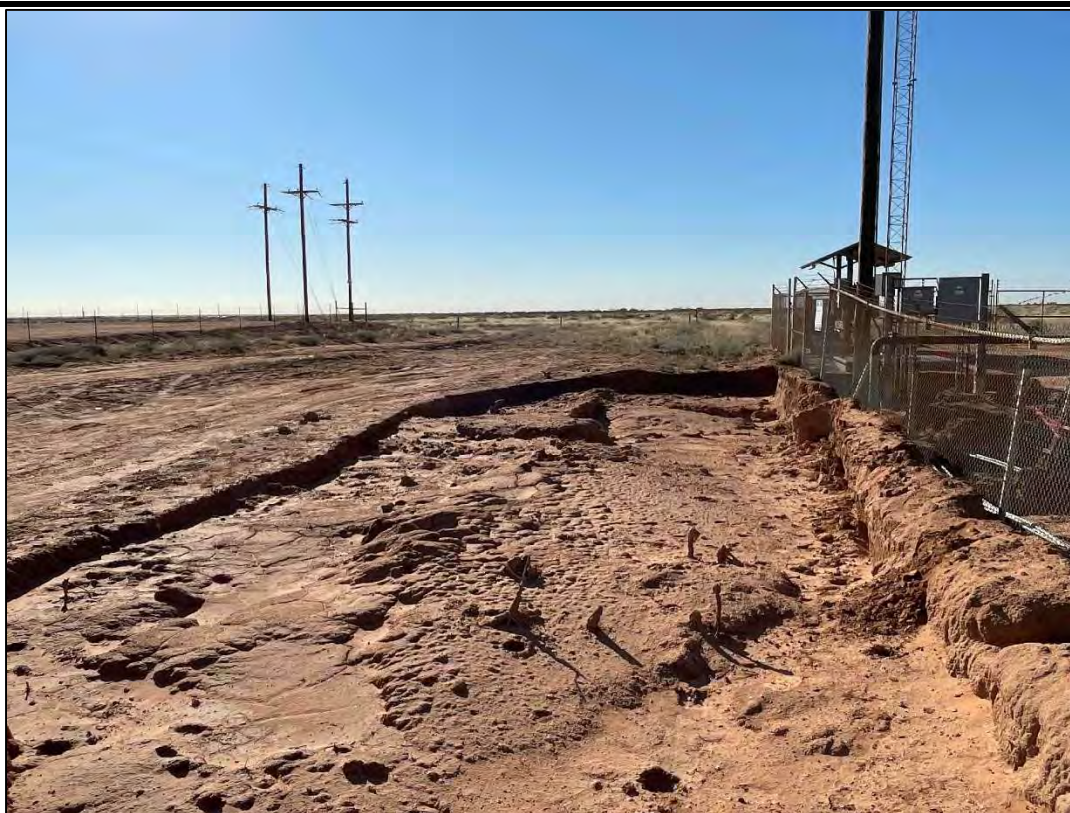
PHOTO 16: View of the additionally excavated area, associated with sample area CS-20 and CS-21, facing south. 11/28/22
