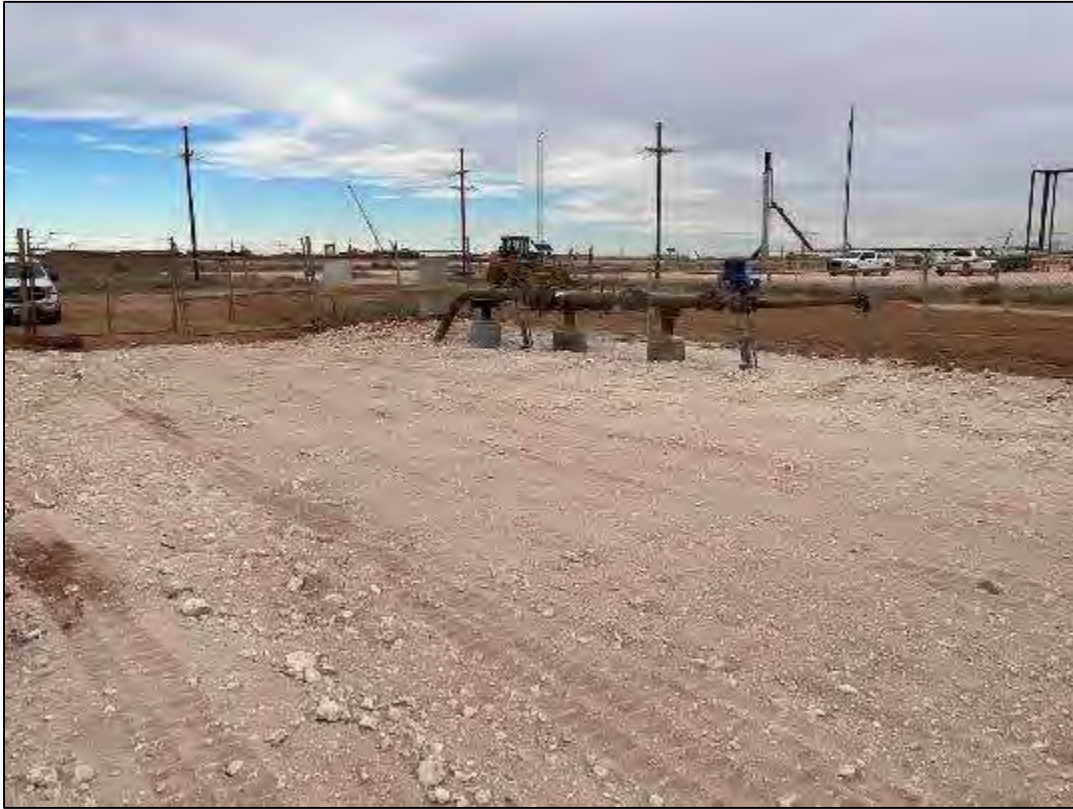
PHOTO 19: View of the remediated and backfilled area within the riser security fence facing northeast. 1/3/23
