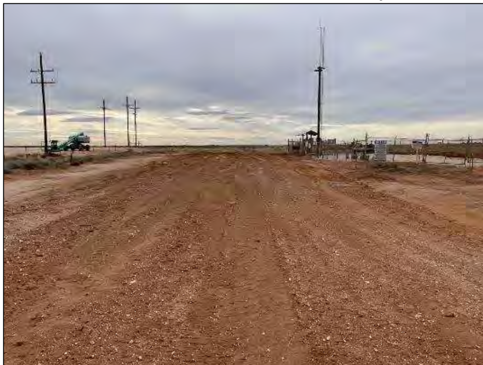
PHOTO 22: View of the remediated and backfilled native soil area east of the riser area facing south. 1/3/23
