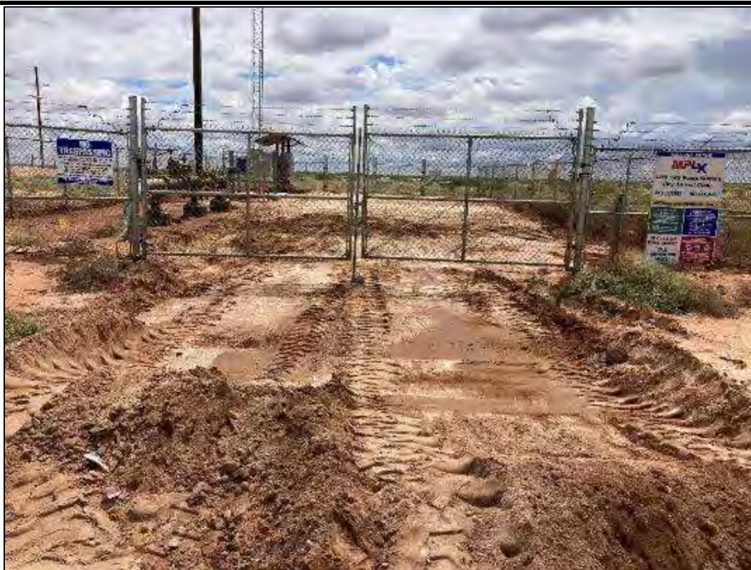
PHOTO 6: View of the excavated area facing south. 8/30/22
