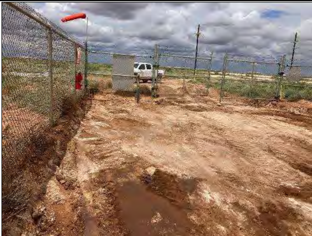
PHOTO 7: View of the excavated area facing north. 8/30/22
