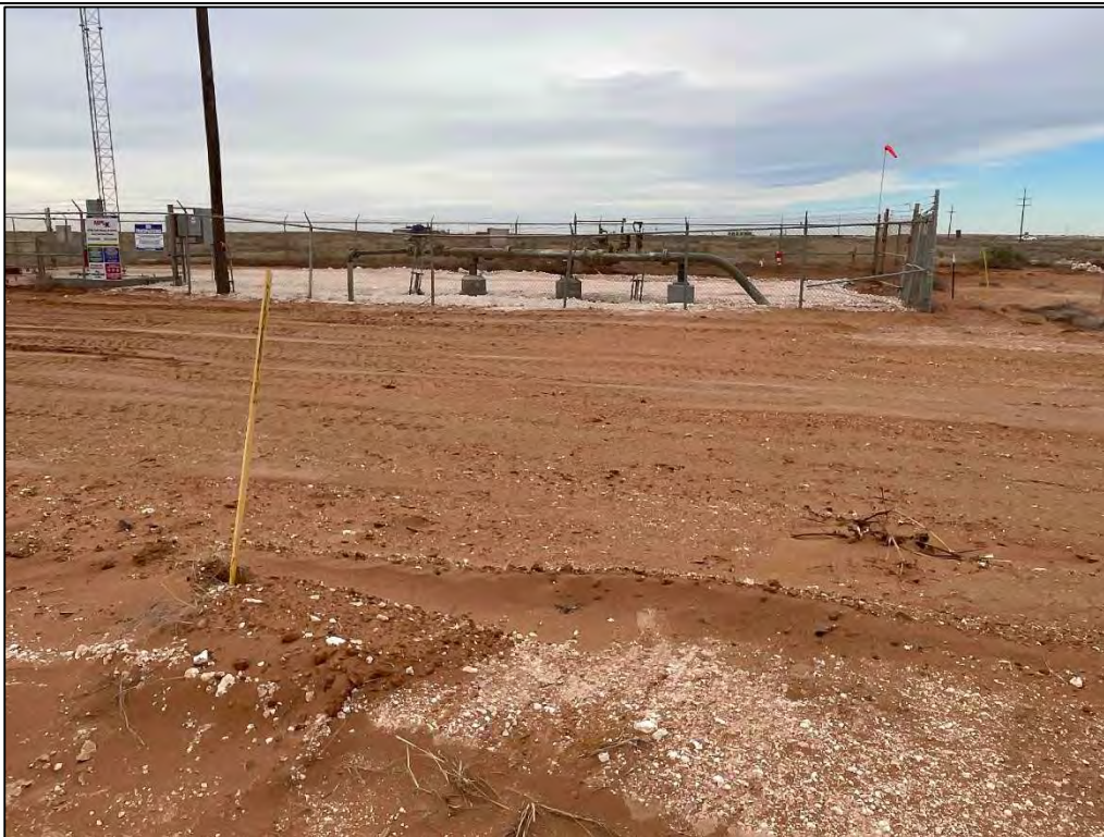
PHOTO 21: View of the remediated and backfilled native soil area east of the riser area facing west. 1/3/23
