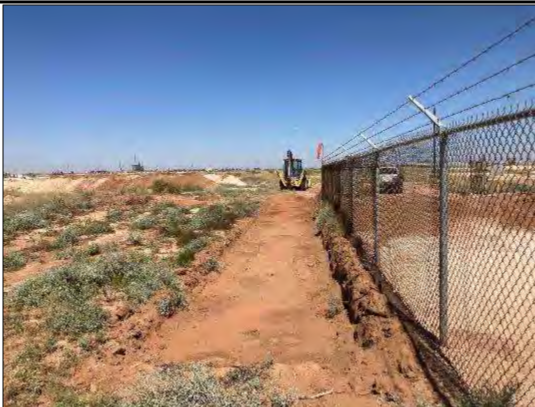
PHOTO 12: View of the excavated area facing north. 10/12/22
