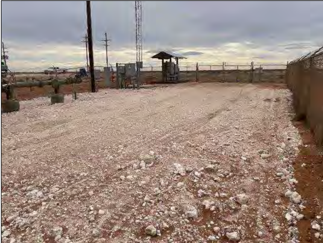
PHOTO 18: View of the remediated and backfilled area within the riser security fence facing southeast. 1/3/23
