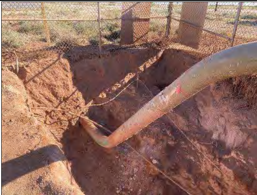
PHOTO 9: View of the excavated area facing northeast. 9/30/22
