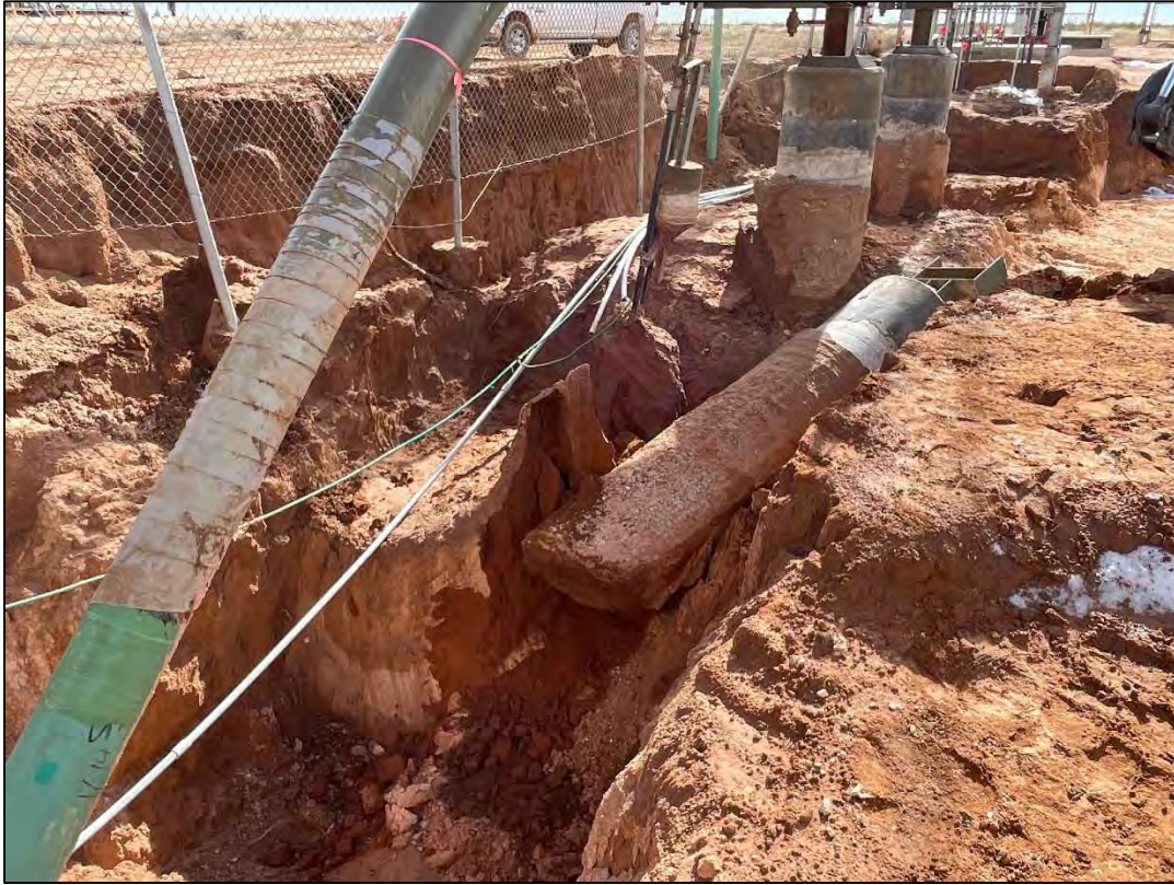
PHOTO 13: View of the additionally excavated area, associated with sample area CS-15, under the riser facing south. 11/28/22
