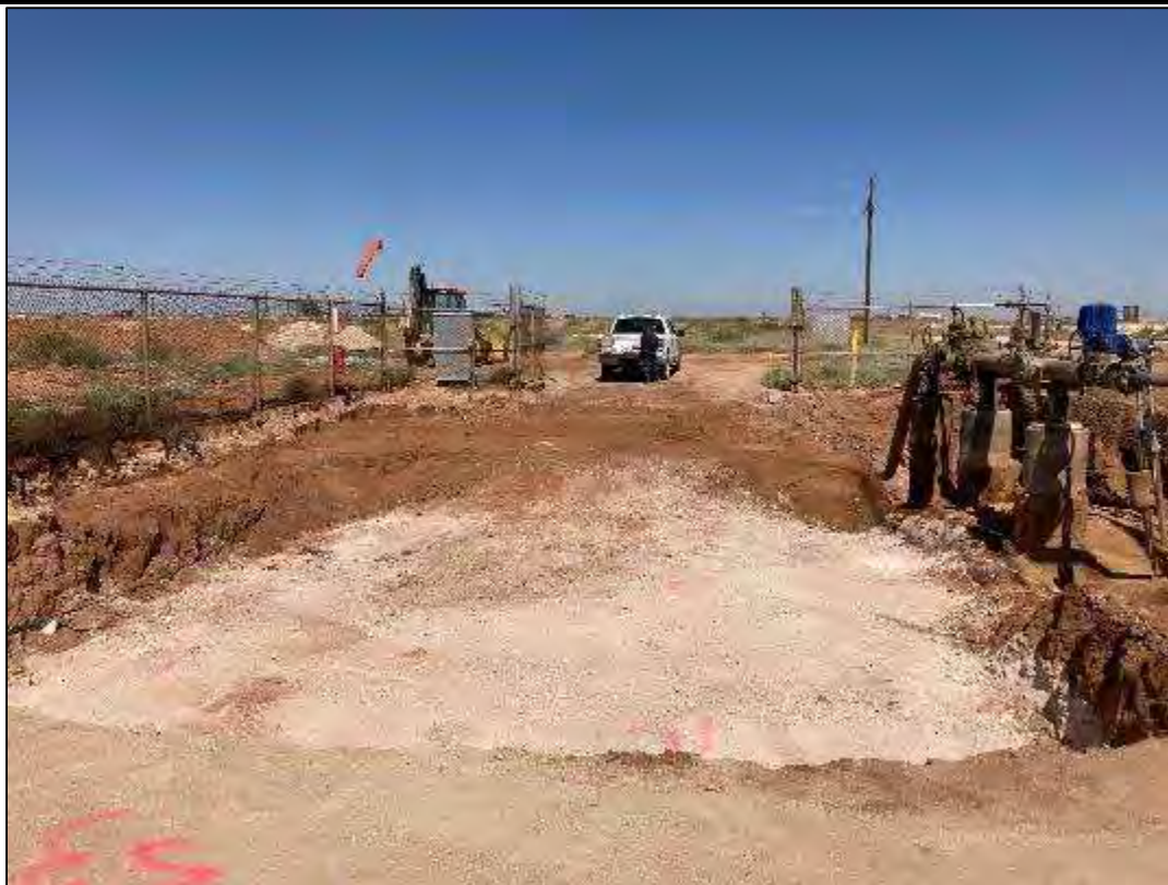
PHOTO 11: View of the excavated area facing north. 10/12/22
