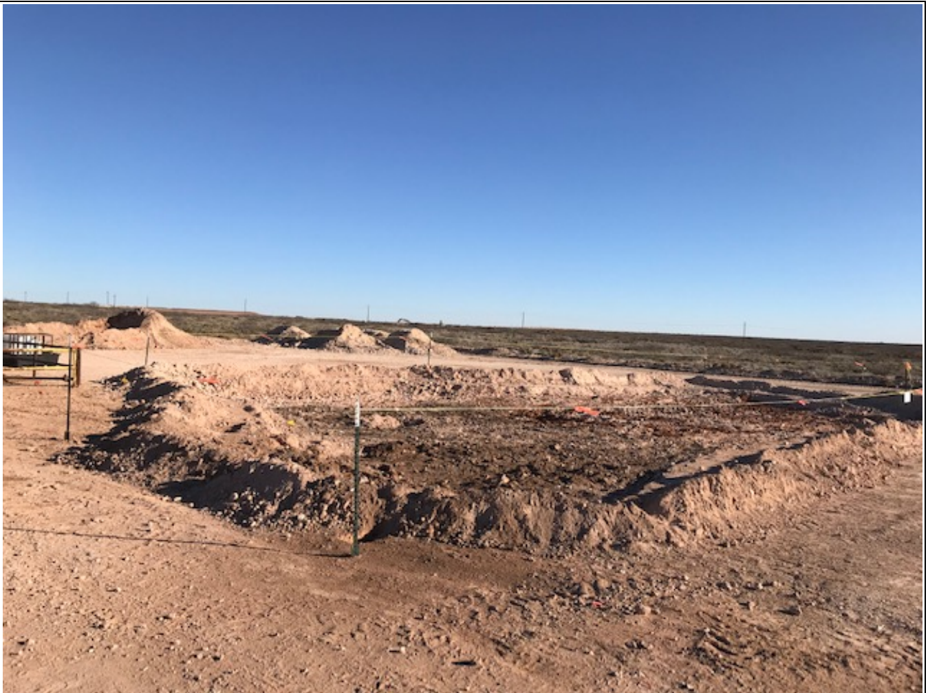
View facing southeast of the open excavation.
