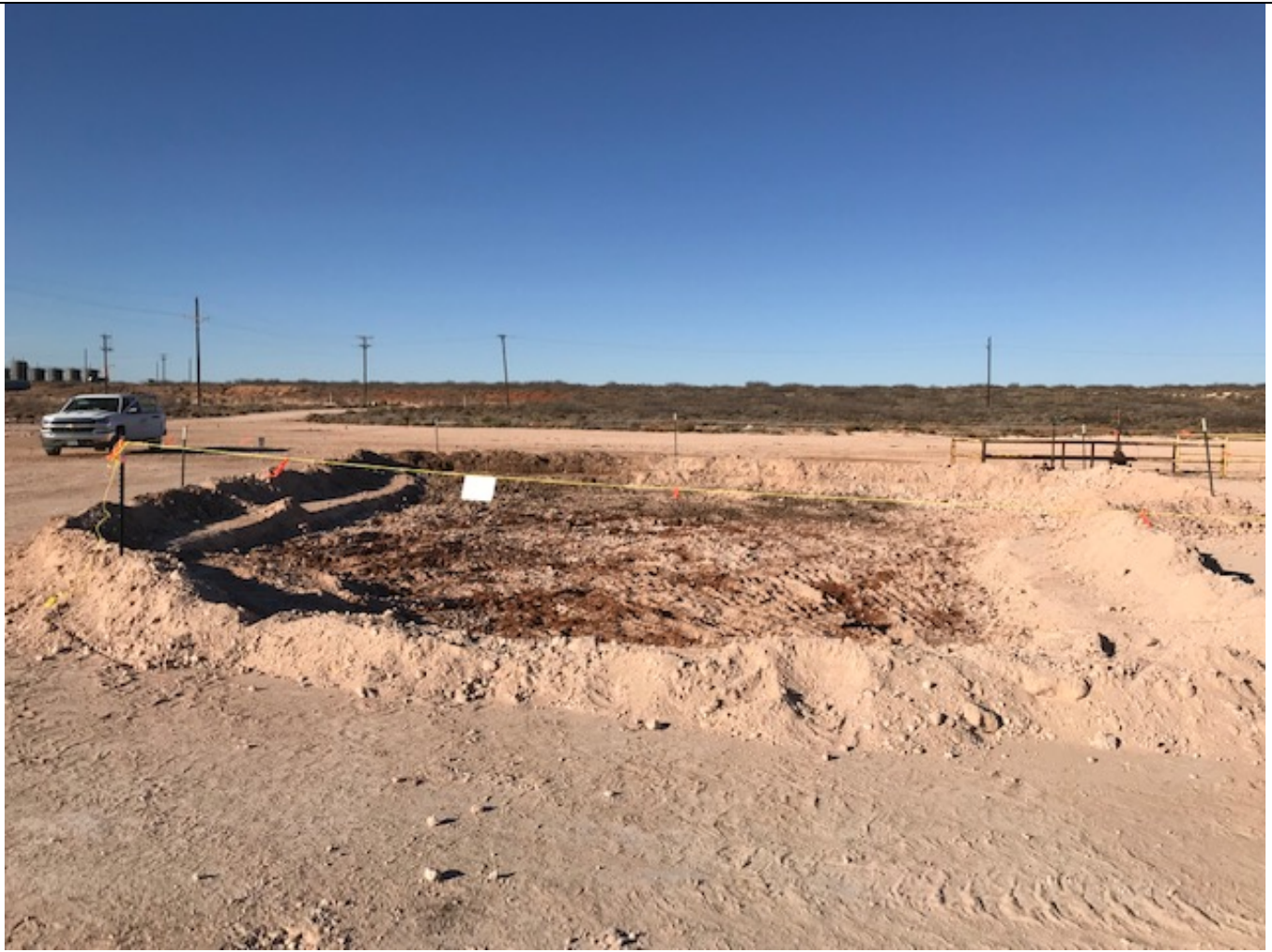
View facing north of the open excavation.
