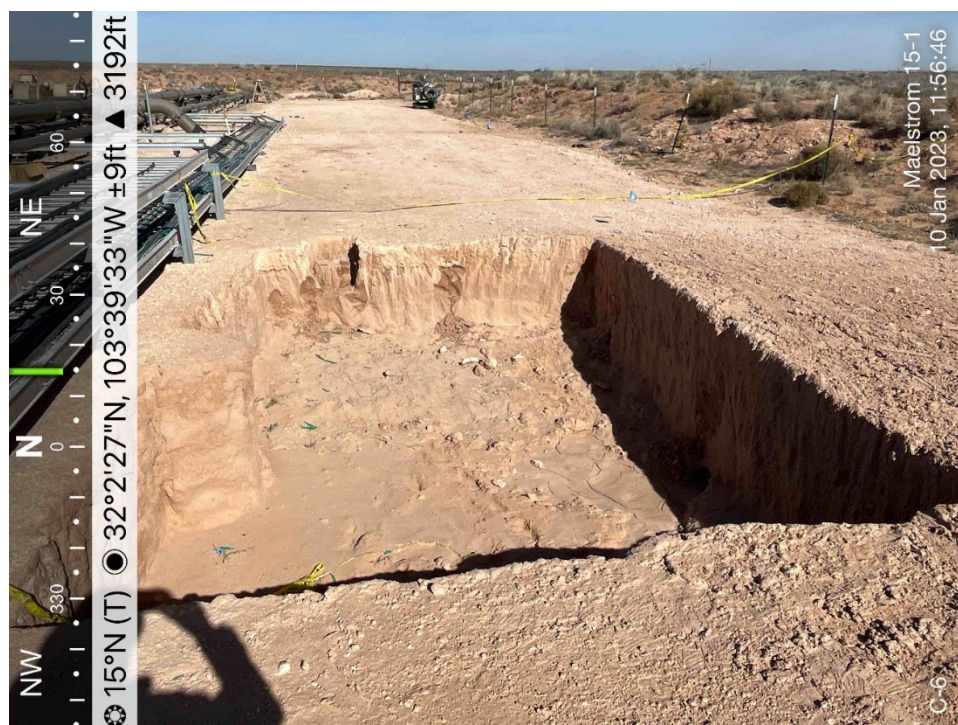
Excavated soil (nAPP2202549943), January 10, 2023
