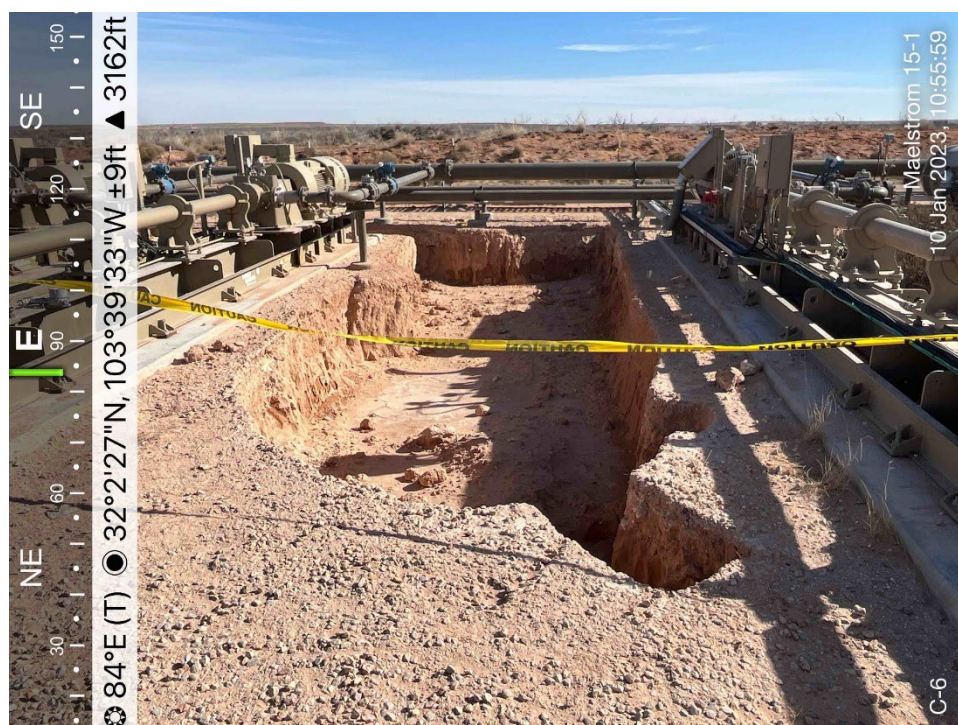
Excavated soil (nAPP2202549943), January 10, 2023
