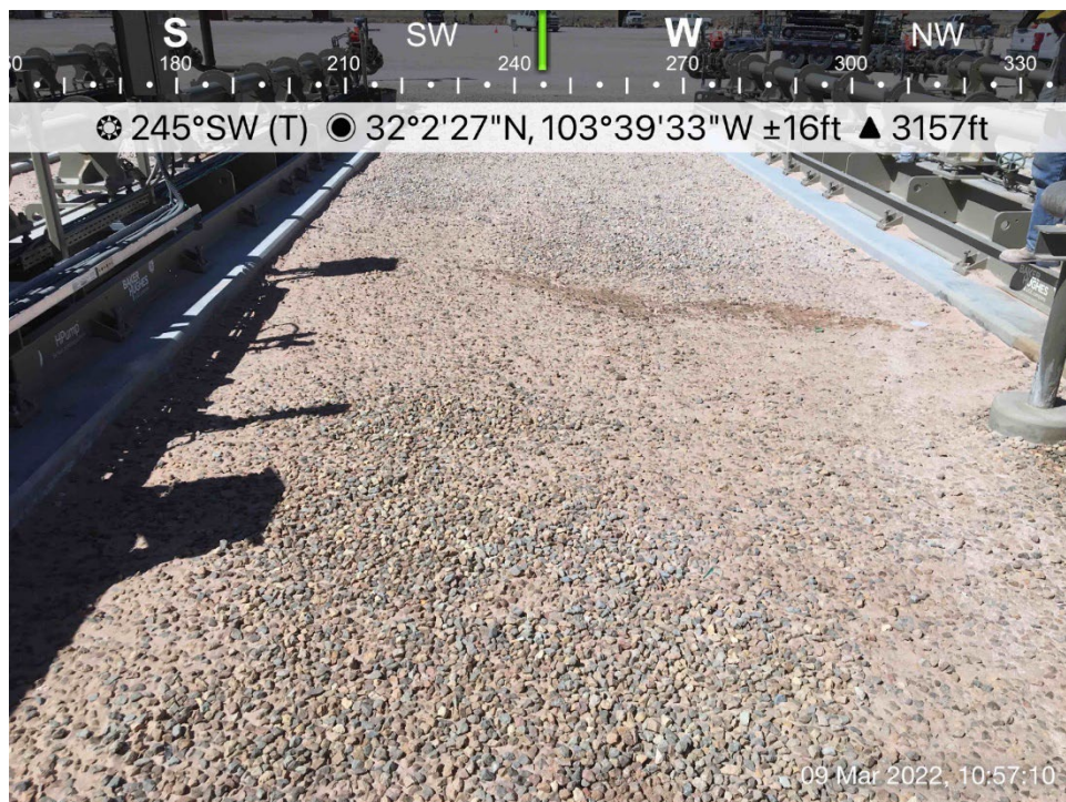
Impacted area (nAPP2202549943) viewing southwest, March 9, 2022
