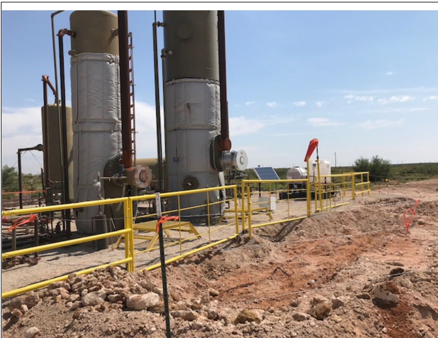
East facing view of the open excavation on the south side of the process equipment.
