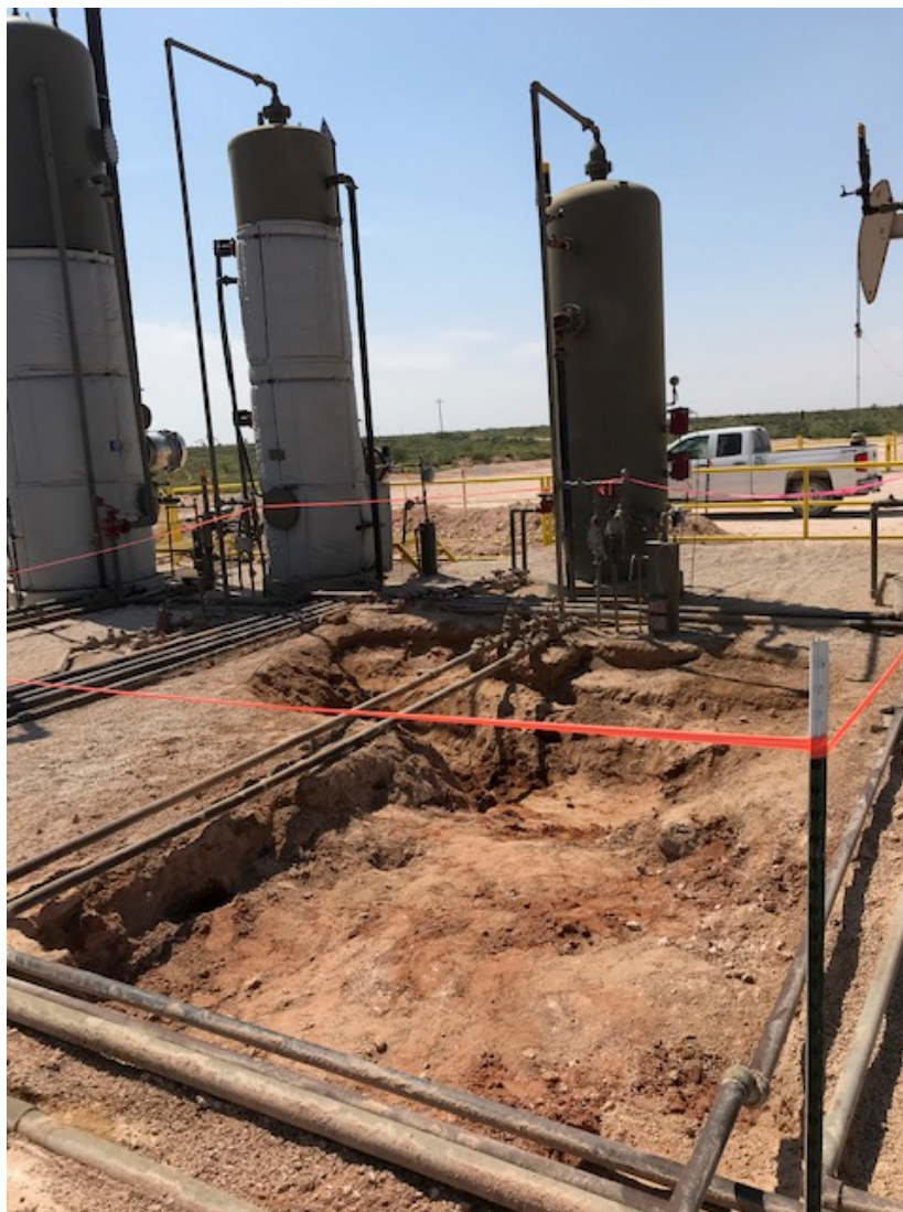
South facing view of the open excavation on the north side of the process equipment.
