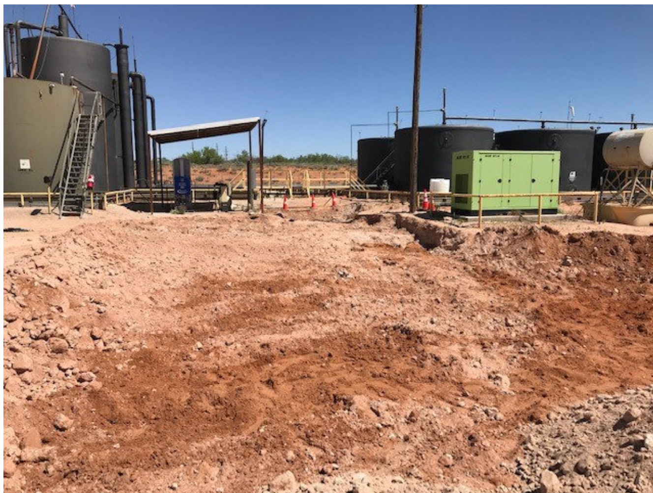
Northeastern view from northern edge of excavated area during excavation activities.
