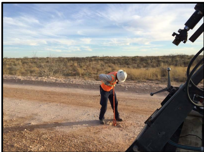
Collection of soil samples along Monsanto Road utilizing a hang auger.
