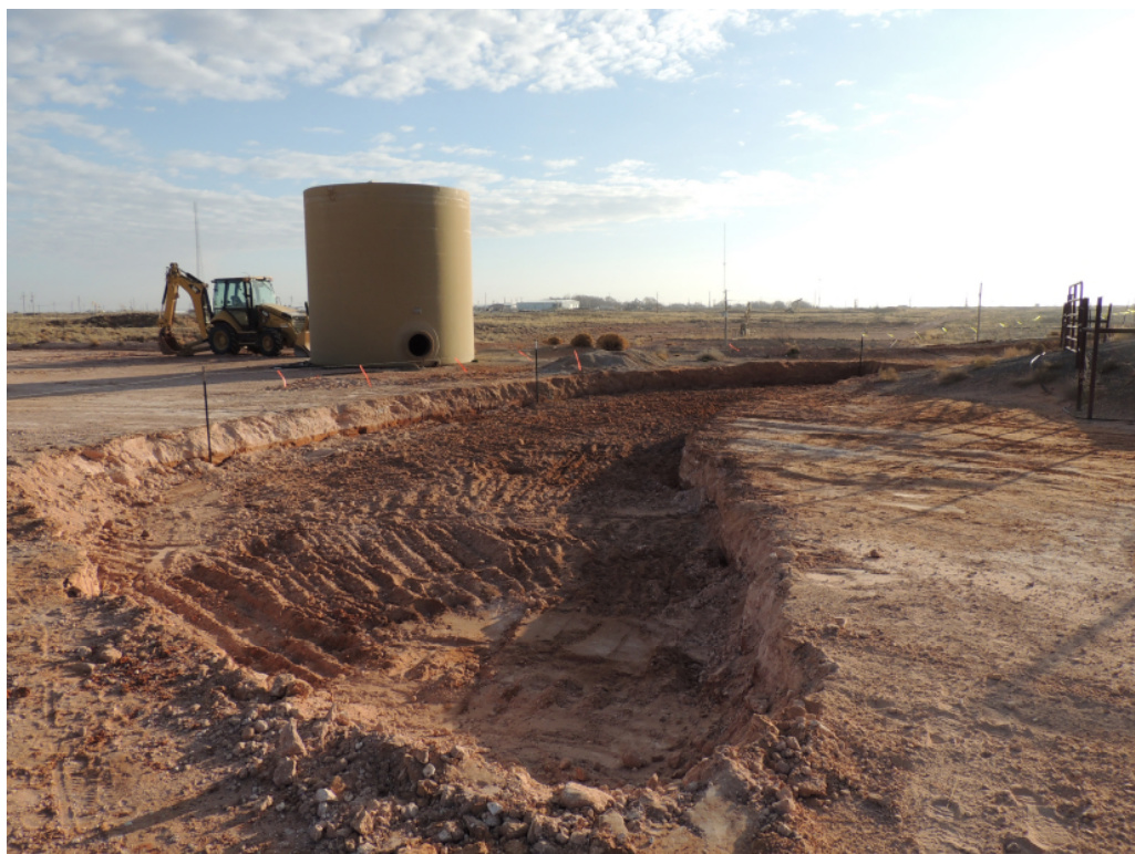
View East – Excavated Area of T-2
