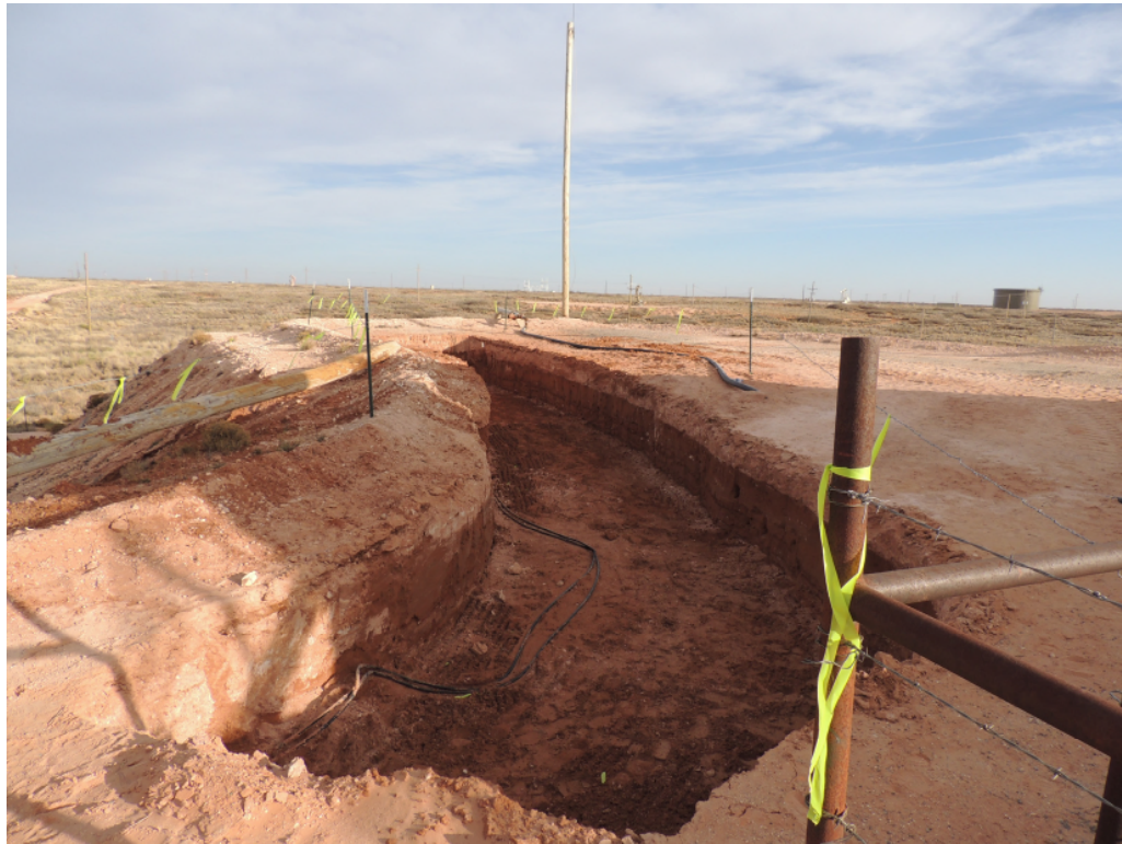
View East – Excavated Area of T-1
