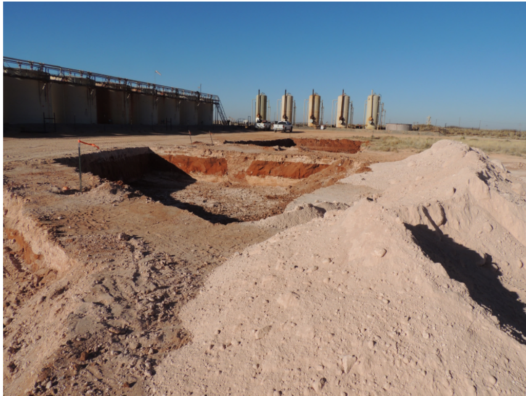
View West – Excavated Area of T-3
