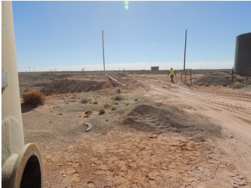
View East – Backfilled Area of T-1
