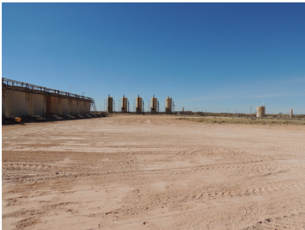
View West – Backfilled Areas of T-2, T-3, and T-4
