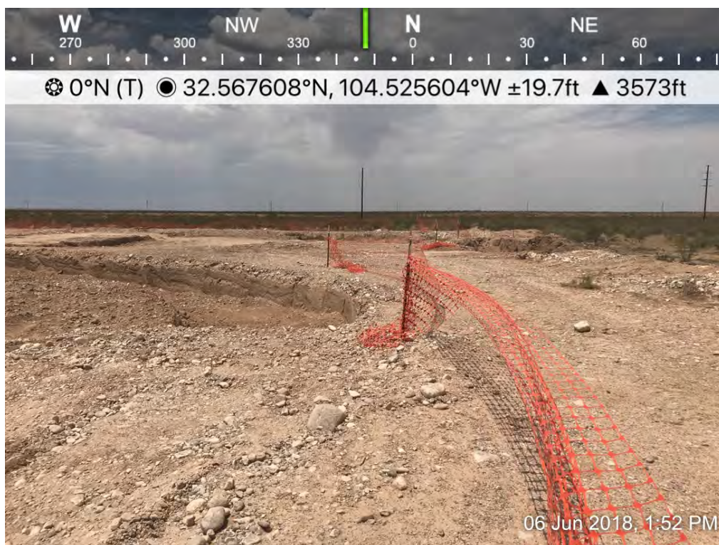
Osage 18 Fee B Com 0001H – Excavation
