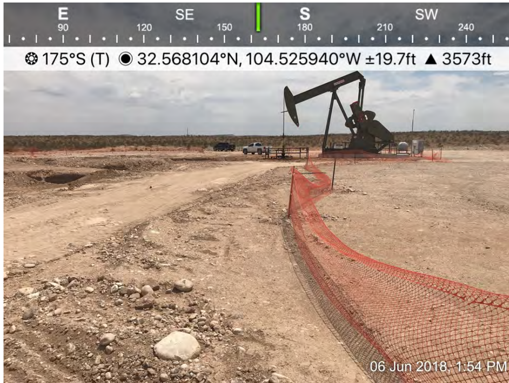
Osage 18 Fee B Com 0001H – Excavation
