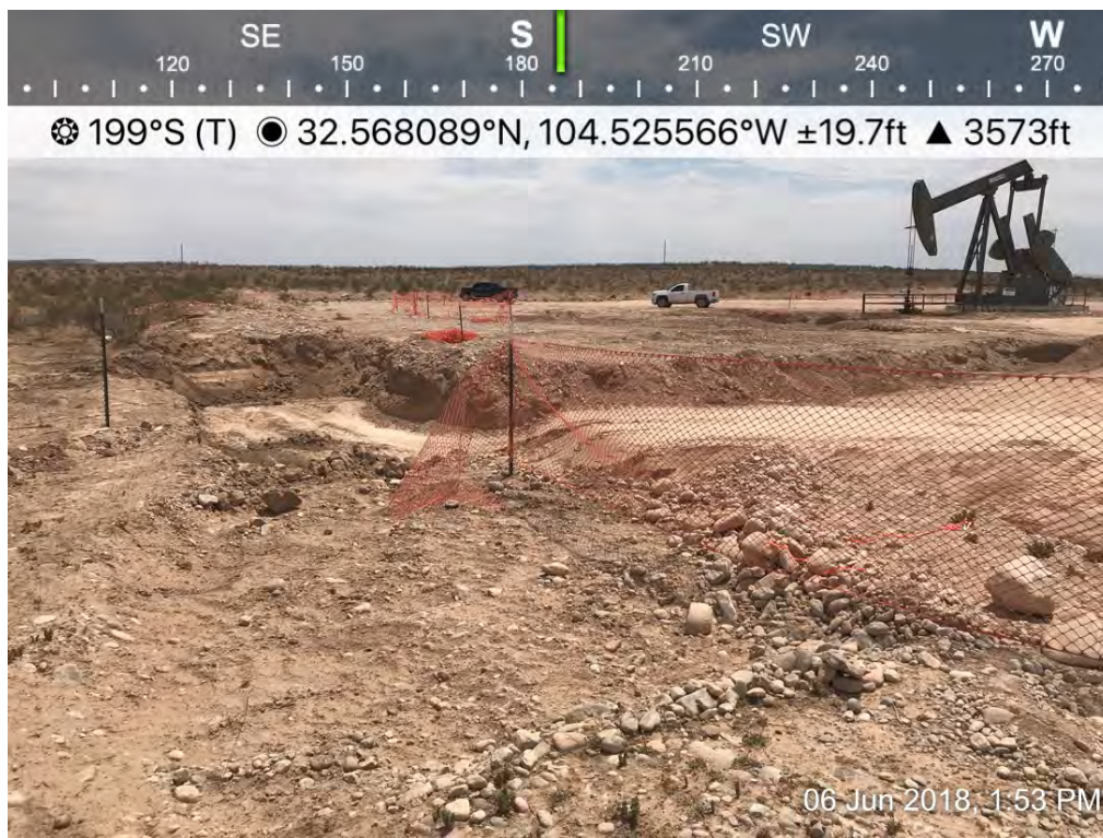
Osage 18 Fee B Com 0001H – Excavation
