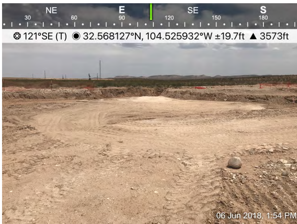
Osage 18 Fee B Com 0001H – Excavation
