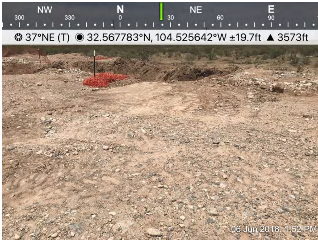
Osage 18 Fee B Com 0001H – Excavation
