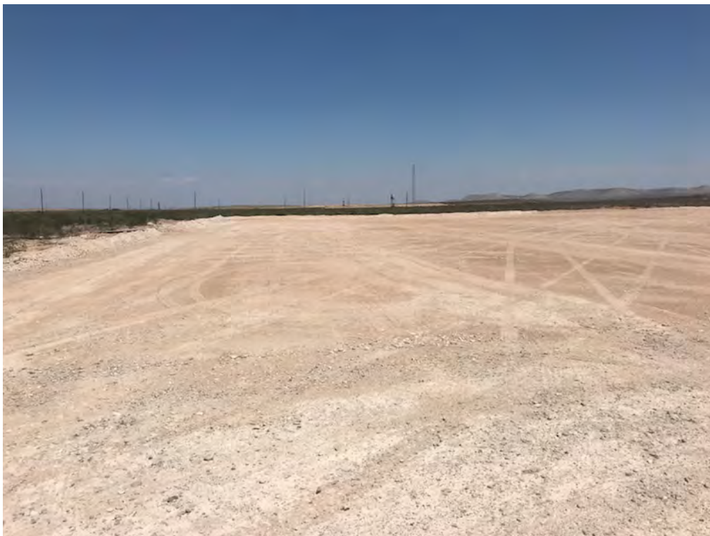
Osage 18 Fee B Com 0001H – Backfilled Excavation (Looking East)
