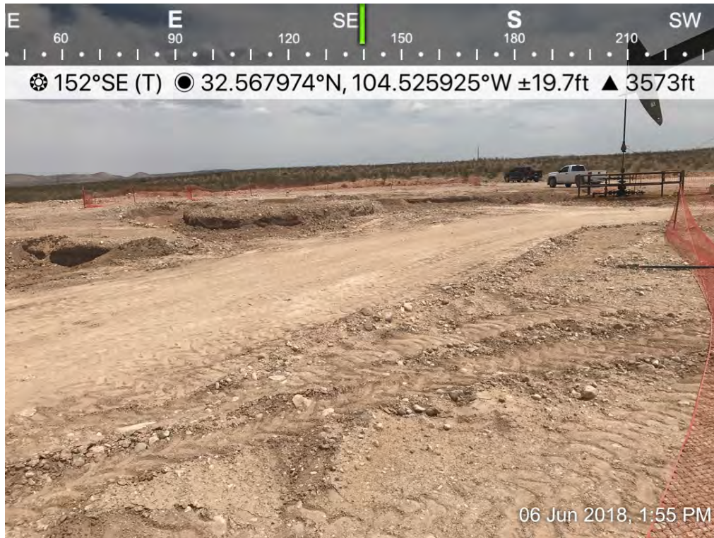
Osage 18 Fee B Com 0001H – Excavation
