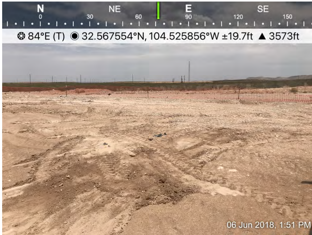
Osage 18 Fee B Com 0001H – Excavation
