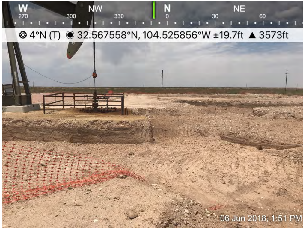
Osage 18 Fee B Com 0001H – Excavation
