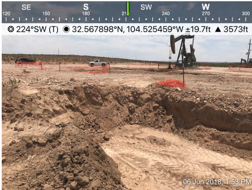
Osage 18 Fee B Com 0001H – Excavation
