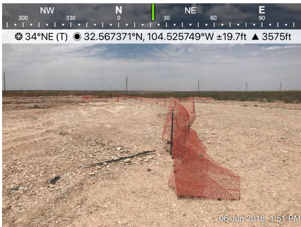
Osage 18 Fee B Com 0001H – Excavation
