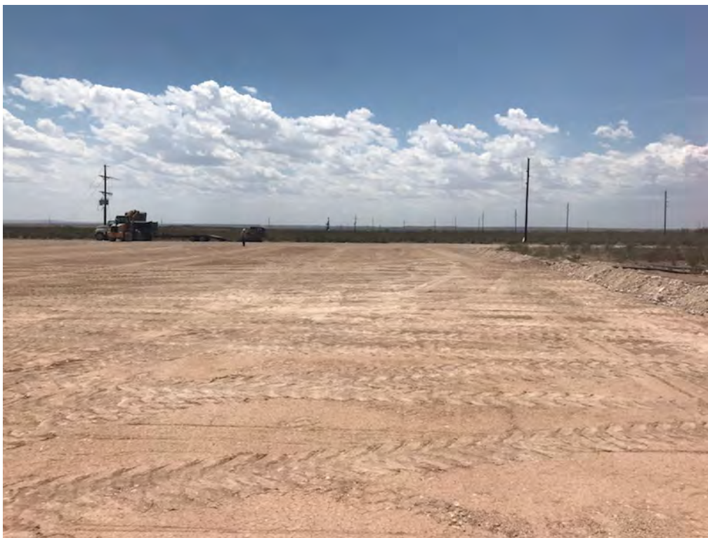
Osage 18 Fee B Com 0001H – Backfilled Excavation (Looking West)
