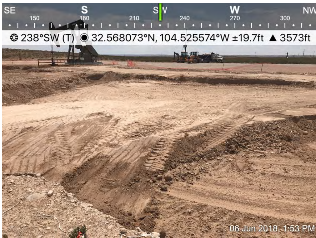
Osage 18 Fee B Com 0001H – Excavation
