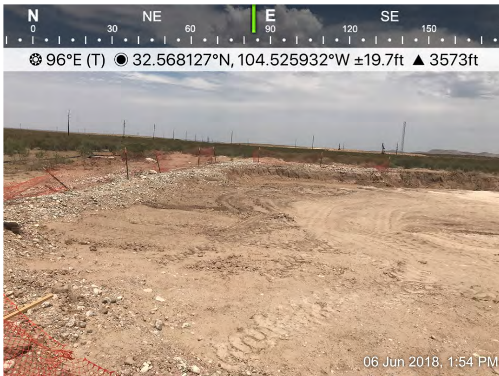
Osage 18 Fee B Com 0001H – Excavation
