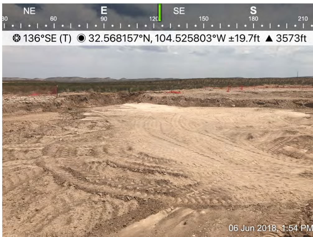
Osage 18 Fee B Com 0001H – Excavation
