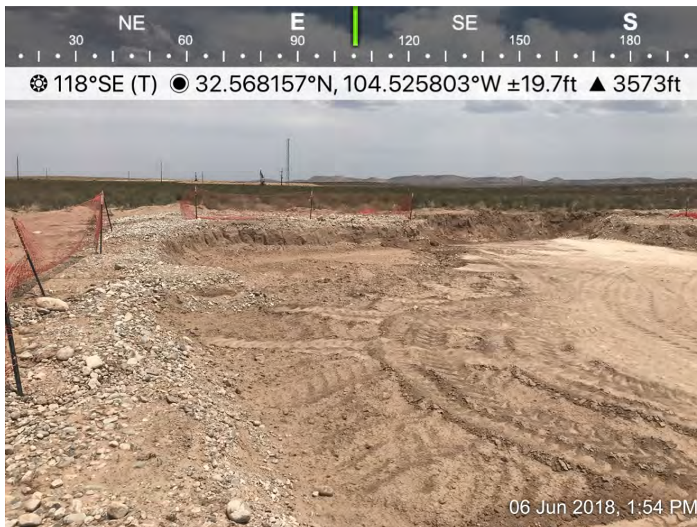
Osage 18 Fee B Com 0001H – Excavation
