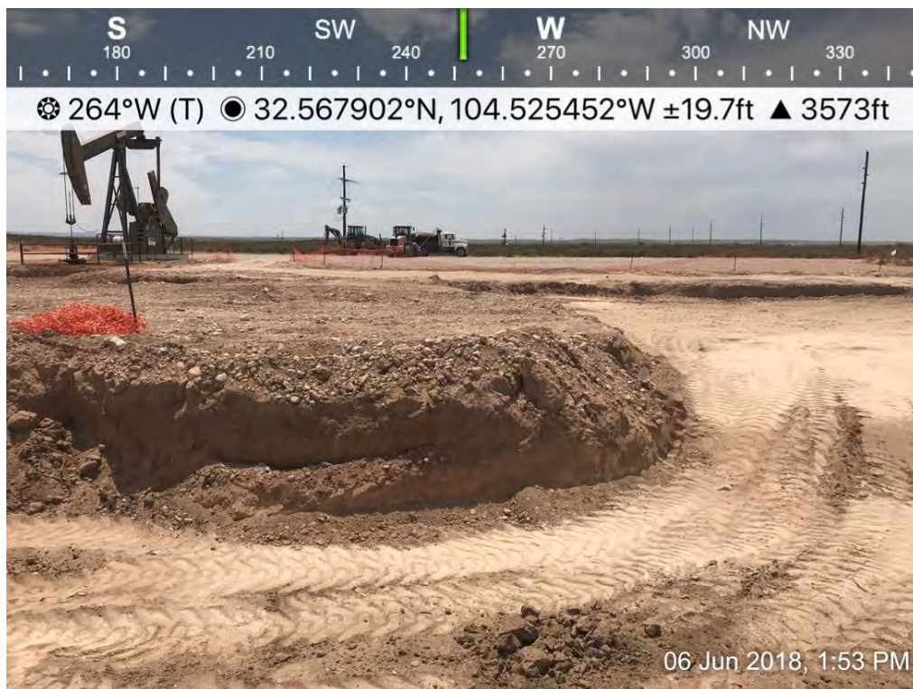
Osage 18 Fee B Com 0001H – Excavation
