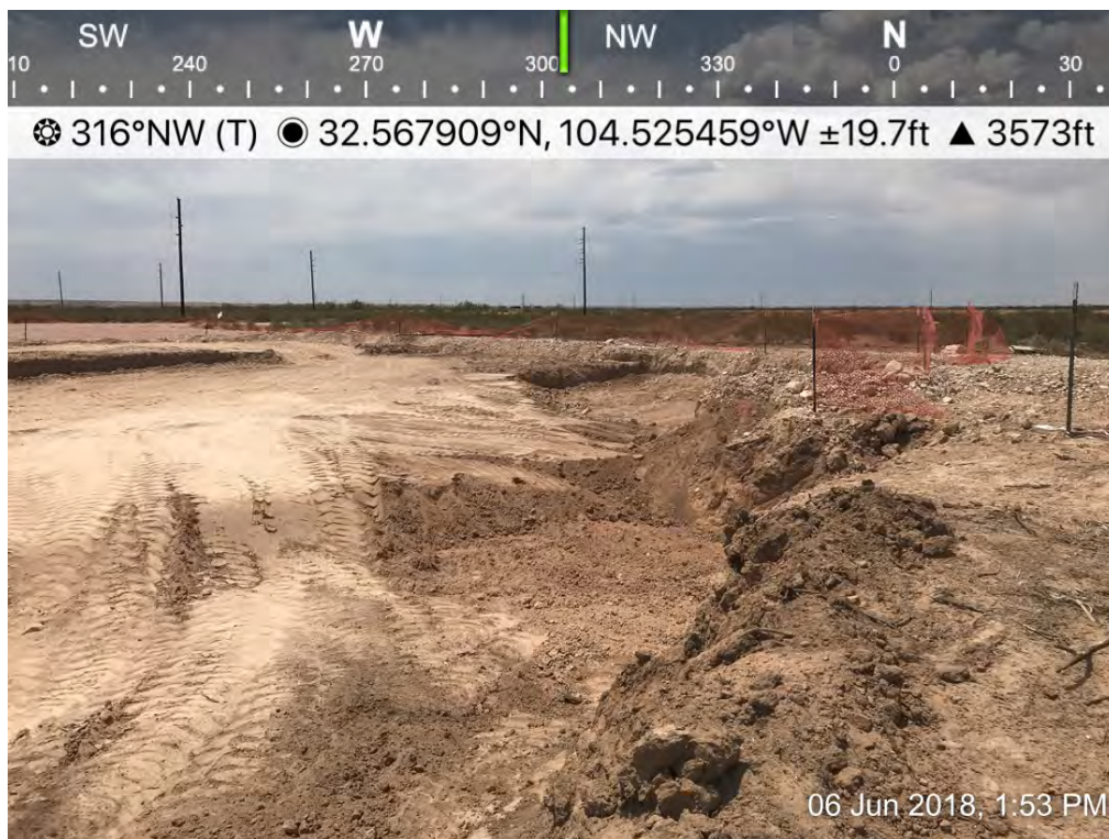
Osage 18 Fee B Com 0001H – Excavation
