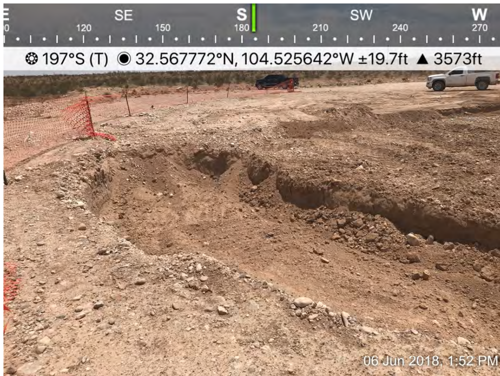
Osage 18 Fee B Com 0001H – Excavation
