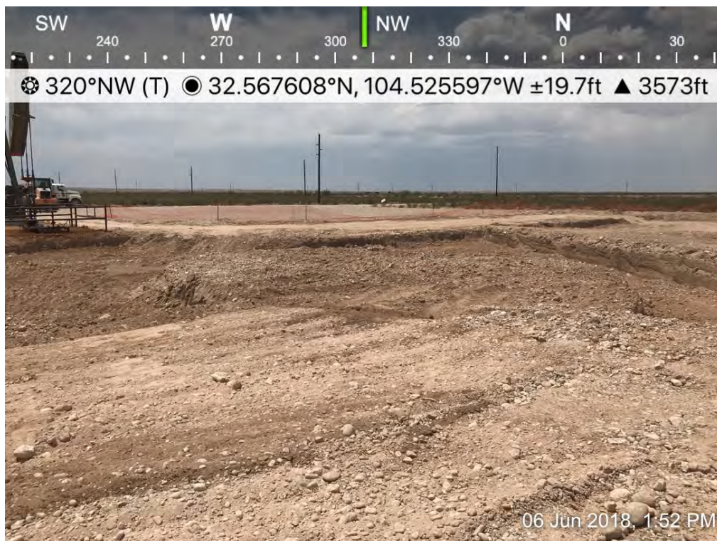
Osage 18 Fee B Com 0001H – Excavation
