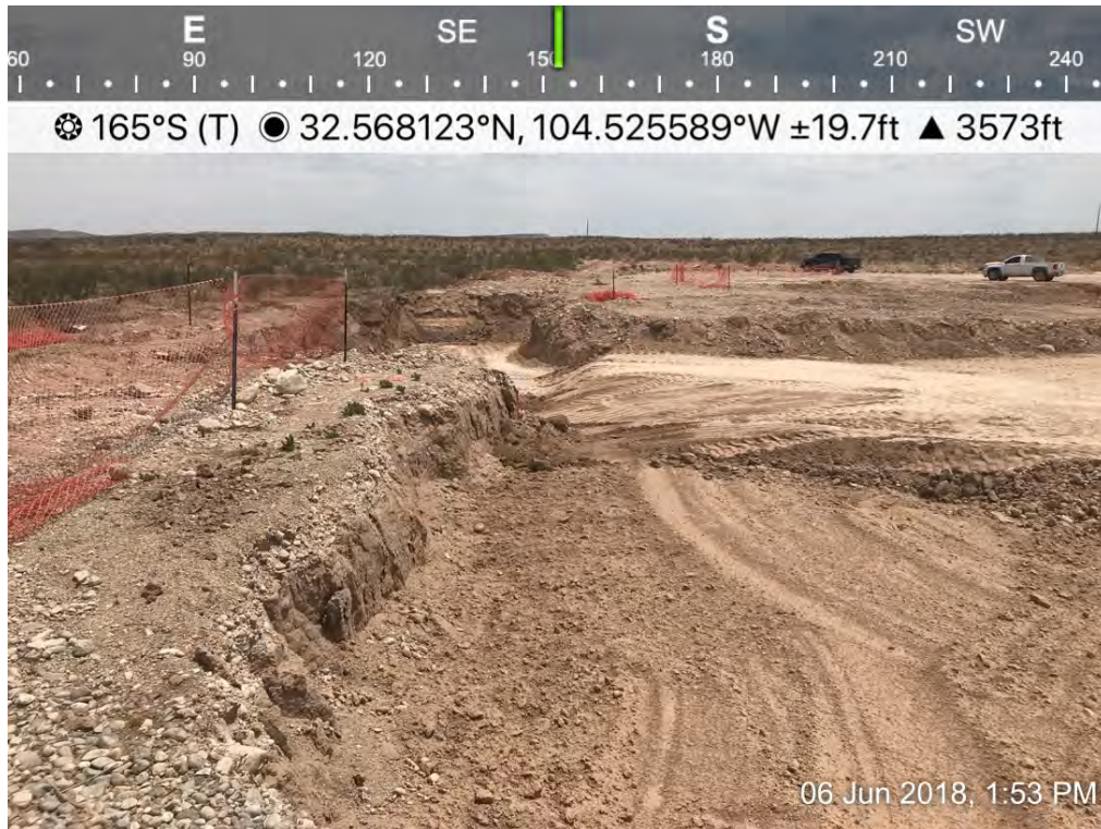
Osage 18 Fee B Com 0001H – Excavation
