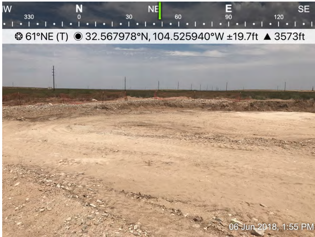
Osage 18 Fee B Com 0001H – Excavation
