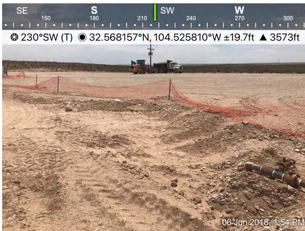
Osage 18 Fee B Com 0001H – Excavation
