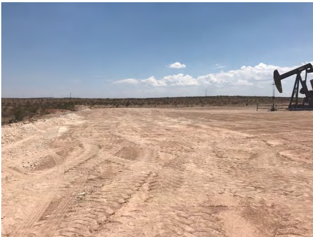
Osage 18 Fee B Com 0001H – Backfilled Excavation (Looking South)
