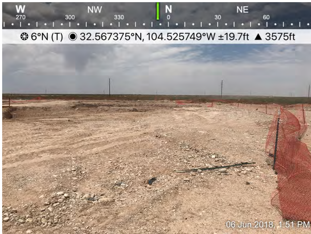
Osage 18 Fee B Com 0001H – Excavation
