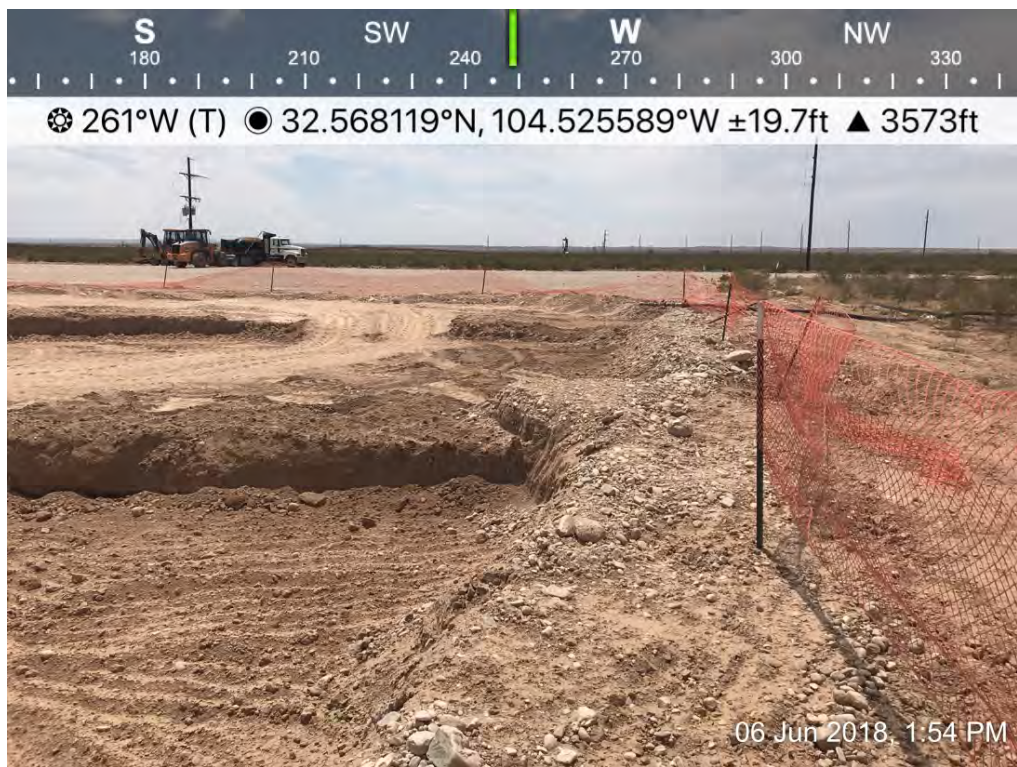
Osage 18 Fee B Com 0001H – Excavation
