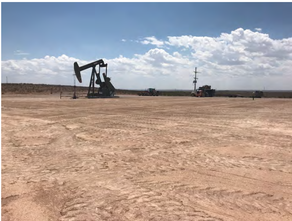
Osage 18 Fee B Com 0001H – Backfilled Excavation (Looking Southwest)
