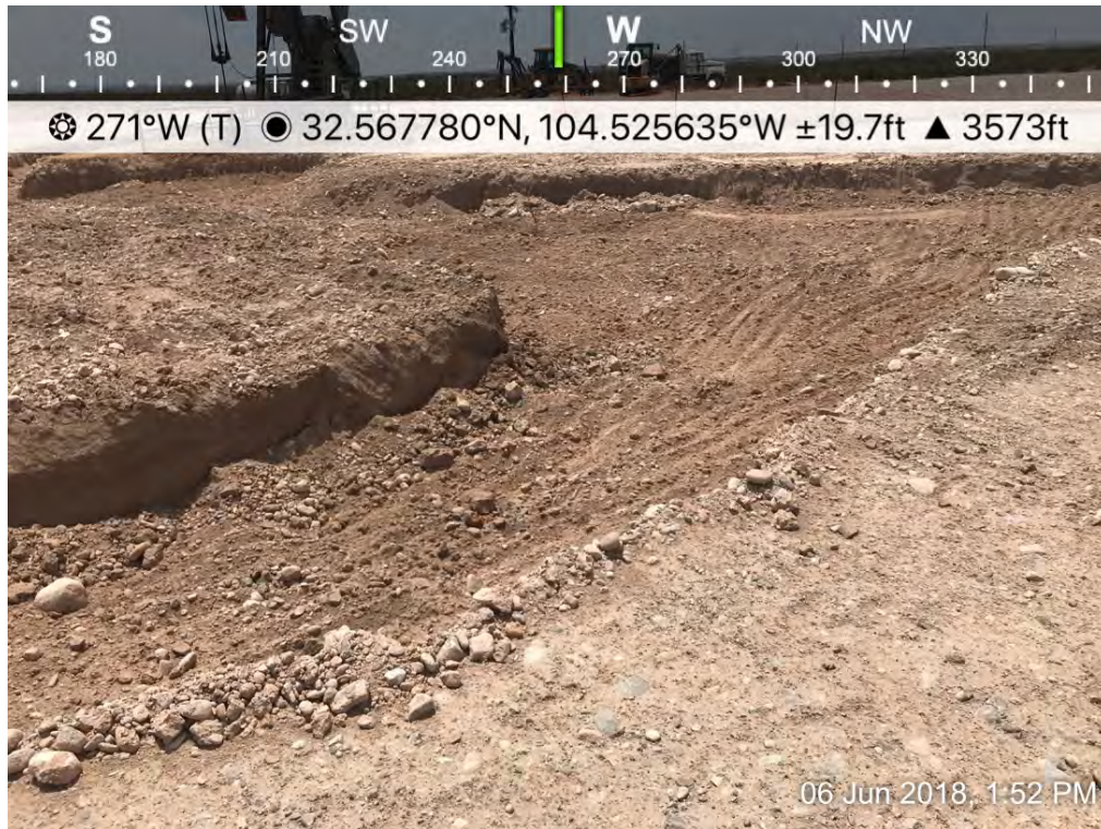
Osage 18 Fee B Com 0001H – Excavation
