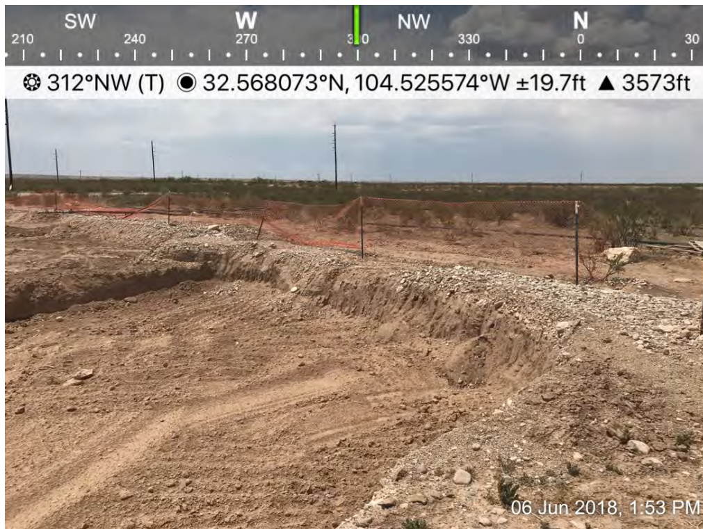
Osage 18 Fee B Com 0001H – Excavation
