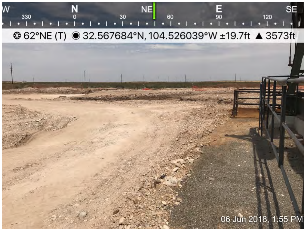
Osage 18 Fee B Com 0001H – Excavation
