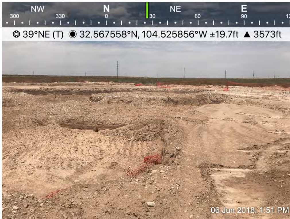
Osage 18 Fee B Com 0001H – Excavation
