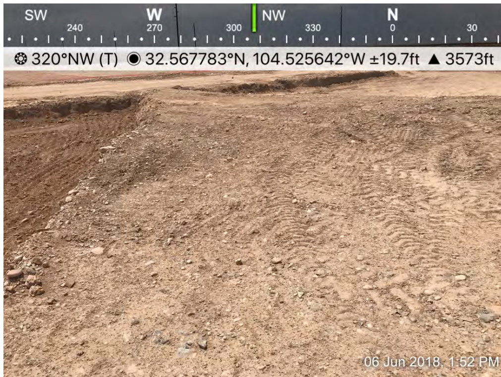
Osage 18 Fee B Com 0001H – Excavation
