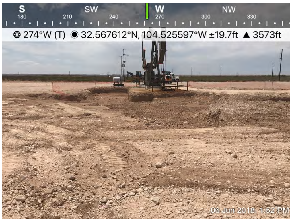
Osage 18 Fee B Com 0001H – Excavation
