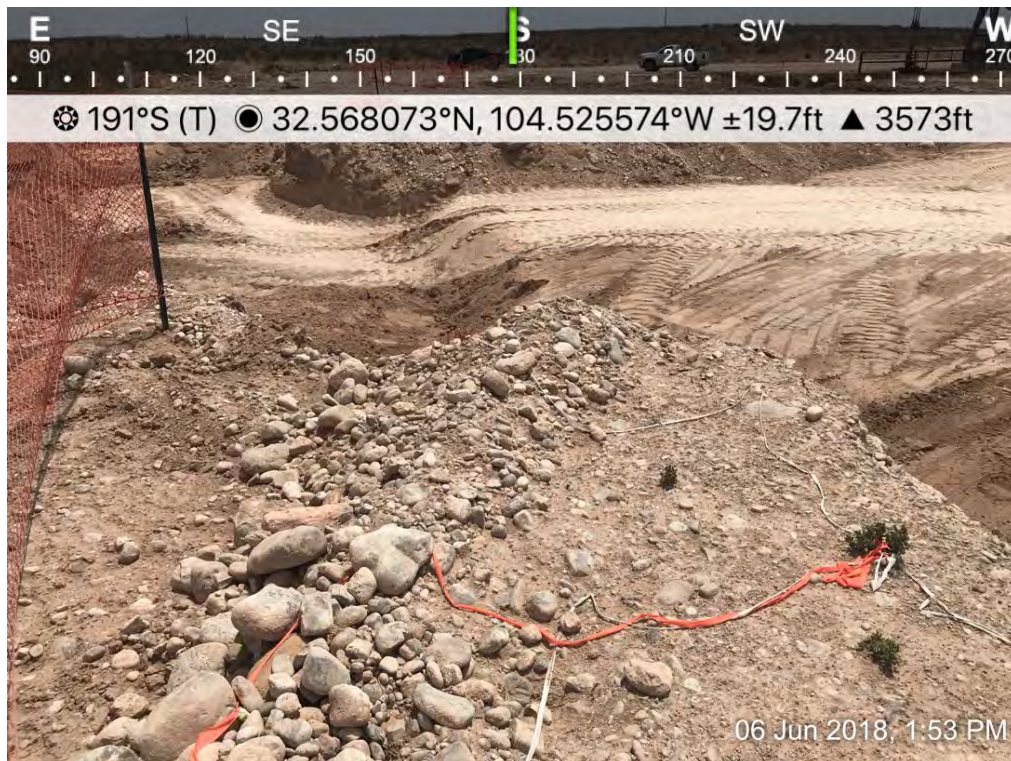
Osage 18 Fee B Com 0001H – Excavation
