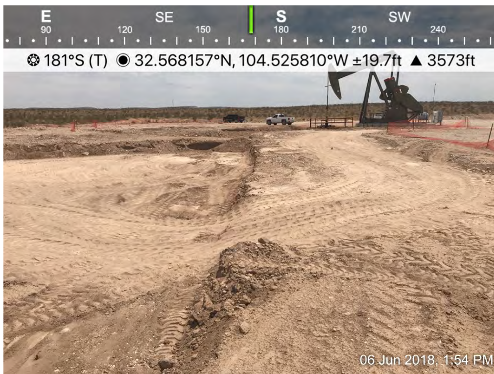
Osage 18 Fee B Com 0001H – Excavation
