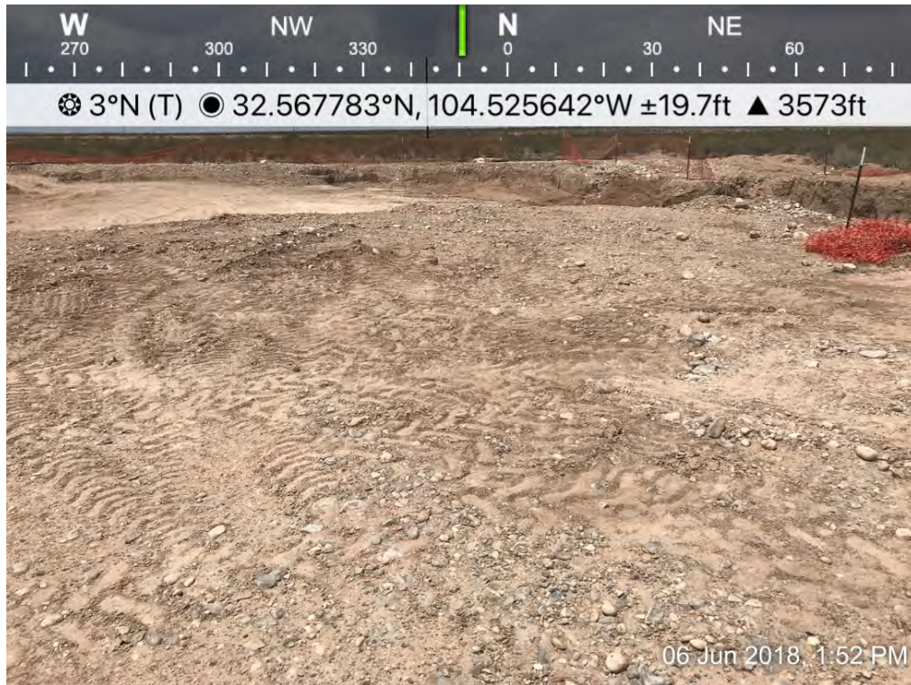
Osage 18 Fee B Com 0001H – Excavation
