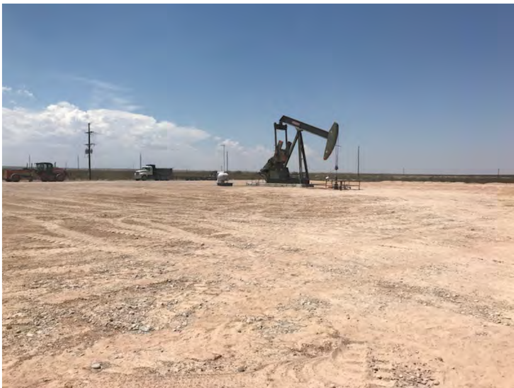
Osage 18 Fee B Com 0001H – Backfilled Excavation (Looking Northwest)
