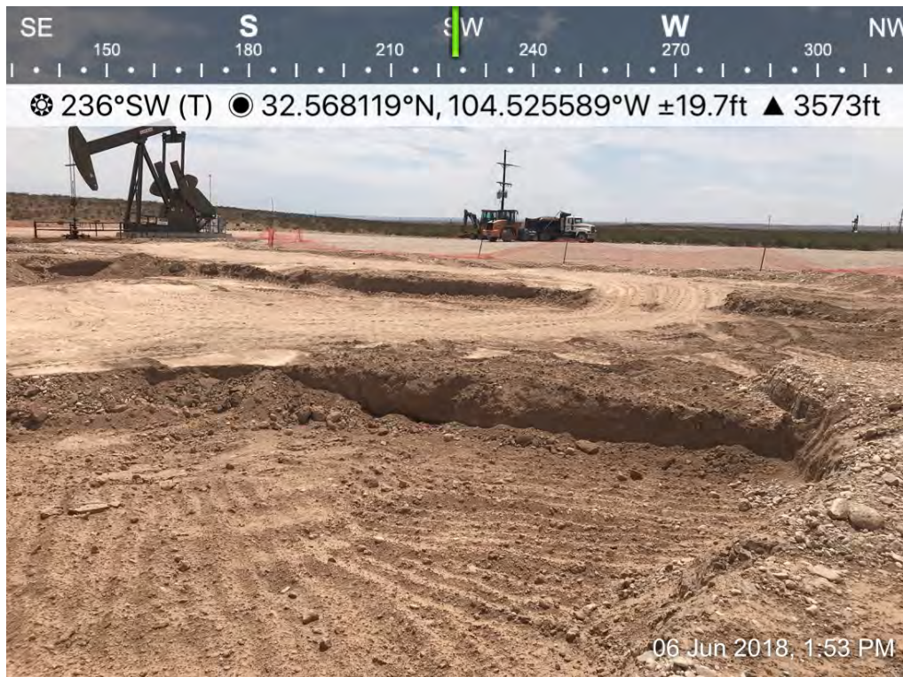
Osage 18 Fee B Com 0001H – Excavation
