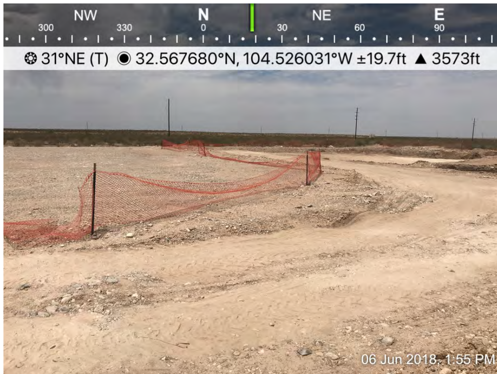
Osage 18 Fee B Com 0001H – Excavation
