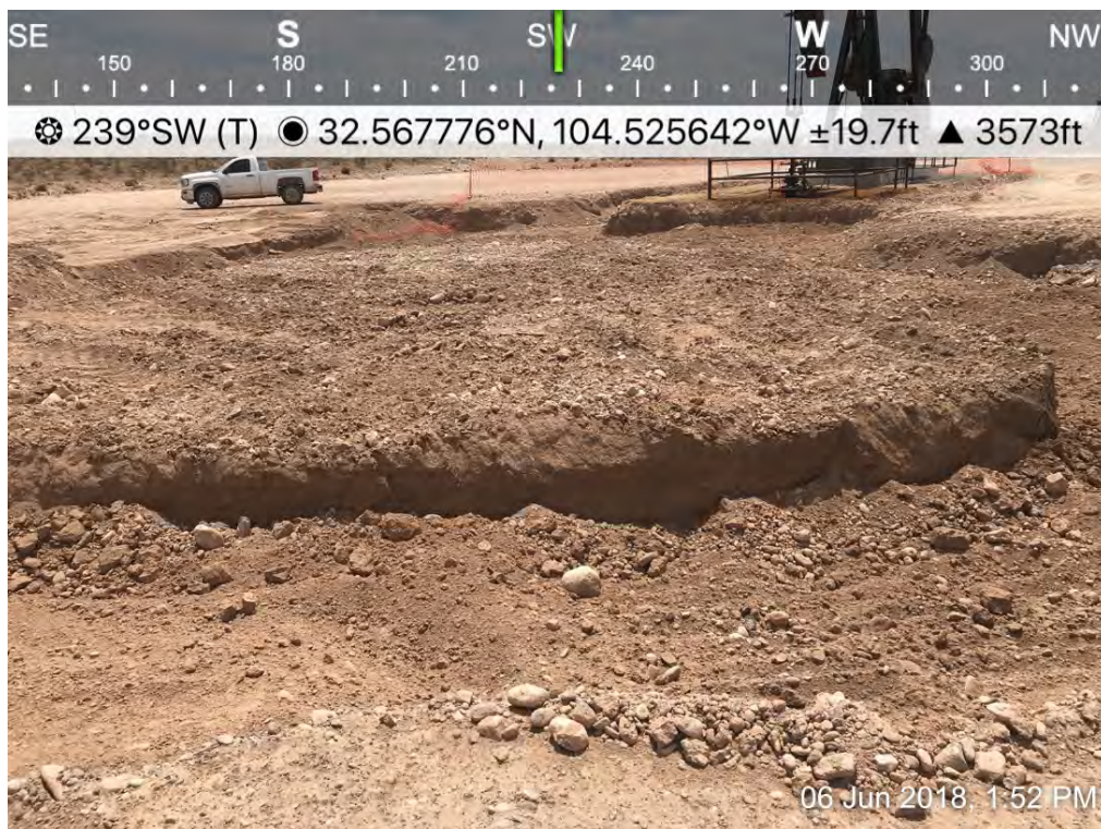
Osage 18 Fee B Com 0001H – Excavation
