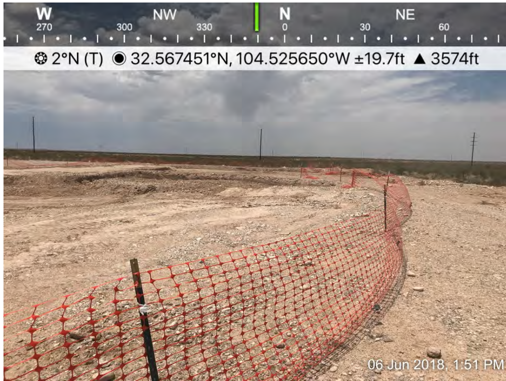
Osage 18 Fee B Com 0001H – Excavation
