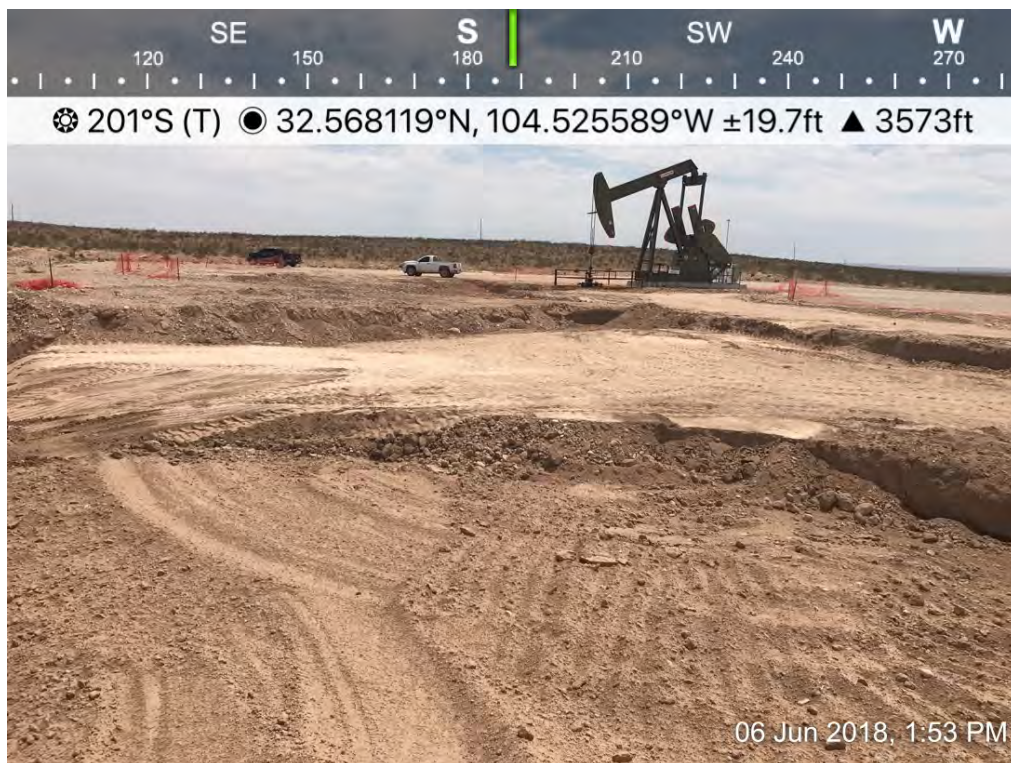
Osage 18 Fee B Com 0001H – Excavation
