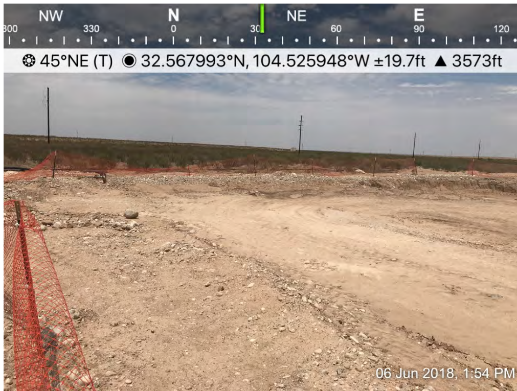
Osage 18 Fee B Com 0001H – Excavation
