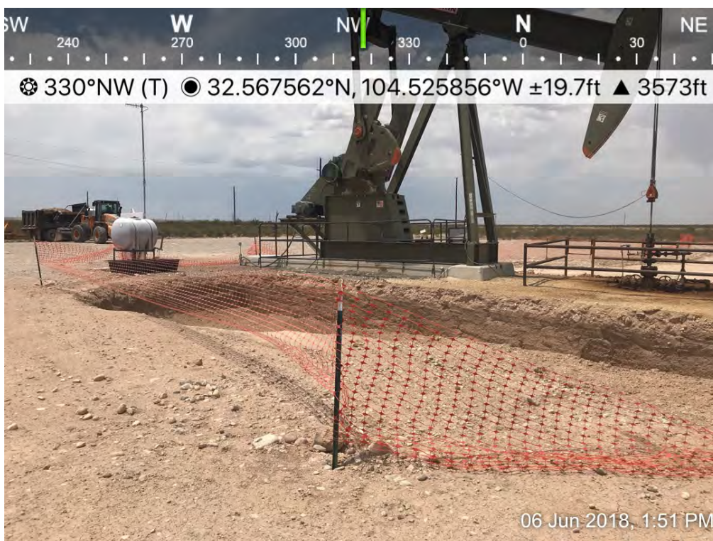
Osage 18 Fee B Com 0001H – Excavation
