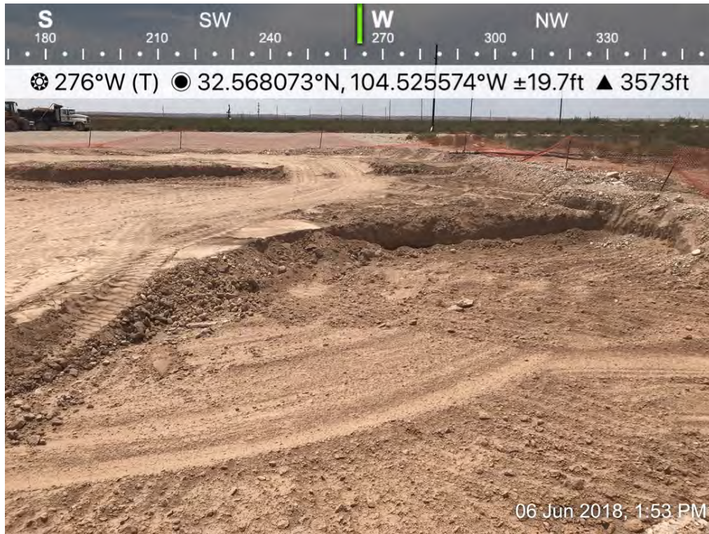
Osage 18 Fee B Com 0001H – Excavation
