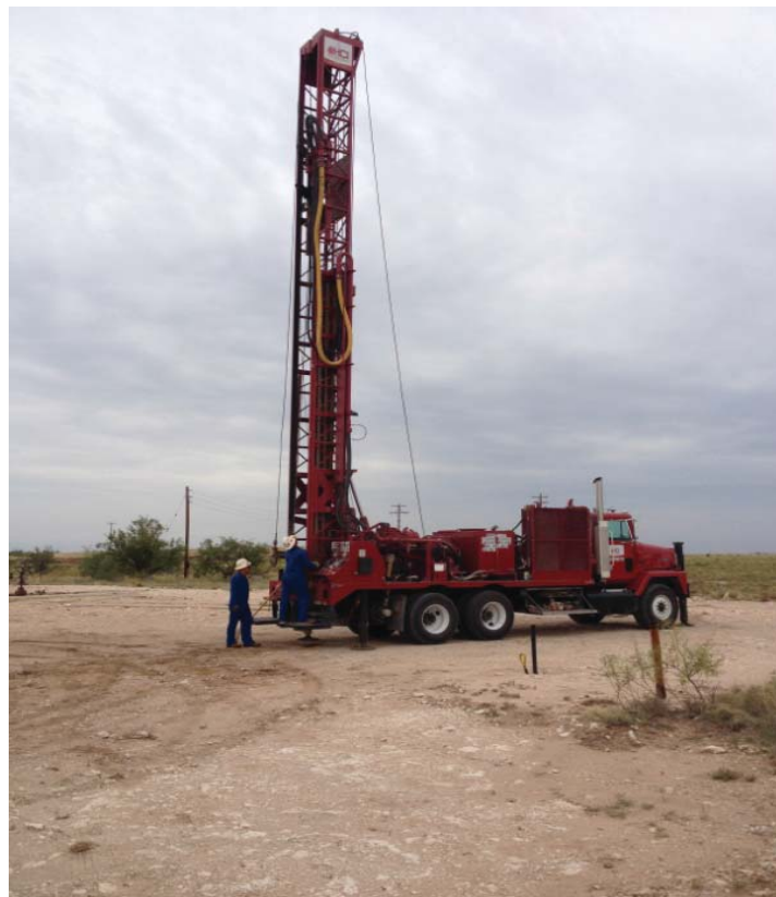
PHOTO 4: View of drilling activities facing north east
