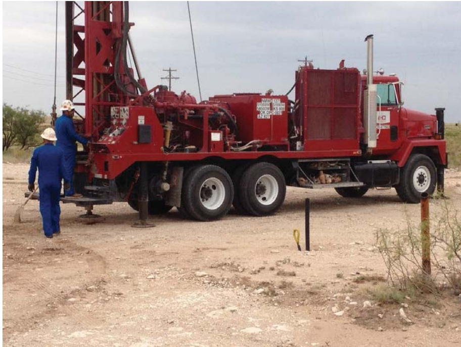
PHOTO 3: View of drilling activities facing south east
