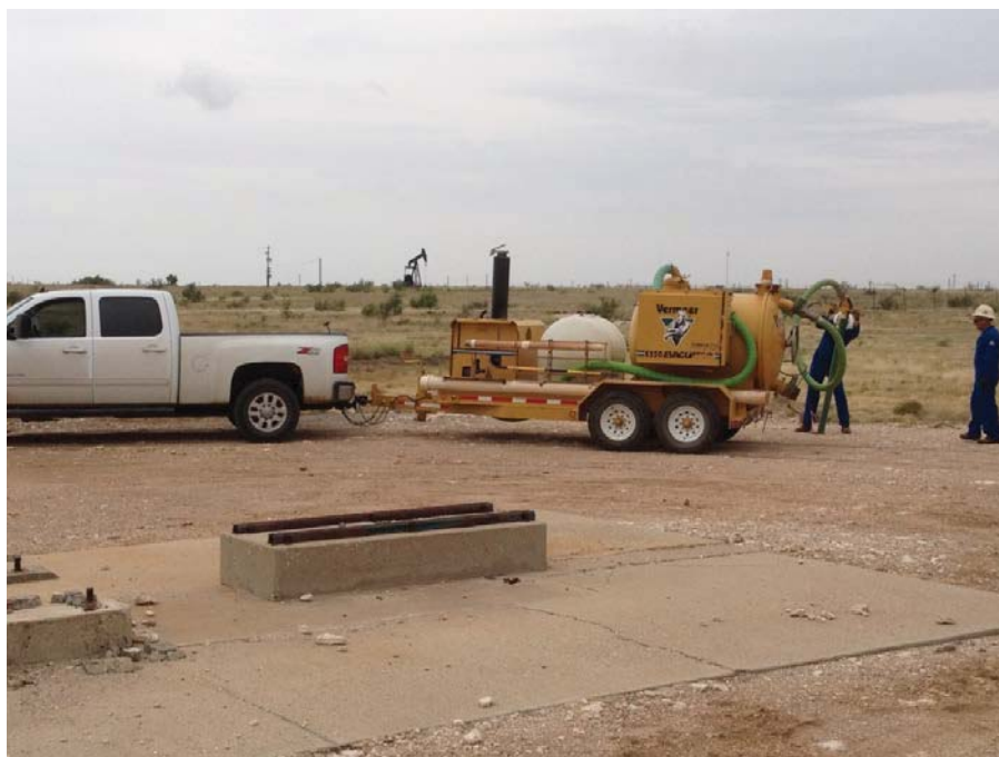
PHOTO 2: View of Air-Knife borehole clearance activities facing north east
