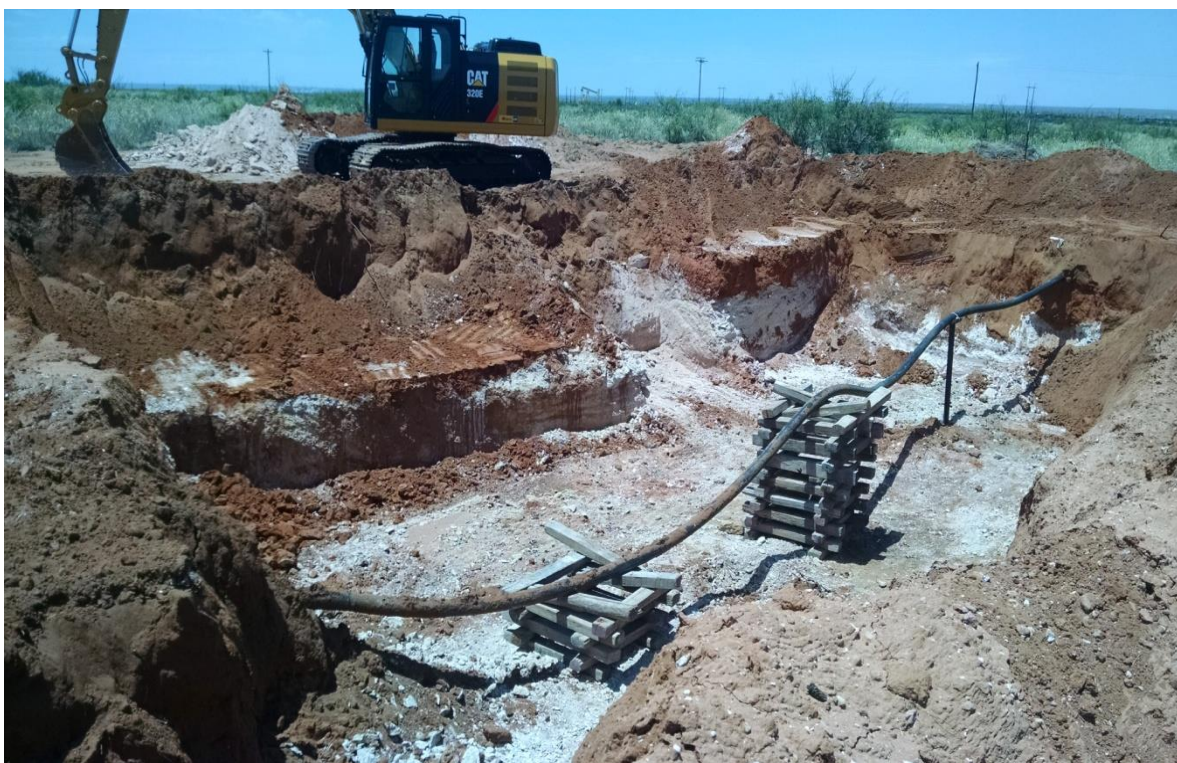
Palladium 7-1 4-Inch Poly – Excavation (Looking North)
