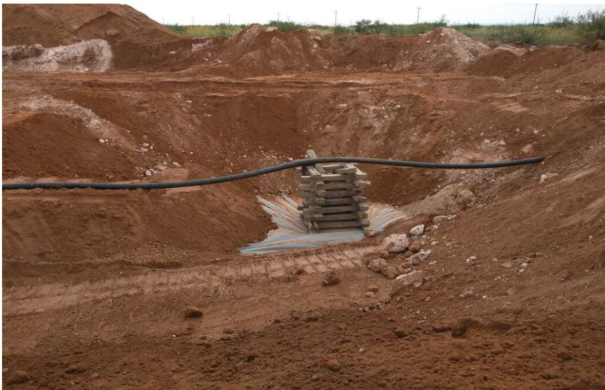
Palladium 7-1 4-Inch Poly - Backfilling (Looking West)
