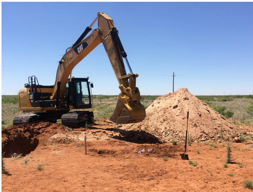
Palladium 7-1 4-Inch Poly – Advancement of Delineation Trench TT-1
