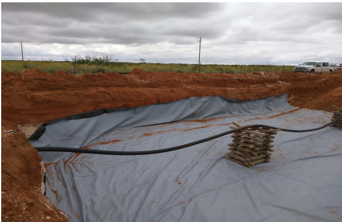
Palladium 7-1 4-Inch Poly – Liner Installation (Looking South-Southeast)
