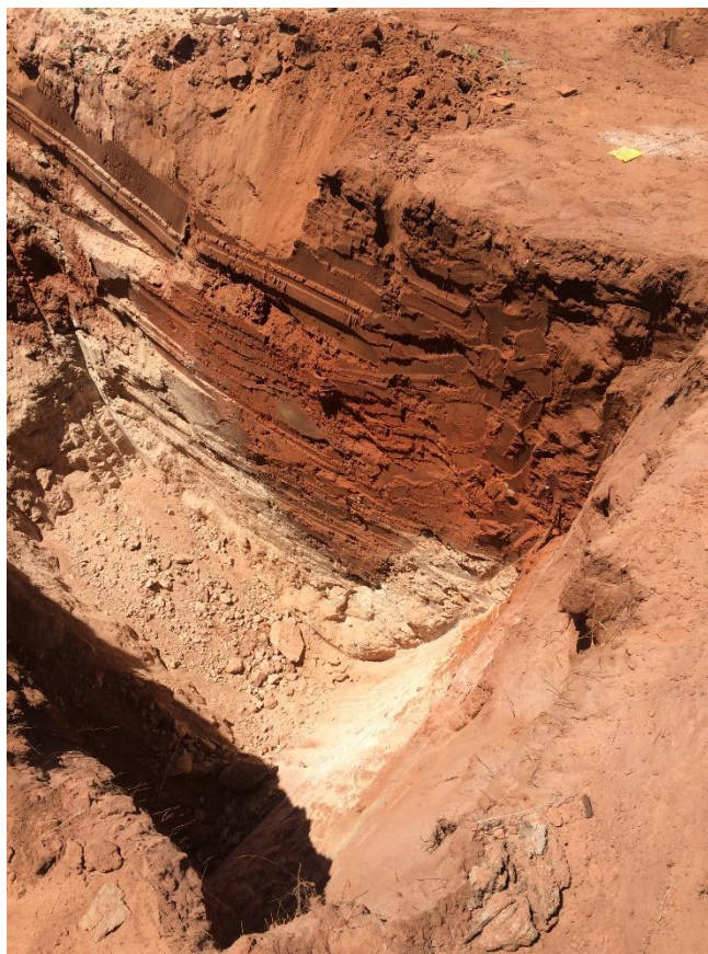
Palladium 7-1 4-Inch Poly – Delineation Trench TT-1 (Staining Visible on Wall of Trench)
