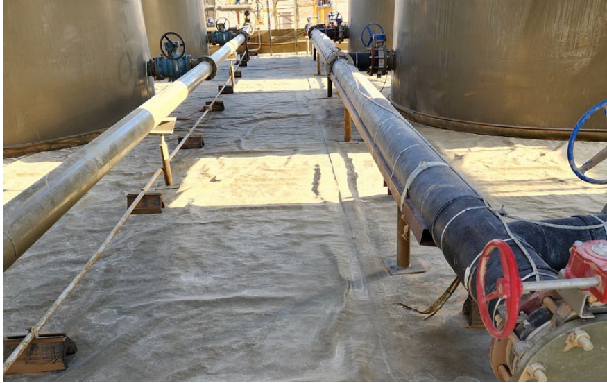
Figure 7: View of liner integrity from the third tank south from the north containment wall; south of the area of interest. No repairs were required north of this point. Photo is viewing north. Date Taken: 2023-04-05. Corrected GPS: 32.164844, 103.2878042. Geotagged GPS: 32.1650055, -103.2878978.
