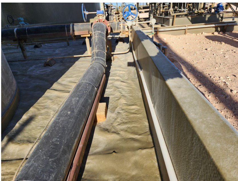
Figure 5: View of liner integrity between the tank that overflowed and the northern containment wall; where the on-site release was adjacent too. No repairs were required in this area of interest. Photo is viewing west. Date Taken: 2023-04-05. GPS: 32.1649385, -103.2878828.
