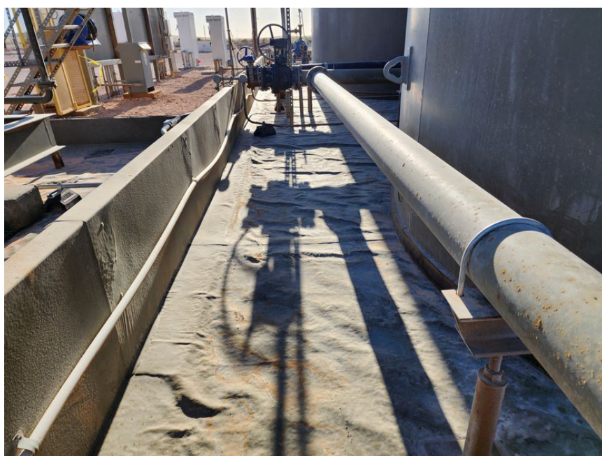
Figure 6: View of liner integrity between the tank that overflowed and the northern containment wall; at the area of interest. No repairs were required. Photo is viewing east. Date Taken: 2023-04-05. GPS: 32.1650055, -103.2878978.
