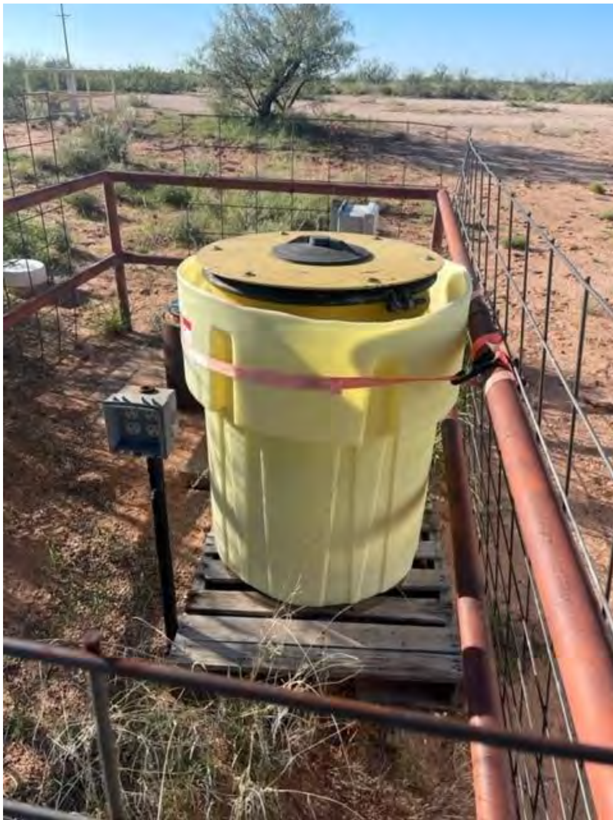
Jal #4 Gas Plant, Jal, New Mexico - drum in open overpack with Ventilated Barrel Cover – evaporates groundwater sampling IDW purgewater “24-7”; HMI will replace existing (rusting drum) with a new drum in 1Q23, due to rust developing where drum body connects to drum bottom, caused by retained rainwater in base of the overpack; the new drum will be elevated off the base of overpack minimize future rusting
