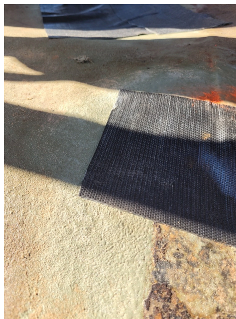
Photograph: 4 Date: 11/12/2022 Description: Photo of patched liner
