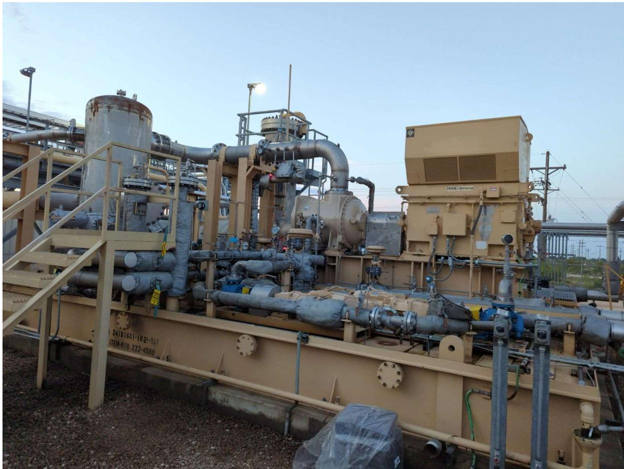
The 4500-compressor shut down on high discharge pressure. We had just gotten our inlet vessel pressures down at the battery, and then 32EC satellite pressured up to 360 psi and caused the compressor to go down. Sending all gas to the emergency flare.
