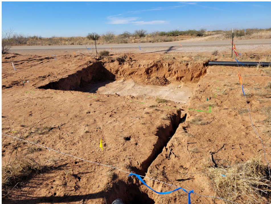
View of northern excavation facing southwest.
