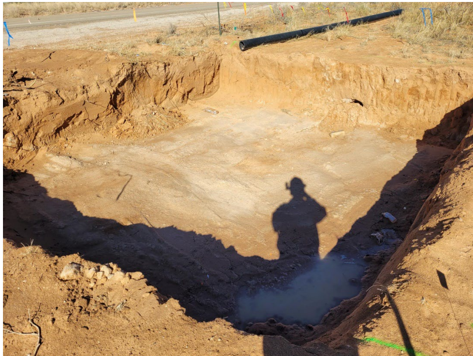
View of northern excavation facing northeast
