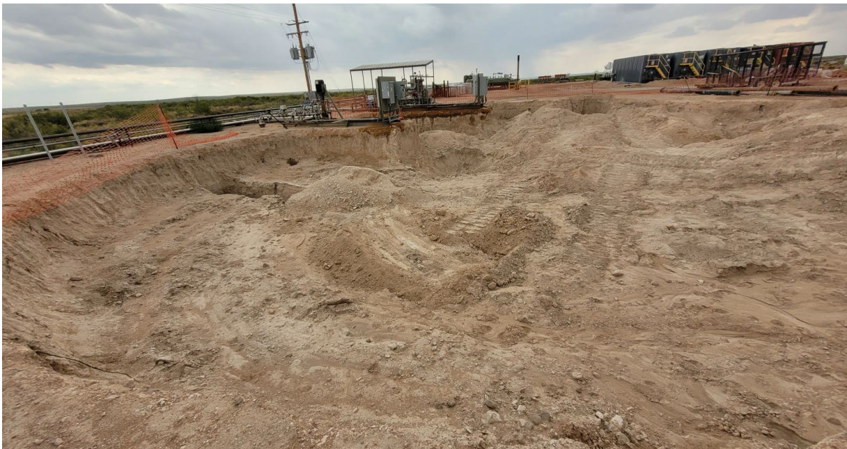
Photo 2 View to the south at the remedial excavation.
