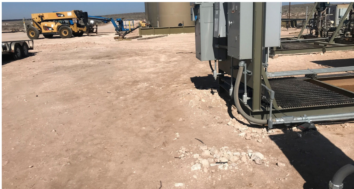
Photo 5 View to the north at the backfilled remedial excavation.
