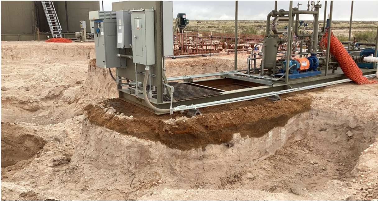
Photo 3 View of the LACT Units following remedial excavation activities.
