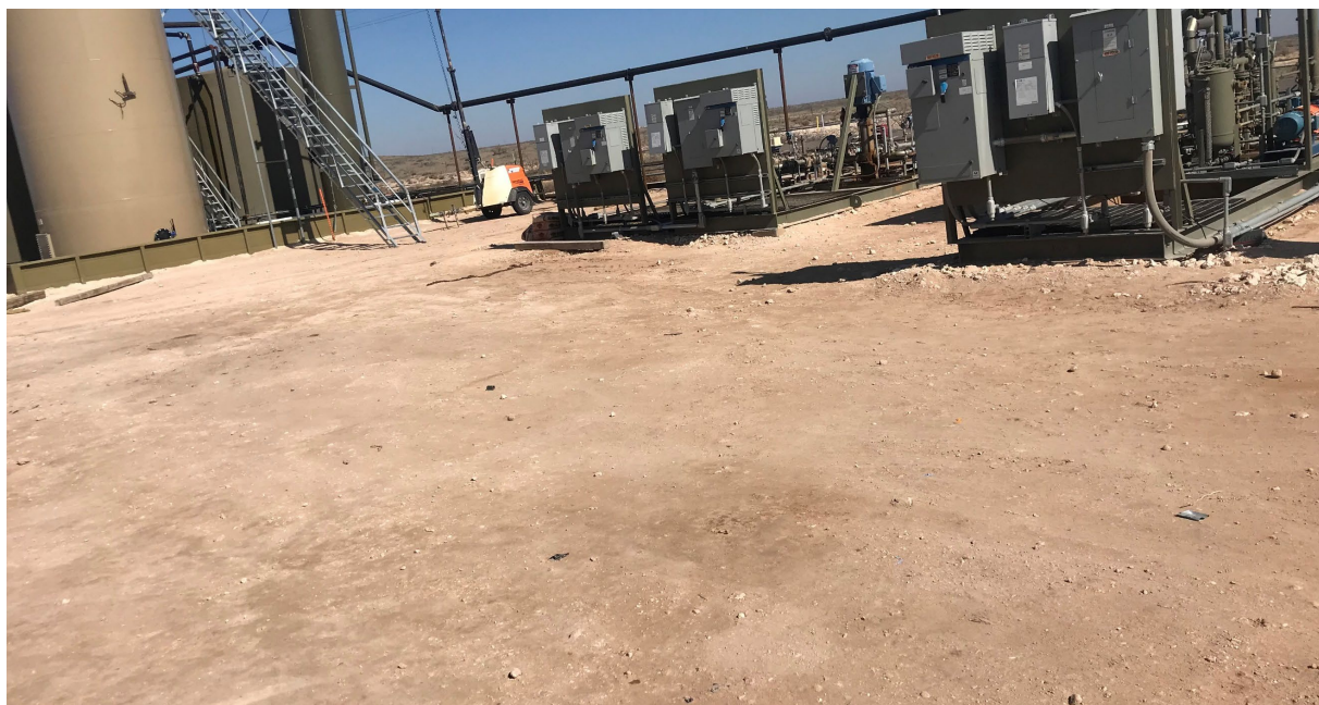
Photo 6 View to the east-northeast at the backfilled remedial excavation.
