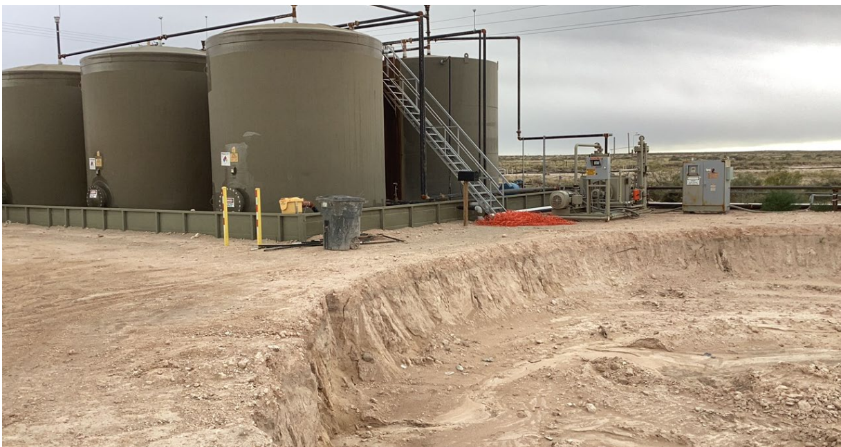
Photo 4 View of the northern portion of the remedial excavation adjacent to the Earthstone tank battery.
