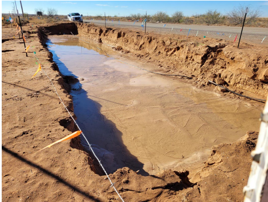
View of southern excavation facing southwest.
