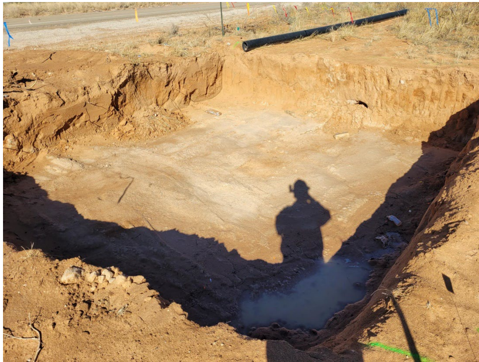
View of northern excavation facing northeast
