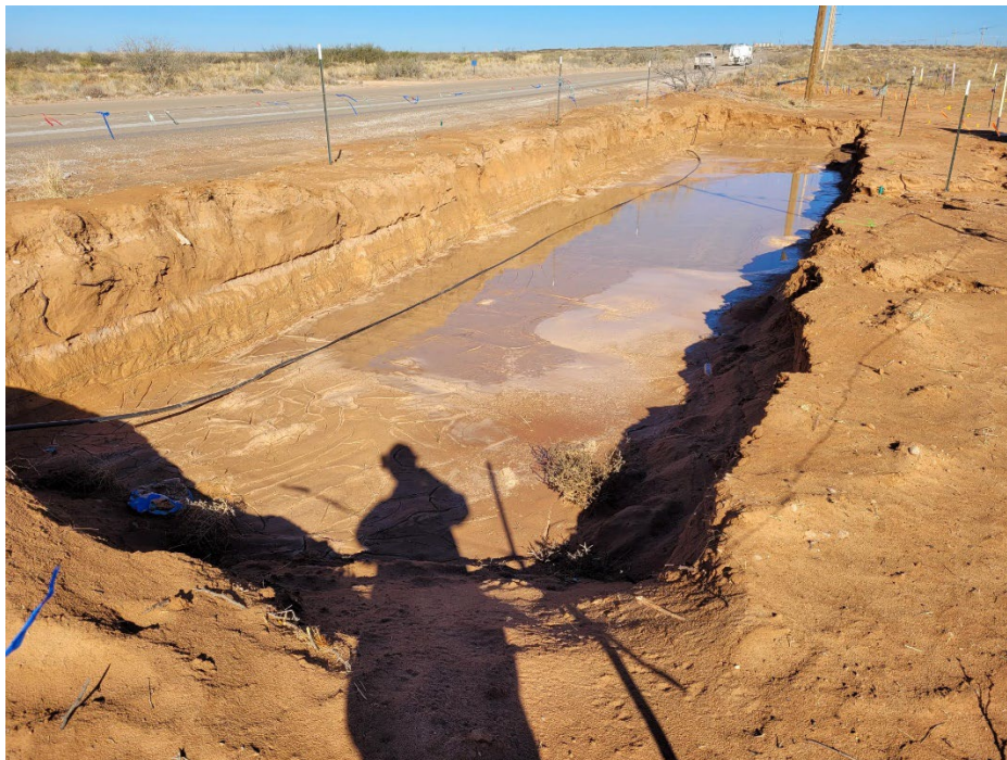
View of southern excavation facing northwest.
