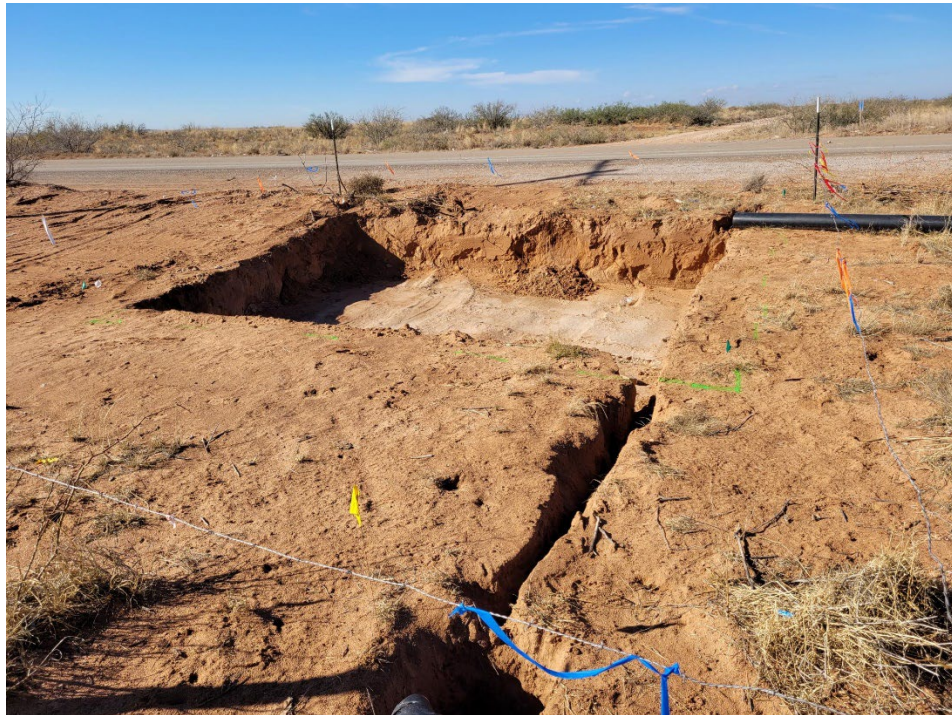
View of northern excavation facing southwest.
