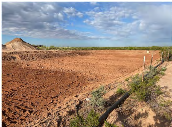
Photograph 1 Date: 4/14/2020 Description: Southwestern excavation area, view southwest
