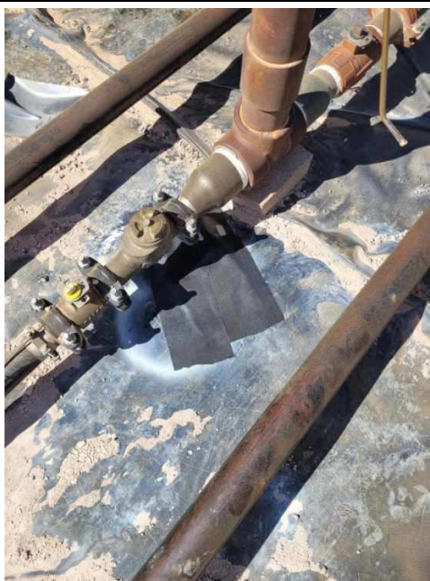
Photograph 1 Date: 4/4/2023 Description: Patched liner and backfilling activities View: Southeast
