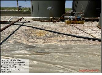
Photograph: 3 Date: 5/30/2023 Description: View of the lined containment deemed to be in good condition. Photograph: 4 Date: 5/30/2023
