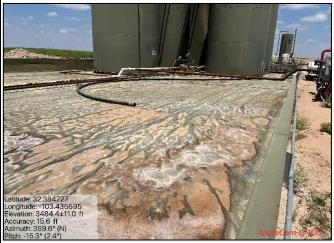
Photograph: 1 Date: 5/30/2023 Description: View of the lined containment deemed to be in good condition.
