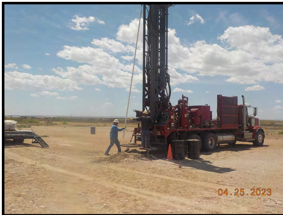
PHOTOGRAPH NO. 9 – A typical view of the April 25, 2023 vertical delineation soil boring and temporary monitor well installation activities.
