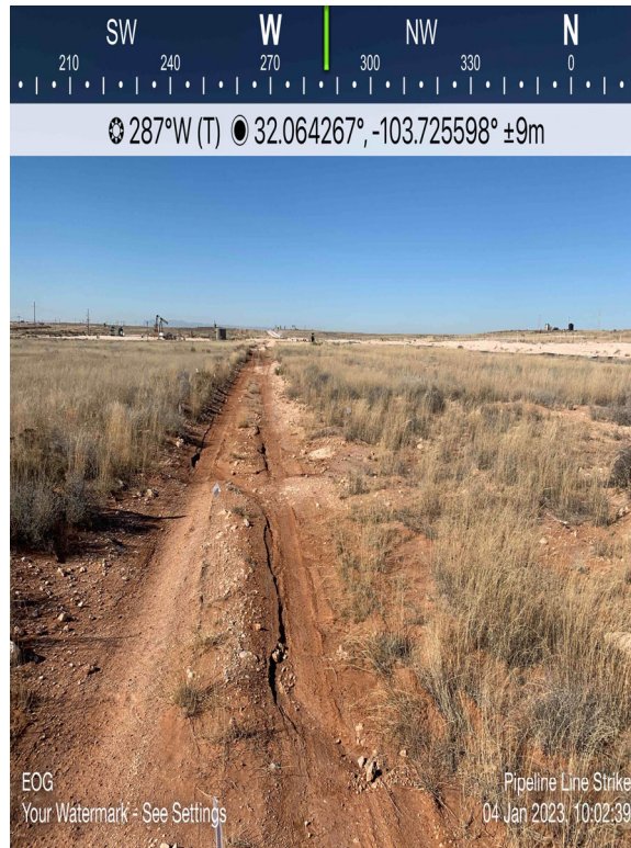
View of Remediation Activities – View West
