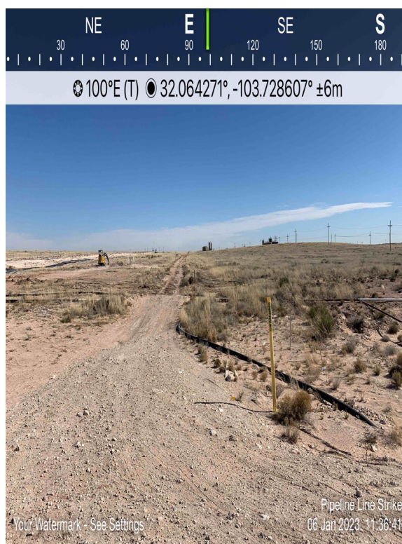
View of Remediation Activities – View East
