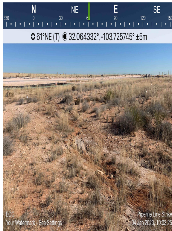
View of Remediation Activities – View Northeast
