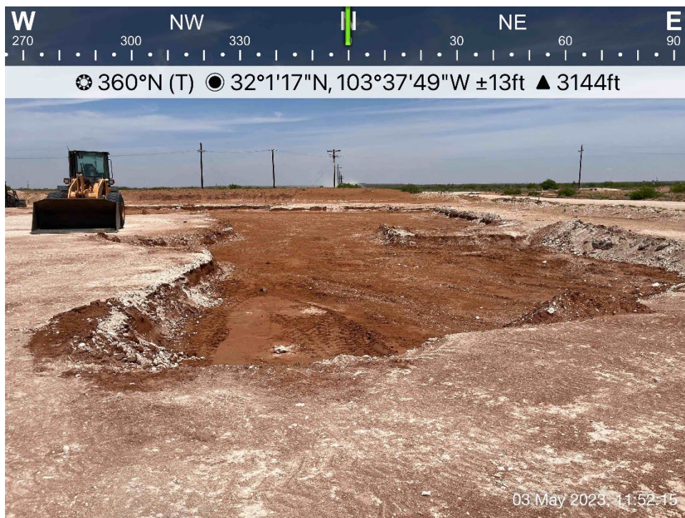
Initially excavated area viewing north, May 3, 2023
