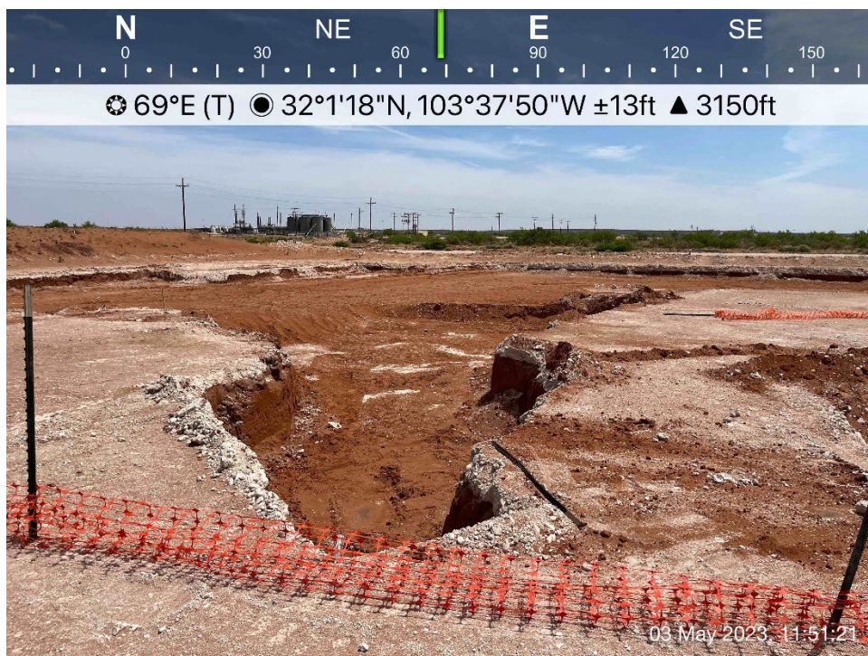
Initially excavated area viewing east, May 3, 2023
