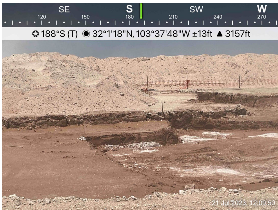
Additional excavated area viewing south, July 21, 2023
