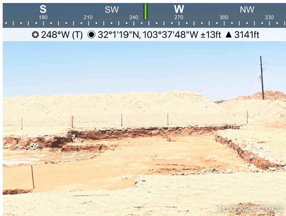
Additional excavated area viewing west, July 21, 2023
