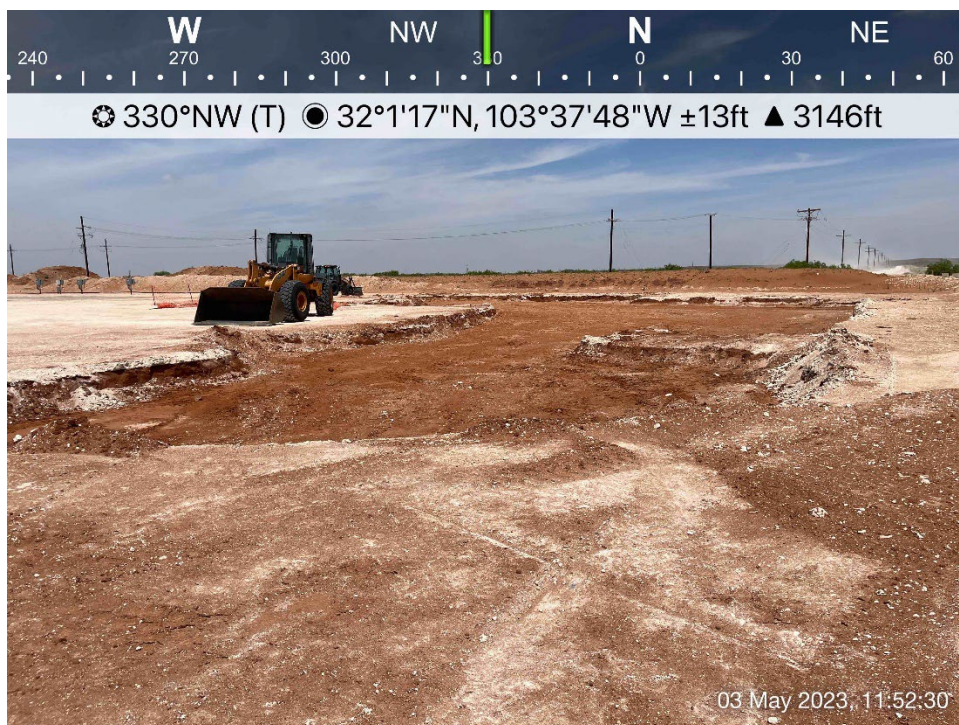
Initially excavated area viewing northwest, May 3, 2023
