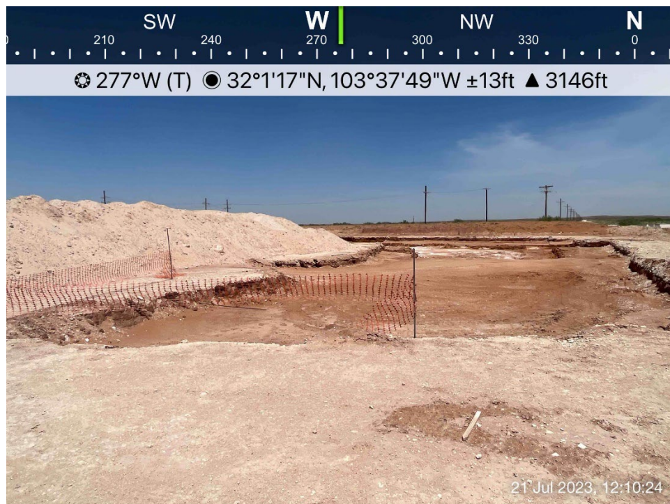
Additional excavated area viewing west, July 21, 2023
