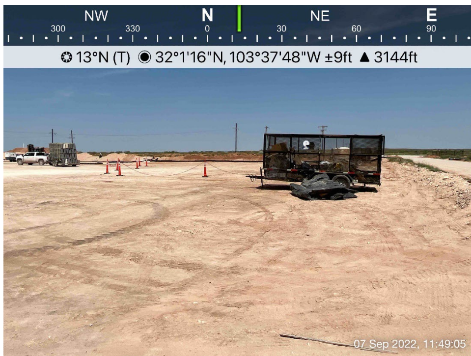
Impacted area viewing north, September 7, 2022
