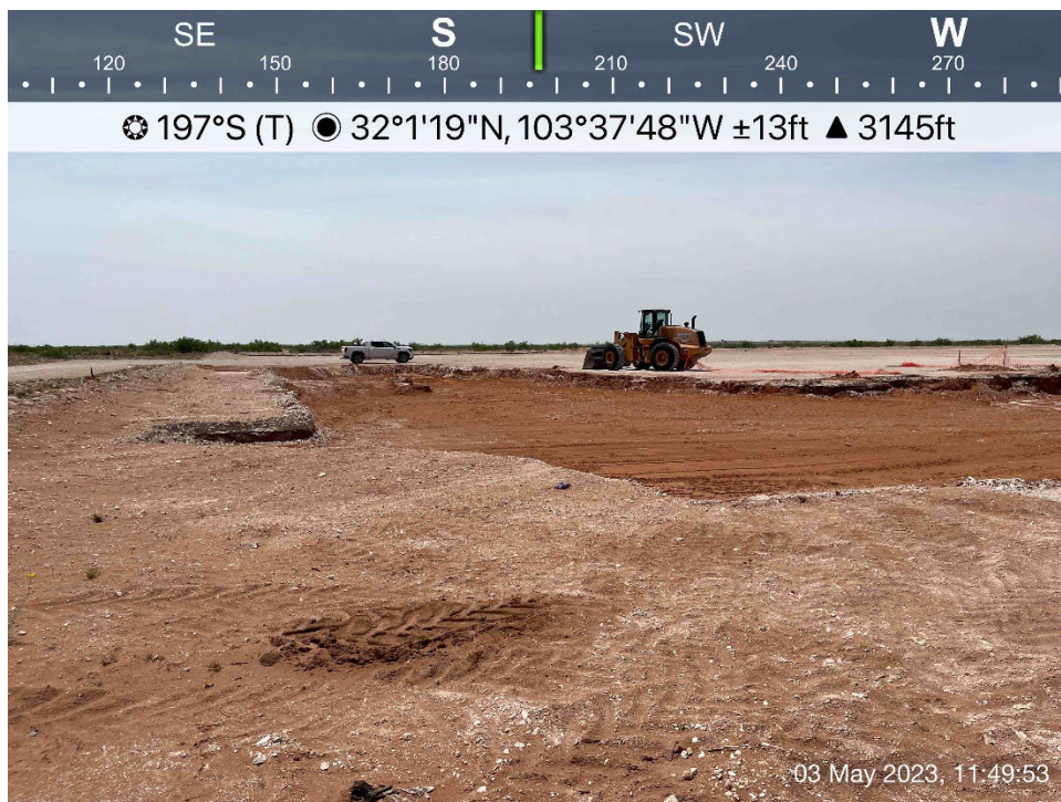
Initially excavated area viewing south, May 3, 2023
