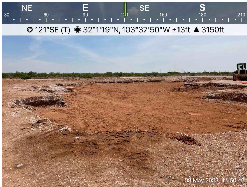
Initially excavated area viewing southeast, May 3, 2023
