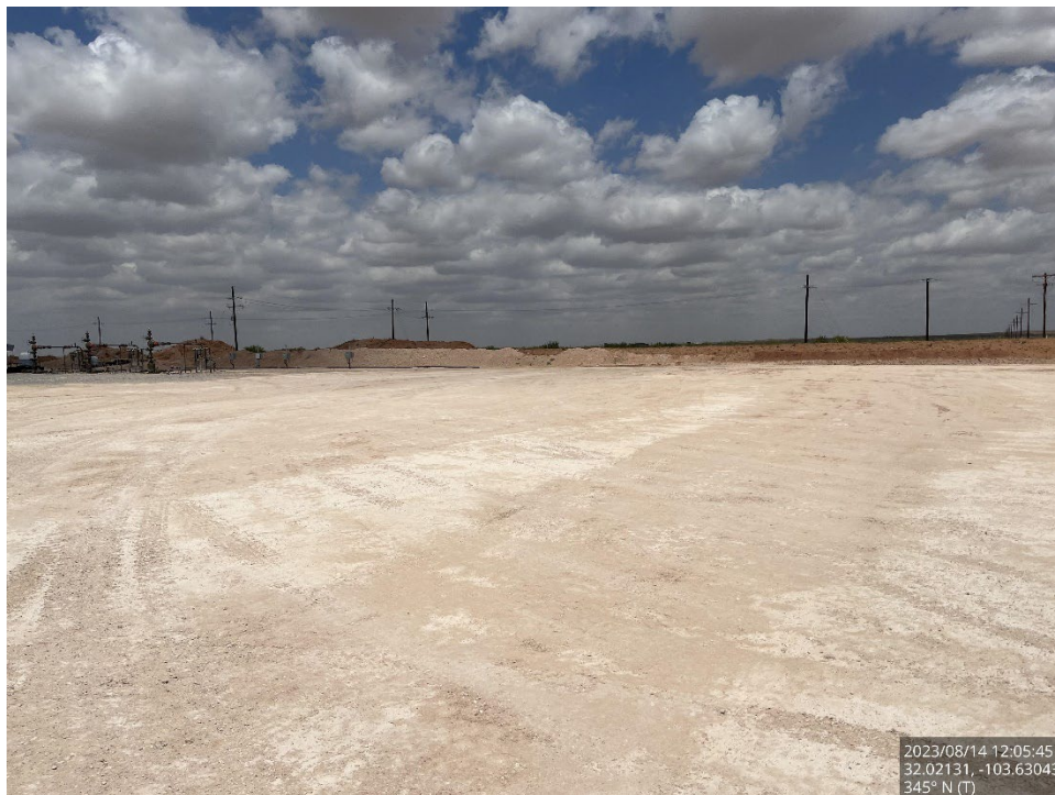
Backfilled area viewing north, August 14, 2023
