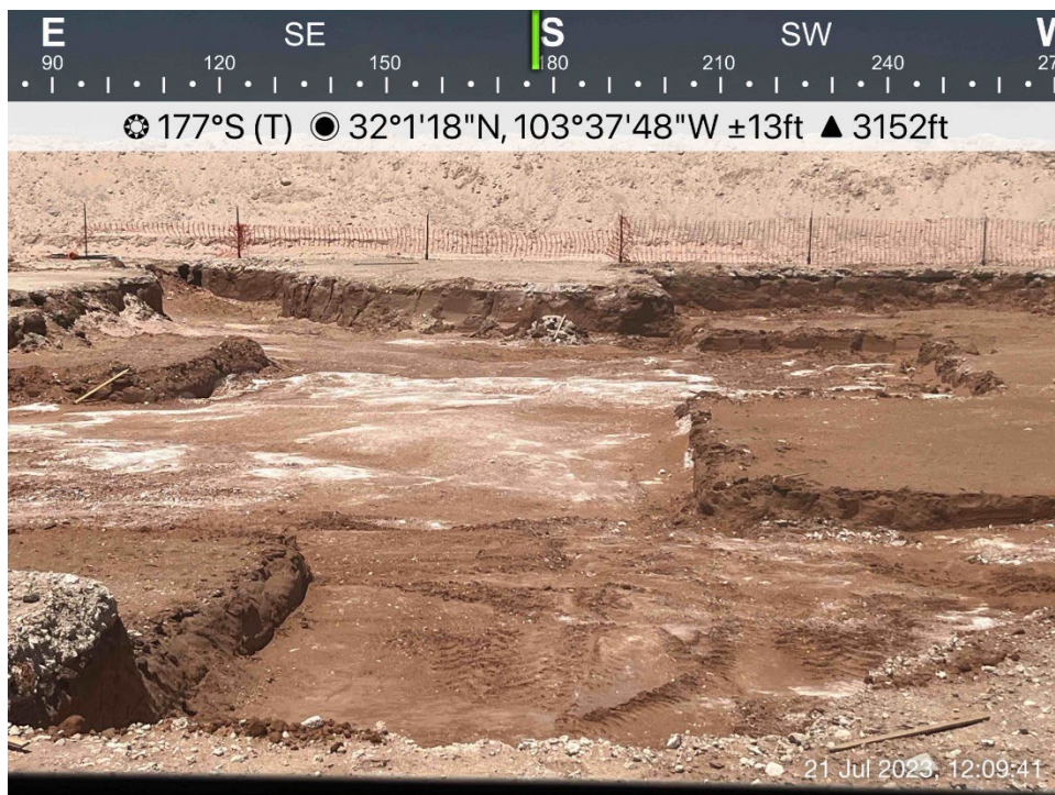
Additional excavated area viewing south, July 21, 2023
