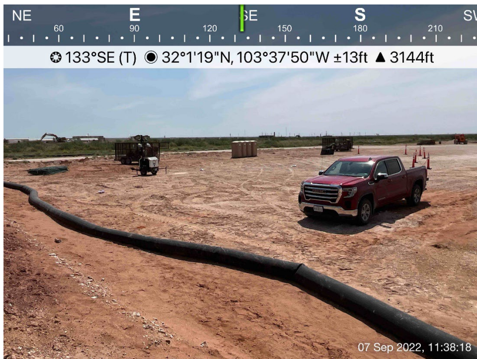
Impacted area viewing southeast, September 7, 2022
