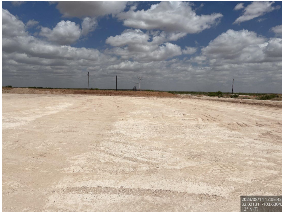
Backfilled area viewing north, August 14, 2023
