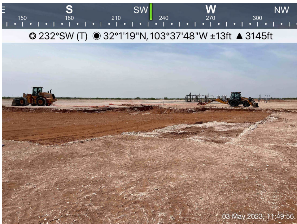
Initially excavated area viewing southwest, May 3, 2023
