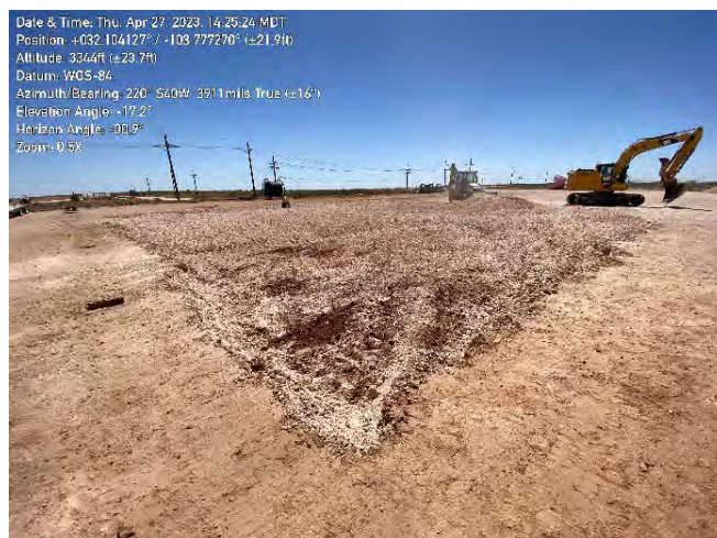
Photograph 3 Date: 04/27/2023 Description: Excavation activities on pad View: Southwest
