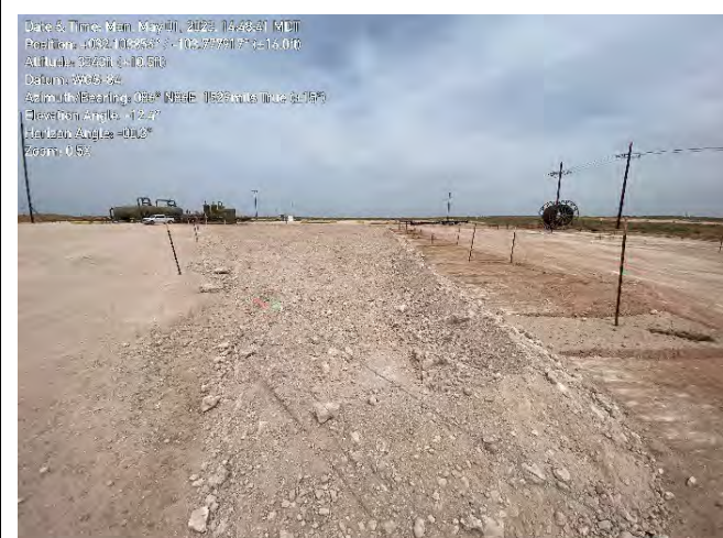
Photograph 4 Date: 05/01/2023 Description: Completed excavation extent View: Northeast
