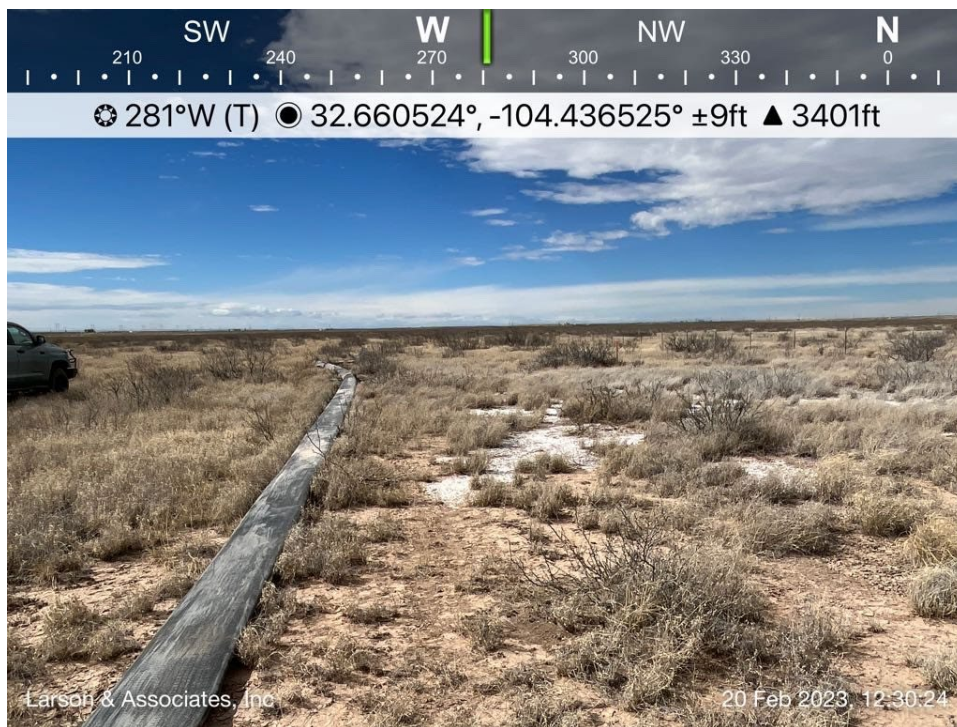
Surface chloride staining in pasture area, viewing to the west.
