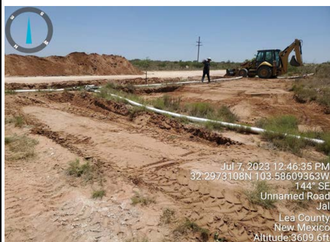
Photograph: 4 Date: 7/7/2022 Description: Excavation activities View: East
