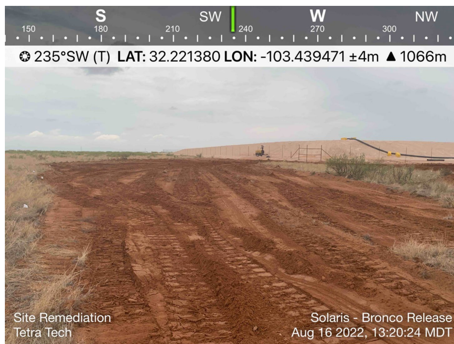
View of Initial Remediation Activities – View Southwest
