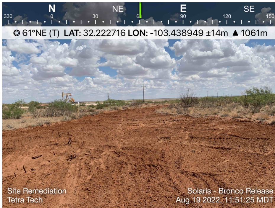
View of Initial Remediation Activities – View Northeast
