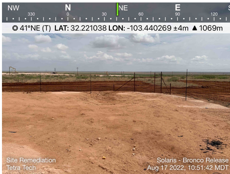
View of Release Area – View Northeast
