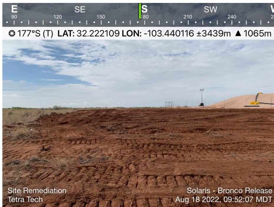
View of Initial Remediation Activities – View South
