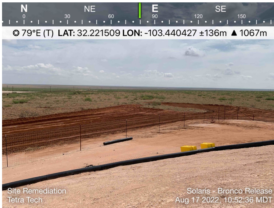
View of Initial Remediation Activities – View East
