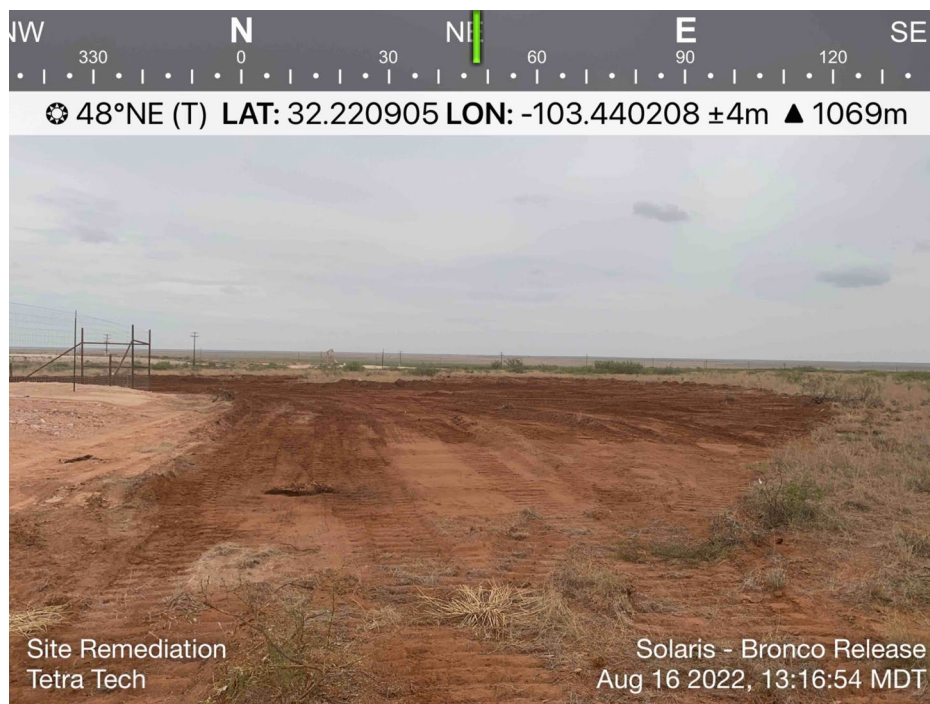
View of Initial Remediation Activities – View Northeast
