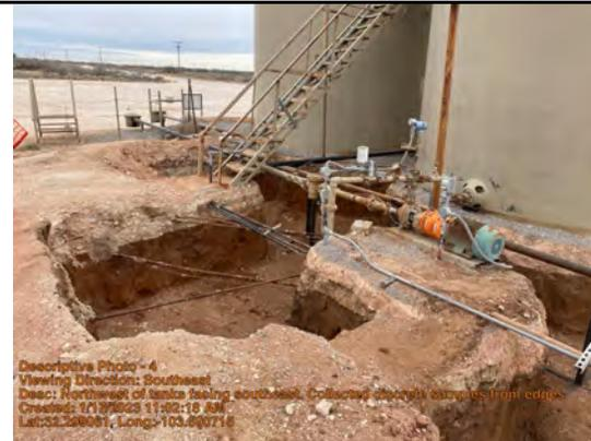
Northwest of tanks facing southeast. Collected discrete samples from edges of excavation.
