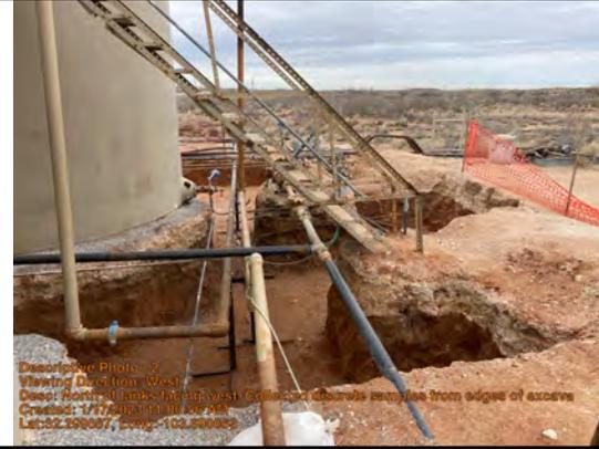
North of tanks facing west. Collected discrete samples from edges of excavation.
