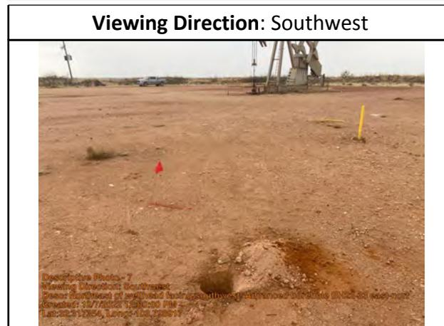
Northeast of wellhead facing southwest. Advanced borehole BH22-33 east-northeast of BH22-32 for horizontal delineation.
