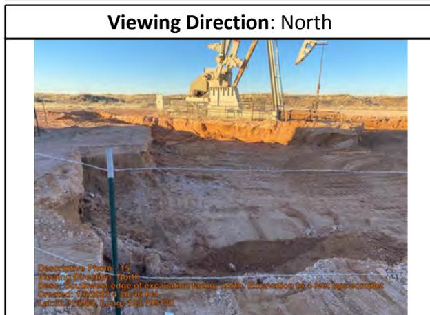
Southwest edge of excavation facing north. Excavation to 4 feet bgs completed.
