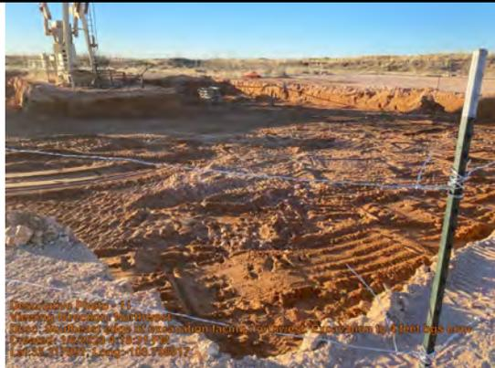
Southeast edge of excavation facing northwest. Excavation to 4 feet bgs completed.
