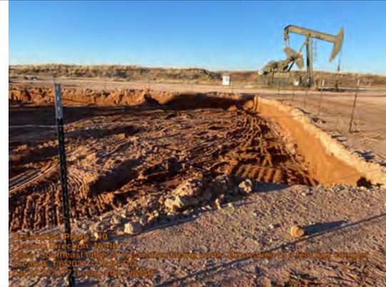
Southeast edge of excavation facing north. Excavation to 4 feet bgs completed.
