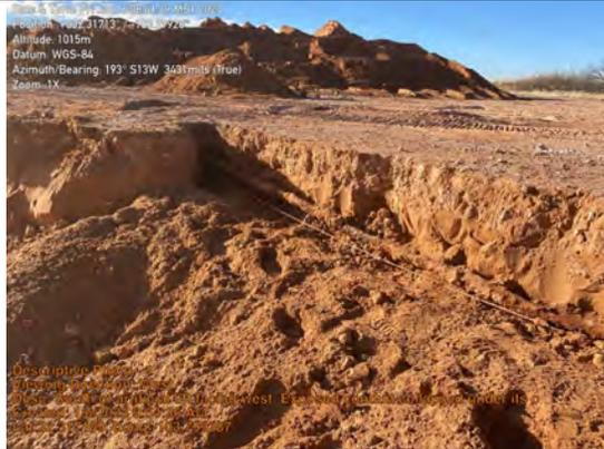
South of artificial lift facing west. Exposed conduit collapsed under its own weight.
