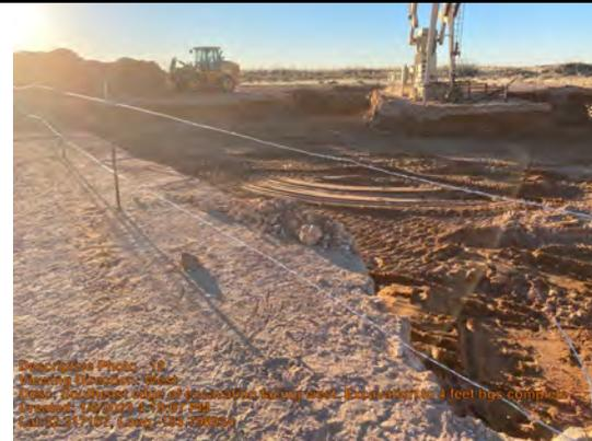
Southeast edge of excavation facing west. Excavation to 4 feet bgs completed.
