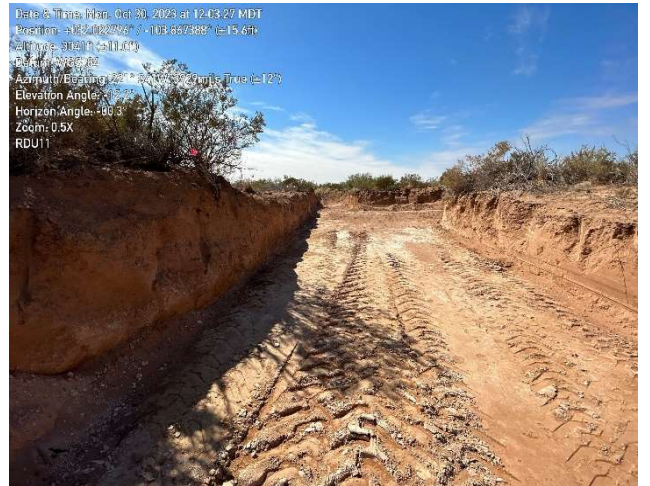
Photograph 4 Date: 10/30/2023 Description: Southwestern view of excavation activities from the northern excavation.
