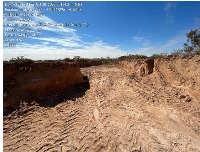
Photograph 3 Date: 10/30/2023 Description: Southwestern view of excavation activities from the northern excavation.
