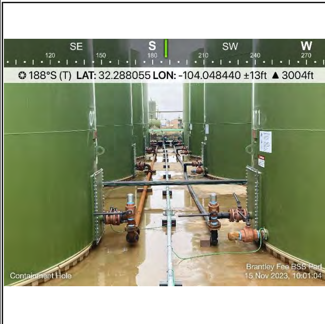
Photograph 1 Description: Containment View: South
