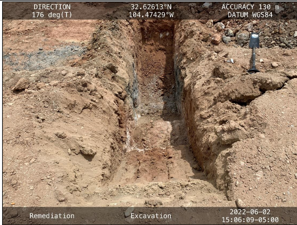
PHOTO 31: View of remediation beginning, facing south.
