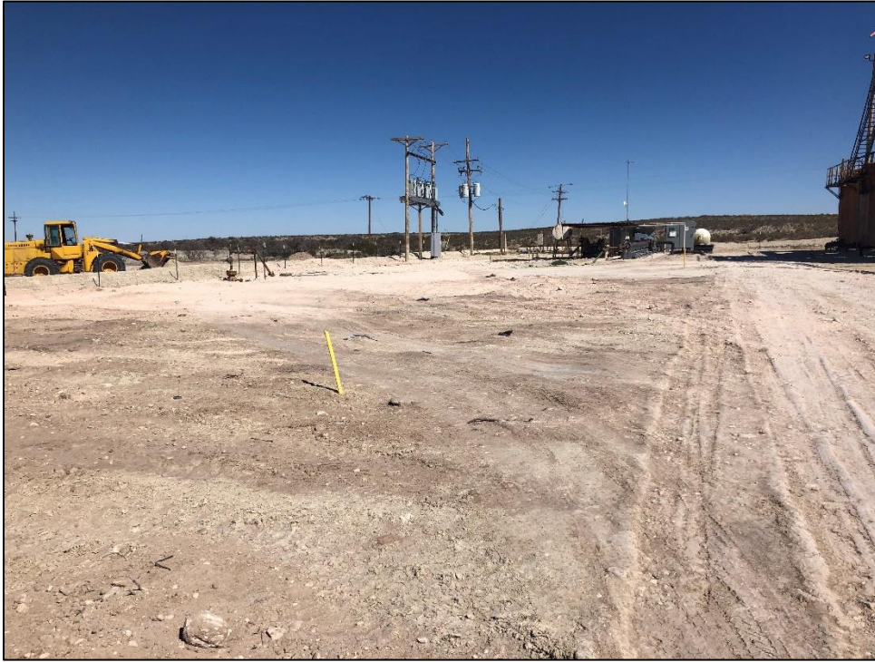
PHOTO 15: View of base of excavation, facing south. 11/22/2019 / TIME: 1:21PM / GPS: 32.1218 -1104.0725
