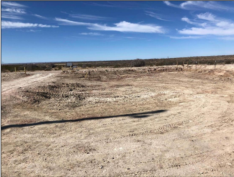
PHOTO 10: View of remediation, facing west. 8/21/2019 / TIME: 1:07PM / GPS: 32.1218 -1104.0725
