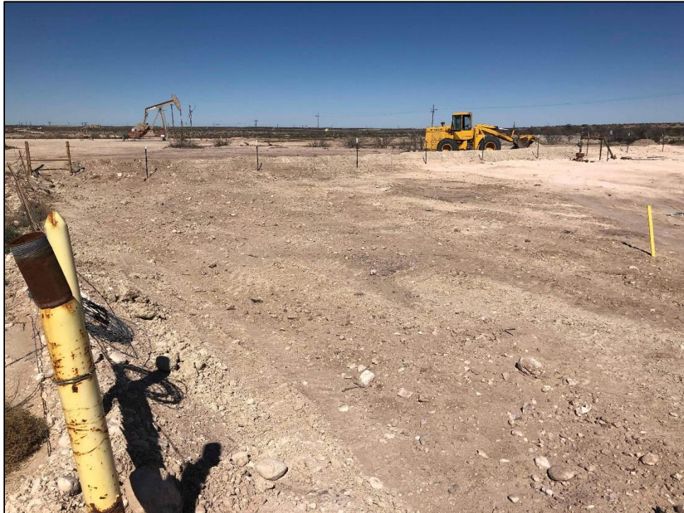
PHOTO 14: View of remediation, facing south. 11/22/2019 / TIME: 1:07PM / GPS: 32.1218 -1104.0725
