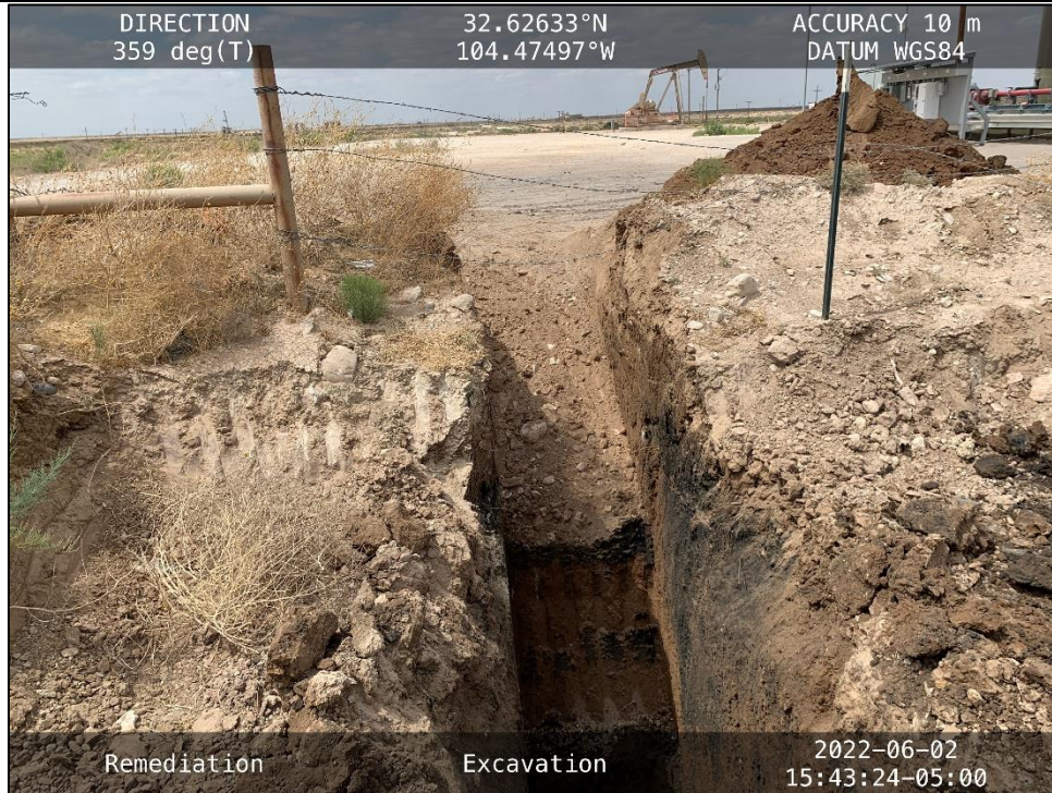
PHOTO 34: View of trenching in northwest corner of excavation, facing north.
