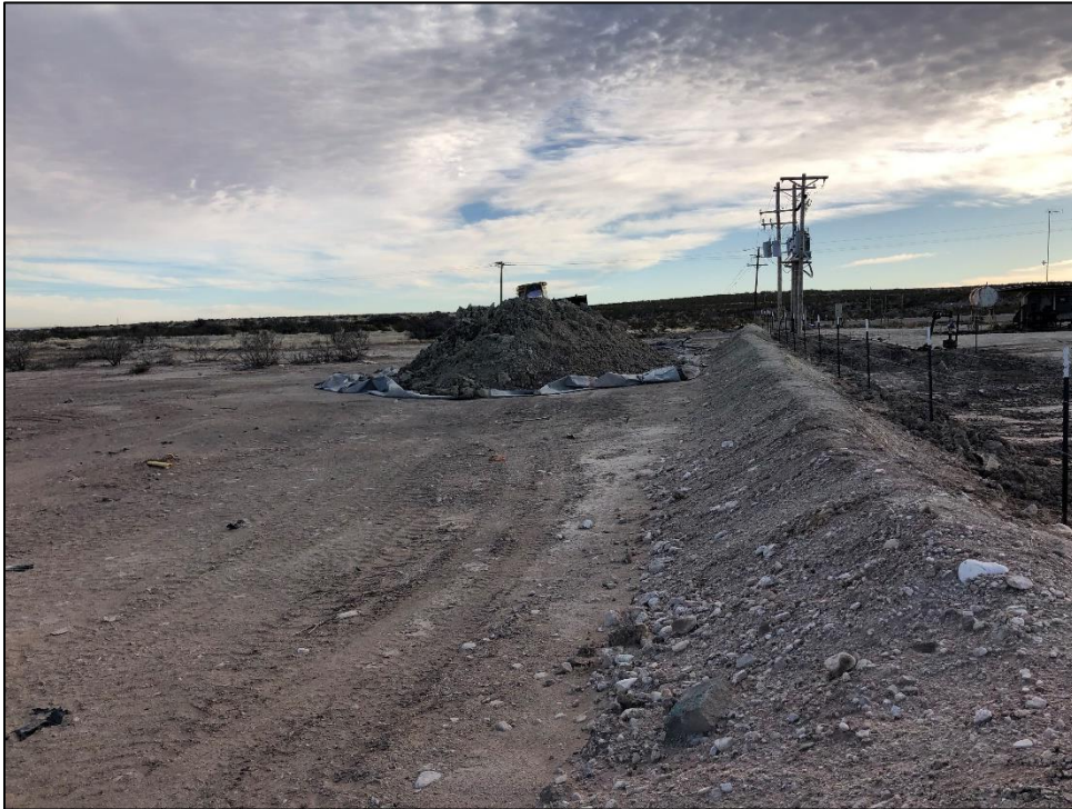
PHOTO 4: View of stockpile north of site, facing east. 1/14/2019 / TIME: 10:16PM / GPS: 32.6261 -104.4748
