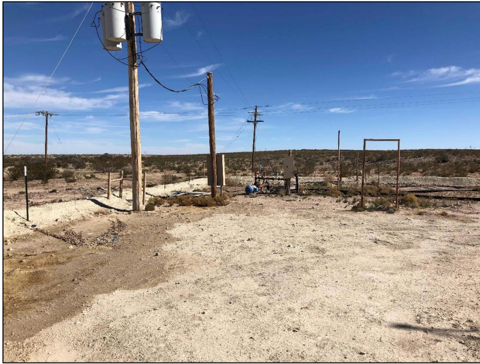
PHOTO 13: View of remediation, facing west. 11/22/2019 / TIME: 1:11PM / GPS: 32.1217 -1104.0726
