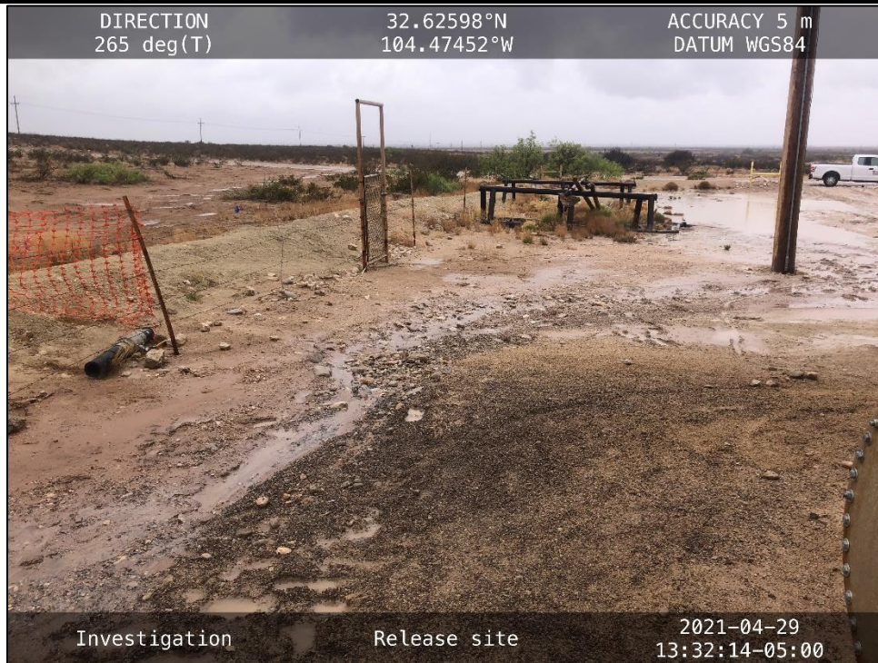
PHOTO 22: View of flow path, facing west.
