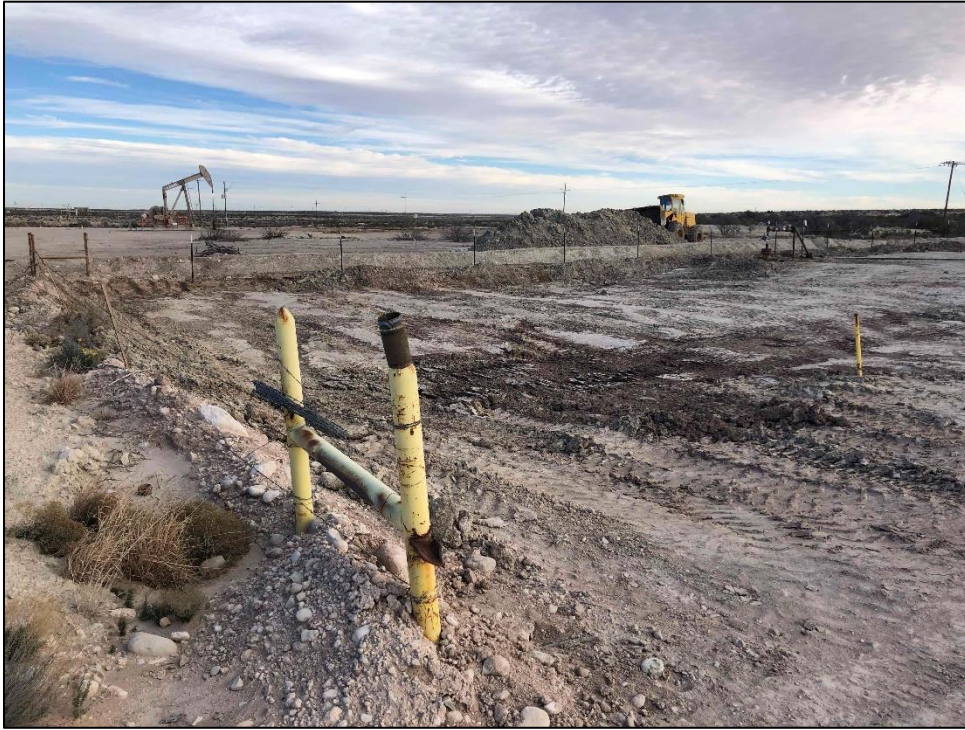
PHOTO 1: View of site, facing north. 1/14/2020 / TIME: 10:11AM / GPS: 32.6261 -104.4748
