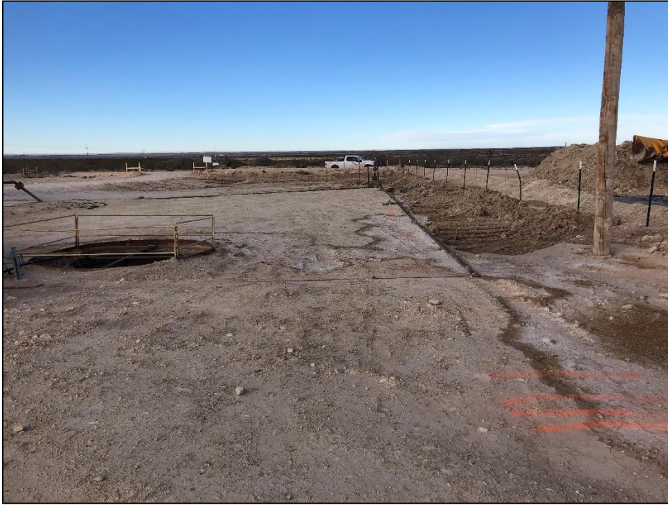
PHOTO 9: View of site, facing west. 7/25/2019 / TIME: 1:11PM / GPS: 32.1217 -1104.0726
