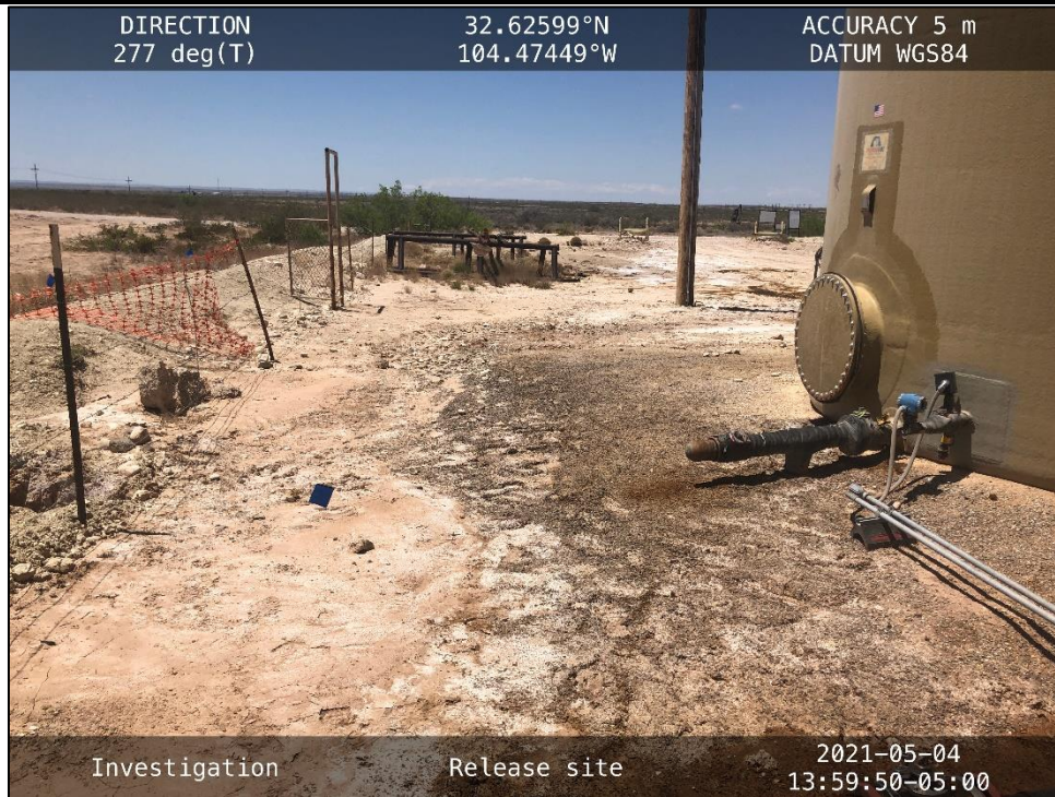
PHOTO 26: View of impacted soils, facing west.
