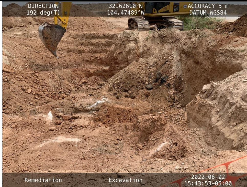
PHOTO 36: View of excavation around (nAPP2127753131), facing south.
