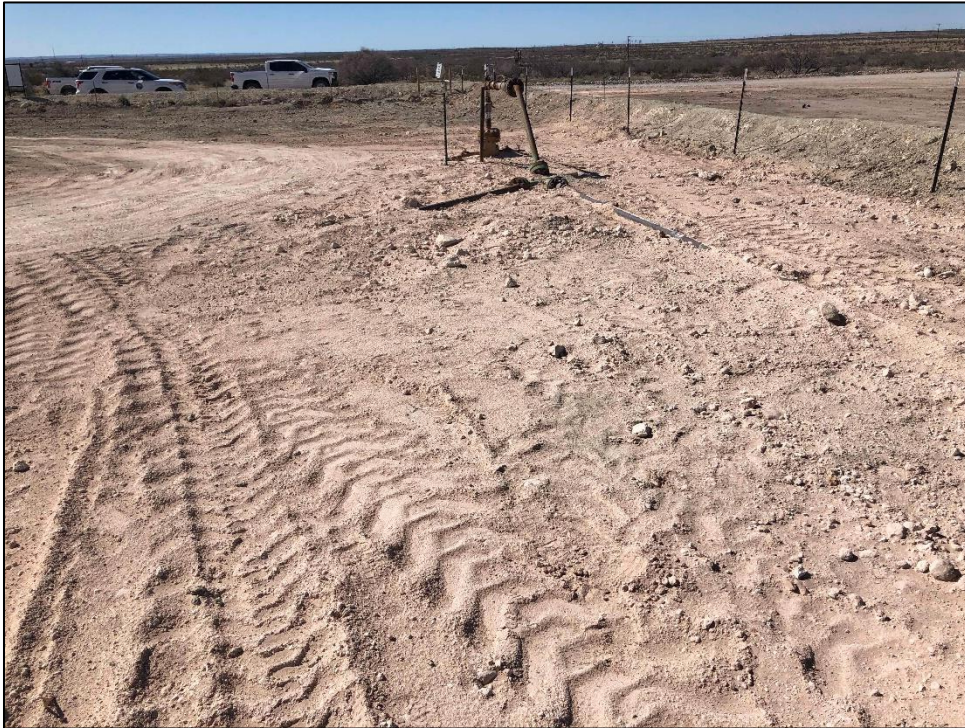
PHOTO 16: View of excavation, facing west. 11/22/2019 / TIME: 1:36PM / GPS: 32.1221 -1104.0725
