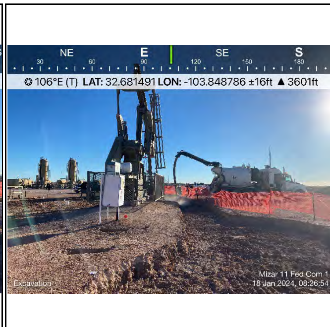
Photograph 18 Description: Hydrovac by well head View: East
