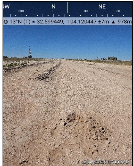
Photograph: 20 Description: Backfill View: North Date: 4/29/2024
