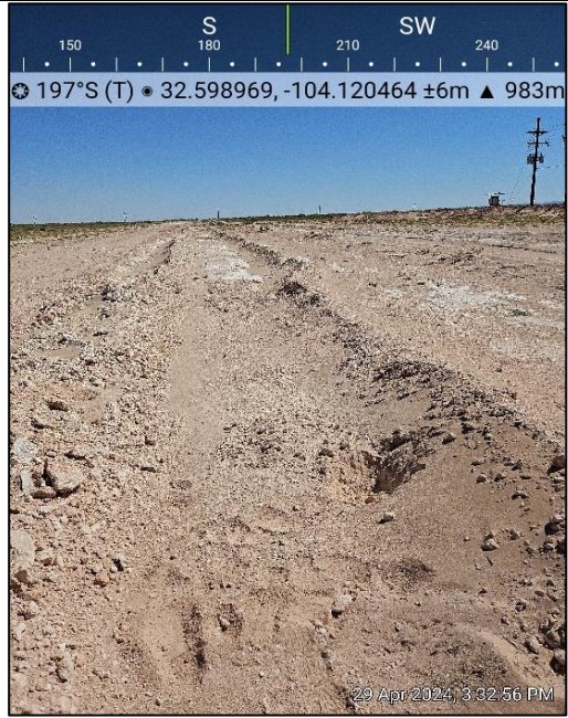
Photograph: 18 Description: Backfill View: South Date: 4/29/2024
