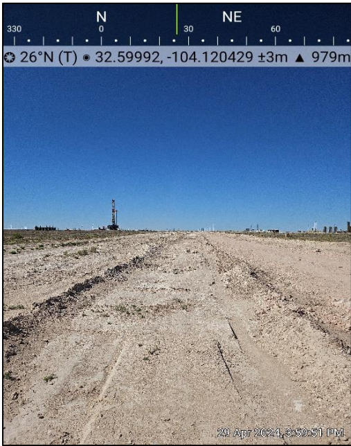
Photograph: 19 Description: Backfill View: North Date: 4/29/2024
