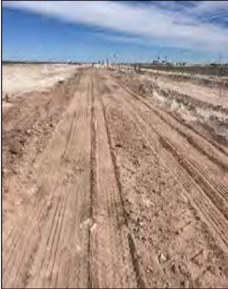
Photograph: 17 Date: 3/25/2024 Description: Backfill View: South
