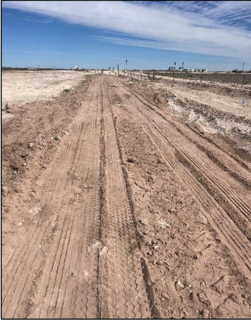
Photograph: 17 Description: Backfill View: South Date: 3/25/2024
