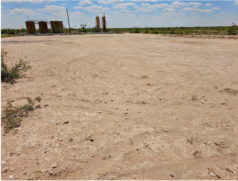
Figure 2: View of pad facing south from the northern edge of the pad. Date Taken: 2023-08-30 13:31:09; GPS: 32.389425, -103.190187
