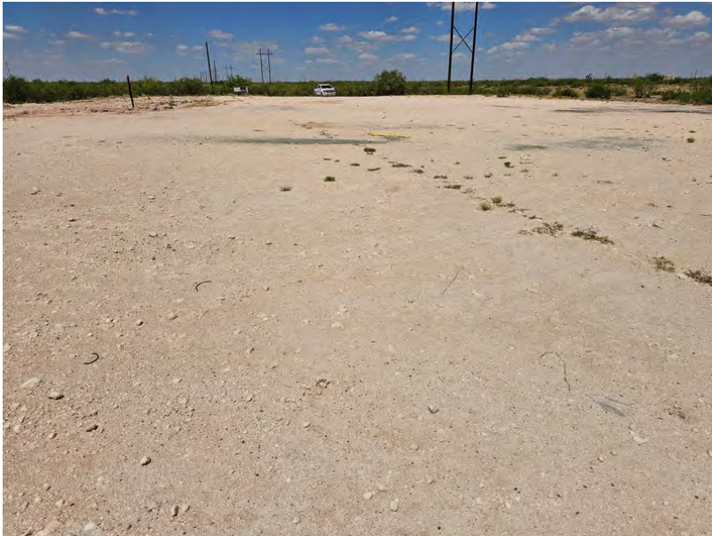
Figure 3: View of well pad facing north from the southern well pad extent. The grey staining in the background is concrete washout/gravel. Date Taken: 2023-08-30 13:32:53; GPS: 32.389005, -103.190061
