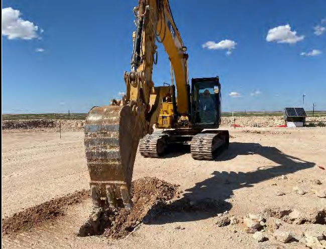
Photograph 1 Date: September 20, 2021 Description: Photo of PH10 taken facing Northwest.
