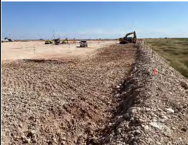
Photograph 3 Date: September 16, 2021 Description: Photo of excavation extent.
