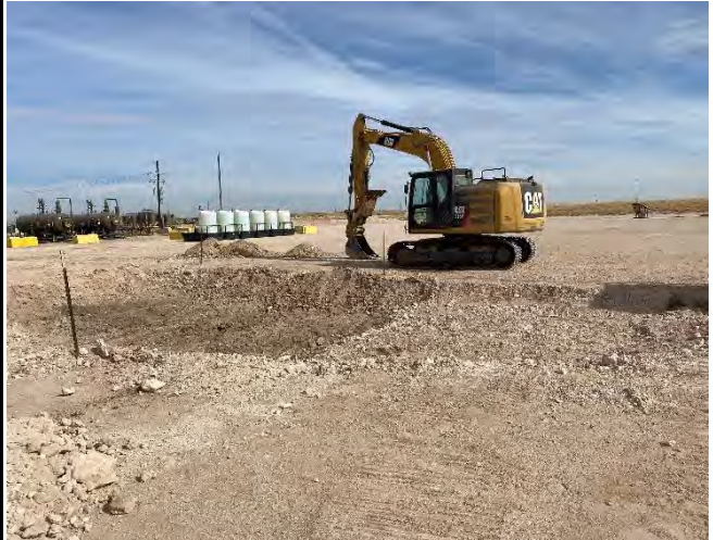
Photograph 2 Date: November 23, 2021 Description: Photo of excavation taken facing East.
