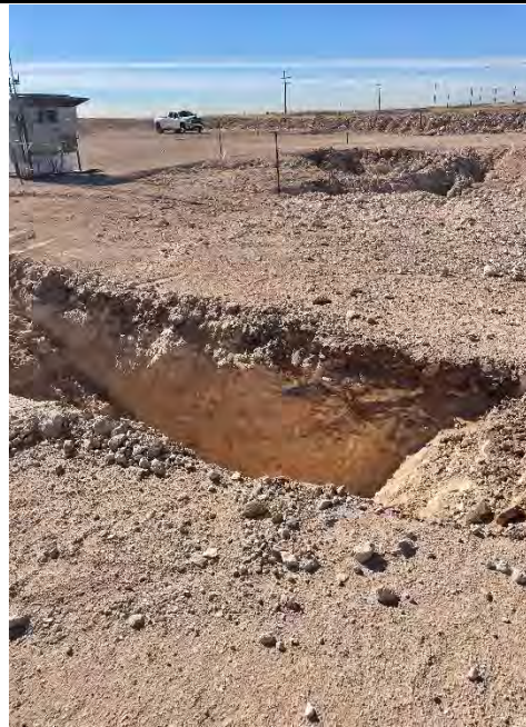
Photograph 4 Date: January 14, 2022 Description: PH20 taken facing West.
