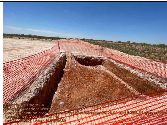
Viewing Direction: West
