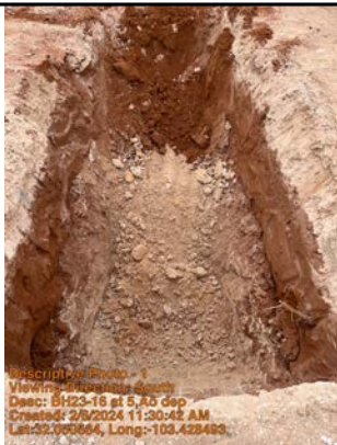
Viewing Direction: South
