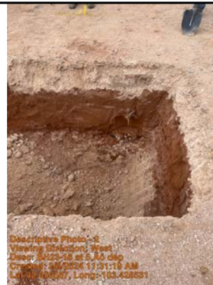
Viewing Direction: West
