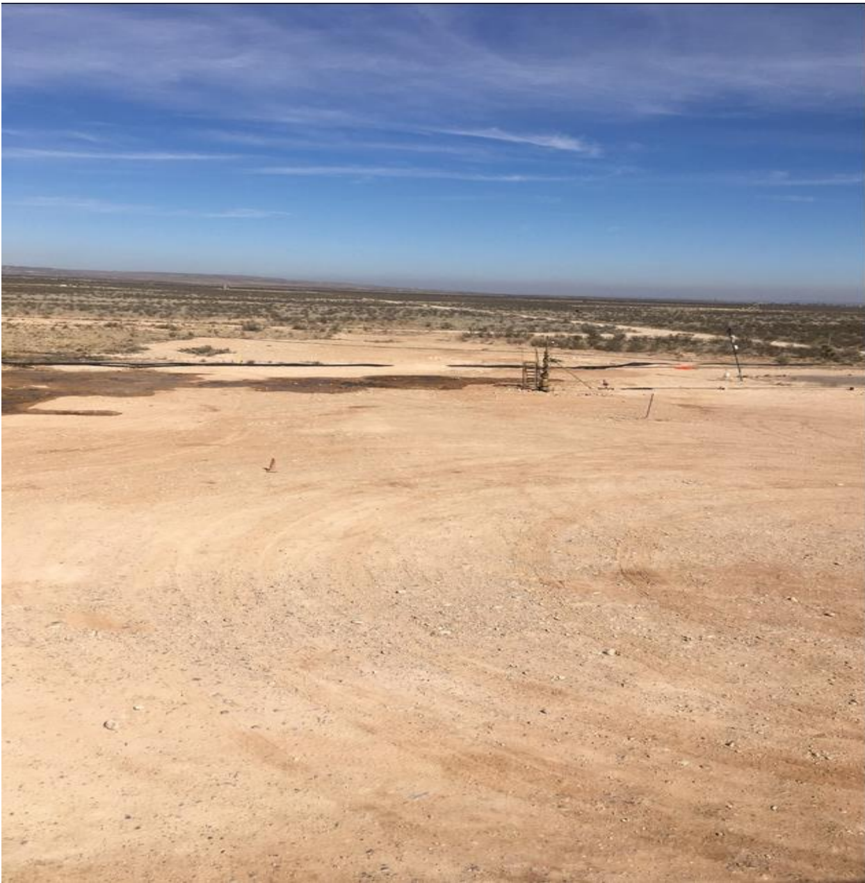
Bandit State #4 Tank Battery looking north.
