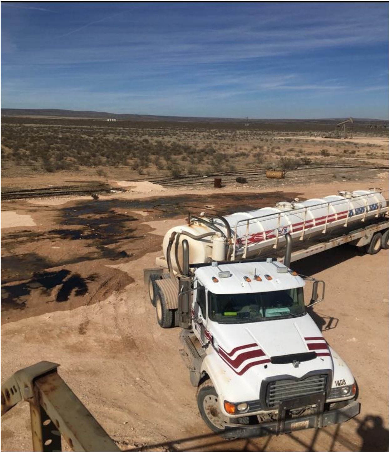
Bandit State #4 Tank Battery looking west.
